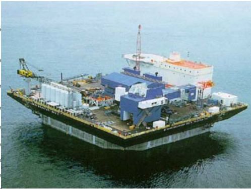
OFFSHORE GAS PLATFORM WITH CONCRETE GRAVITY BASE
