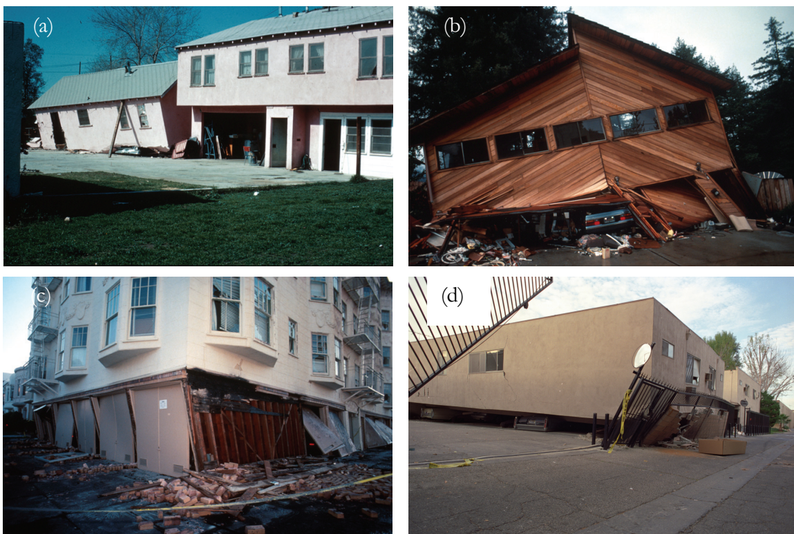
Figure 1.4 (a,b,d) Collapse of Two-Story Buildings due to Inadequate Lateral Strength at the Ground Level, and (c) Excessive Lateral Residual Displacements at the First Story of a Mid-Rise Building. All Cases are Related to a Soft-Story Mechanism (Photo Credit: (a,b,c) USGS, (d) Wikipedia)
