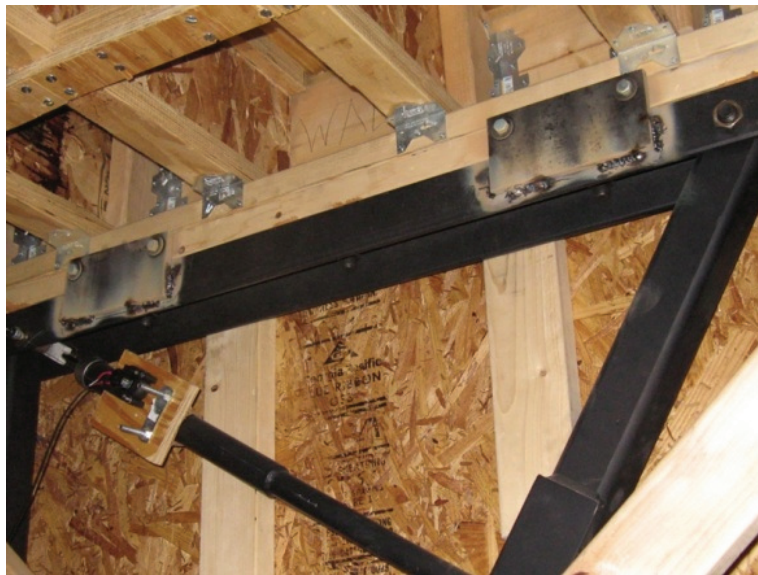
Figure 3.18 Close-Up View of Steel Shear Plates for Reducing Displacement Transmission Losses
