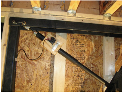
Fluid Viscous Damper Installed with String Potentiometer
