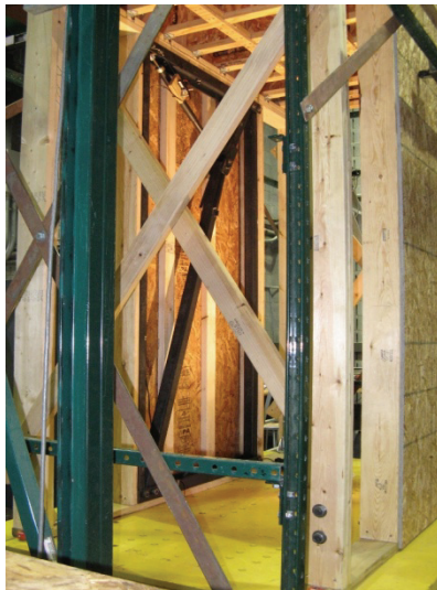
Toggle Assembly Installed inside Retrofitted Wall
