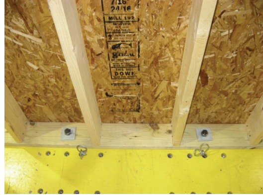
Anchor Bolts with 3 in. Square Washer
