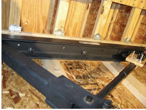
Top Channel Connected to Top Plate with Three A325 Structural Bolts
