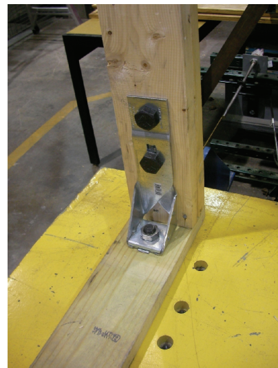
Simpson HD6A Hold-Down Installed in Test Walls
