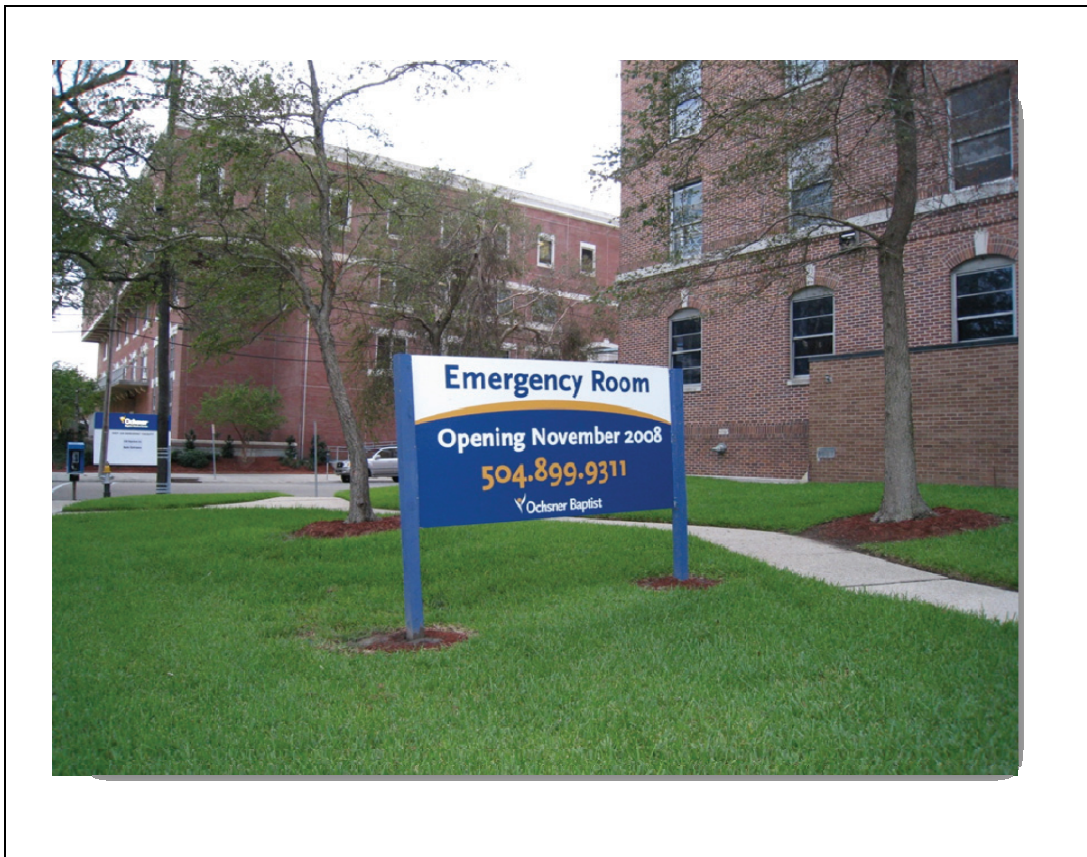
Figure 2-3. Ochsner Baptist, formerly Memorial Medical Center, in Uptown New Orleans. Post-Hurricane Gustav, September 2008.
