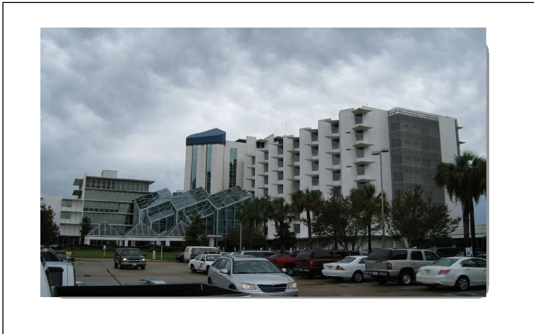
Figure 4-5. West Jefferson Medical Center in Marrero (West Bank of Jefferson Parish). Post-Hurricane Gustav, September 2008.
