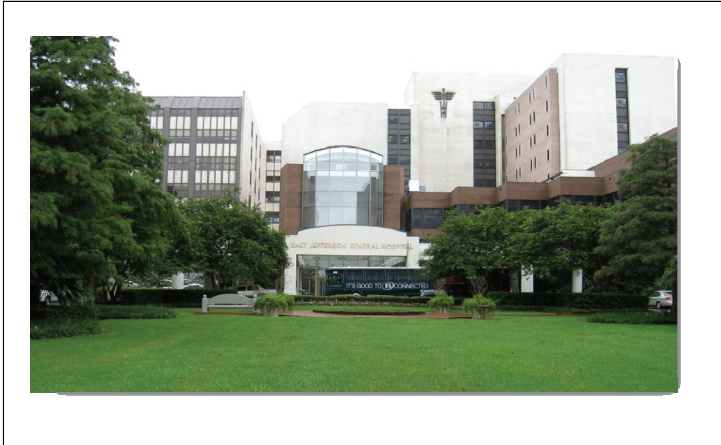
Figure 4-4. East Jefferson General Hospital in Jefferson Parish. Post-Hurricane Gustav, September 2008.
