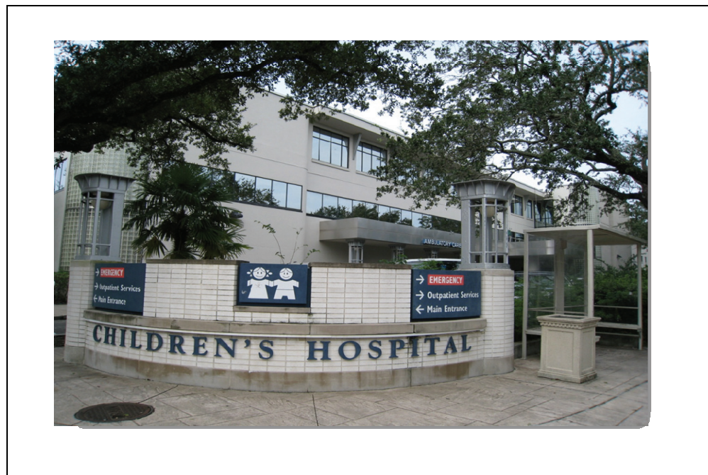
Figure 4-7. Children's Hospital in the Garden District of New Orleans. Post-Hurricane Gustav, September 2008.
