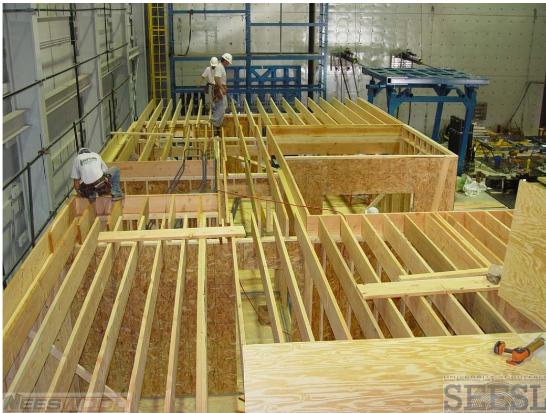
Figure 3.5: Installation of floor joists during construction
