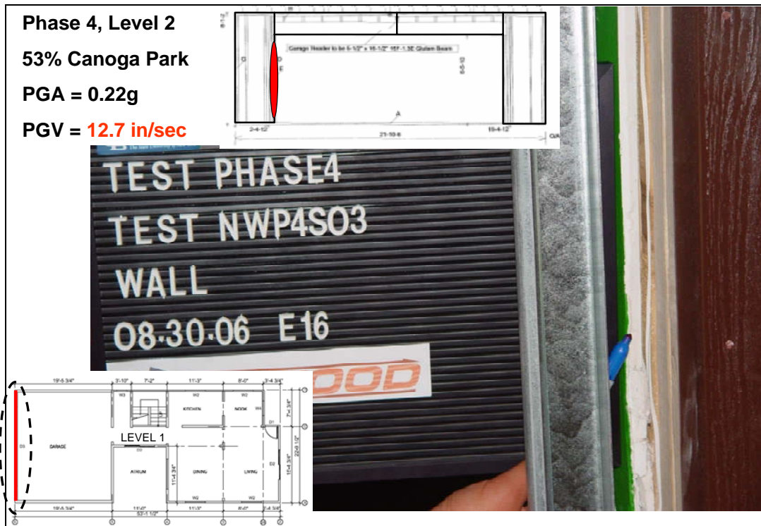
Screw pull-out in gypsum wallboard
