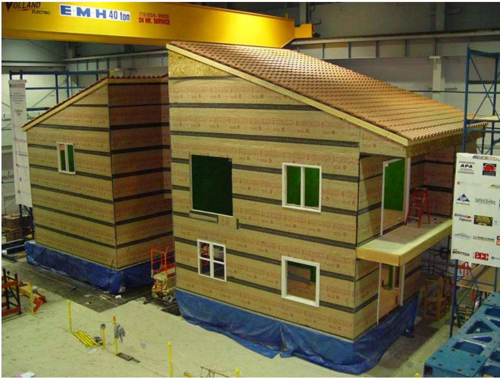
Figure 3.17: Installation of vapor permeable, water-resistant tar paper on the test structure
