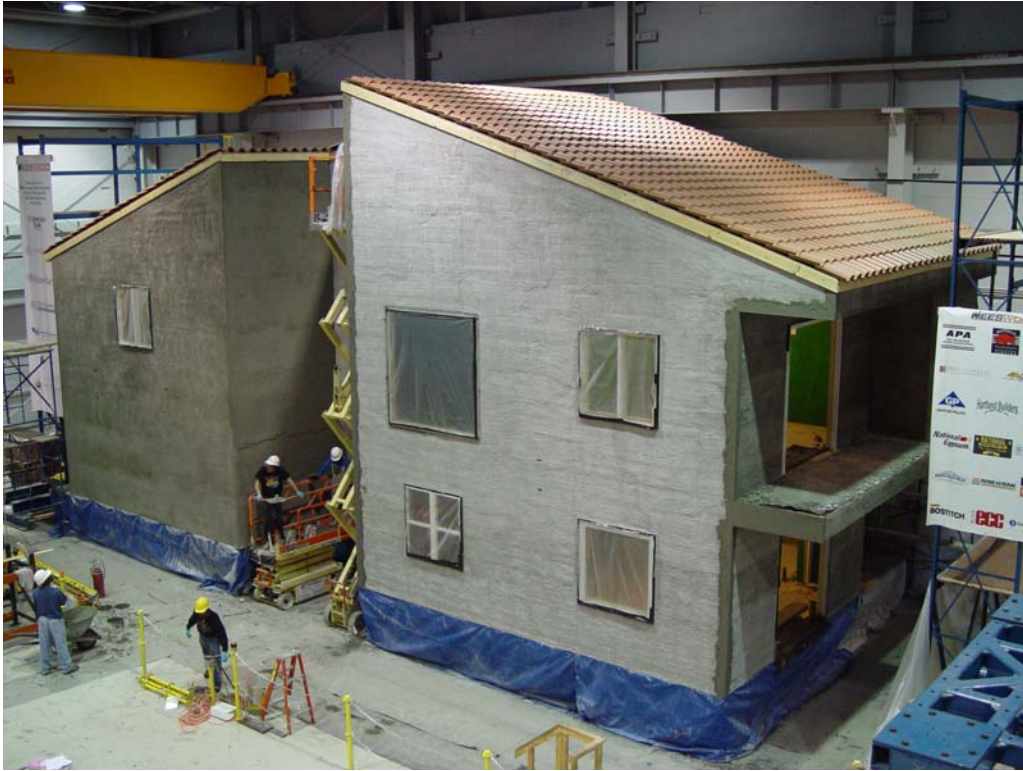
Figure 3.19: Application of the second coat of plaster on the test structure
