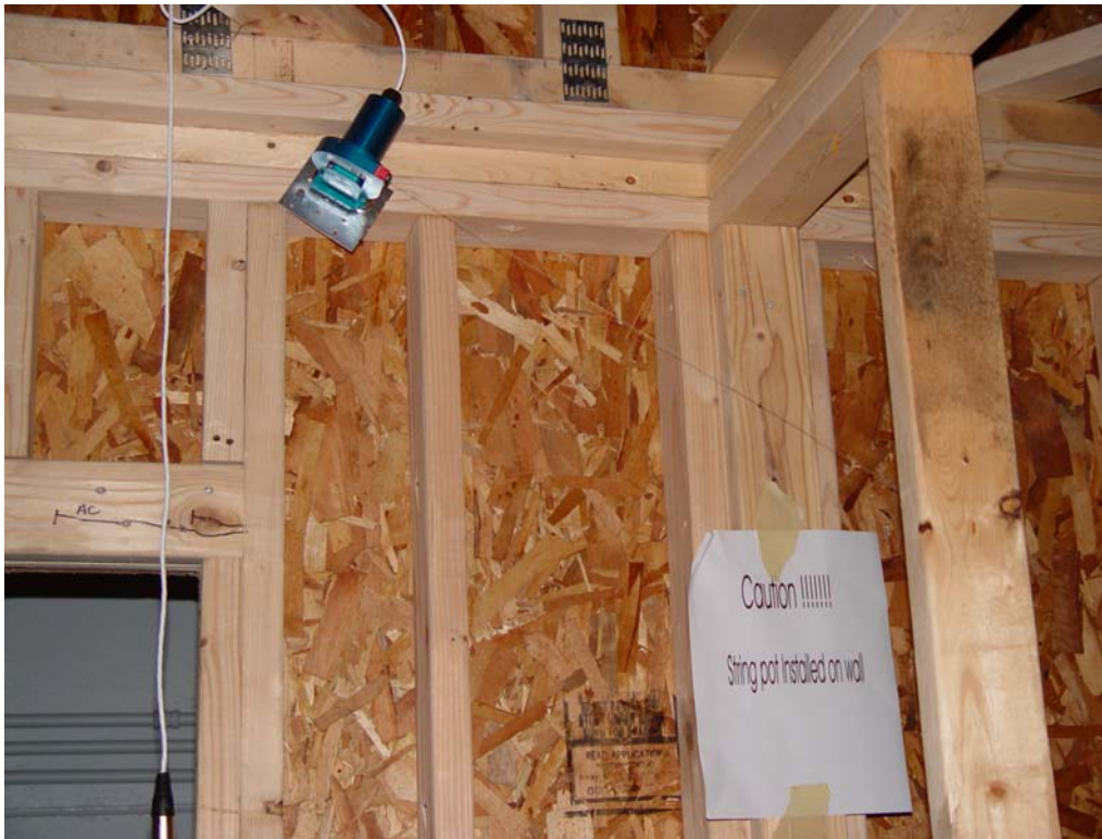
Figure 4.3: String potentiometer located on the top plate of a second floor shear wall
