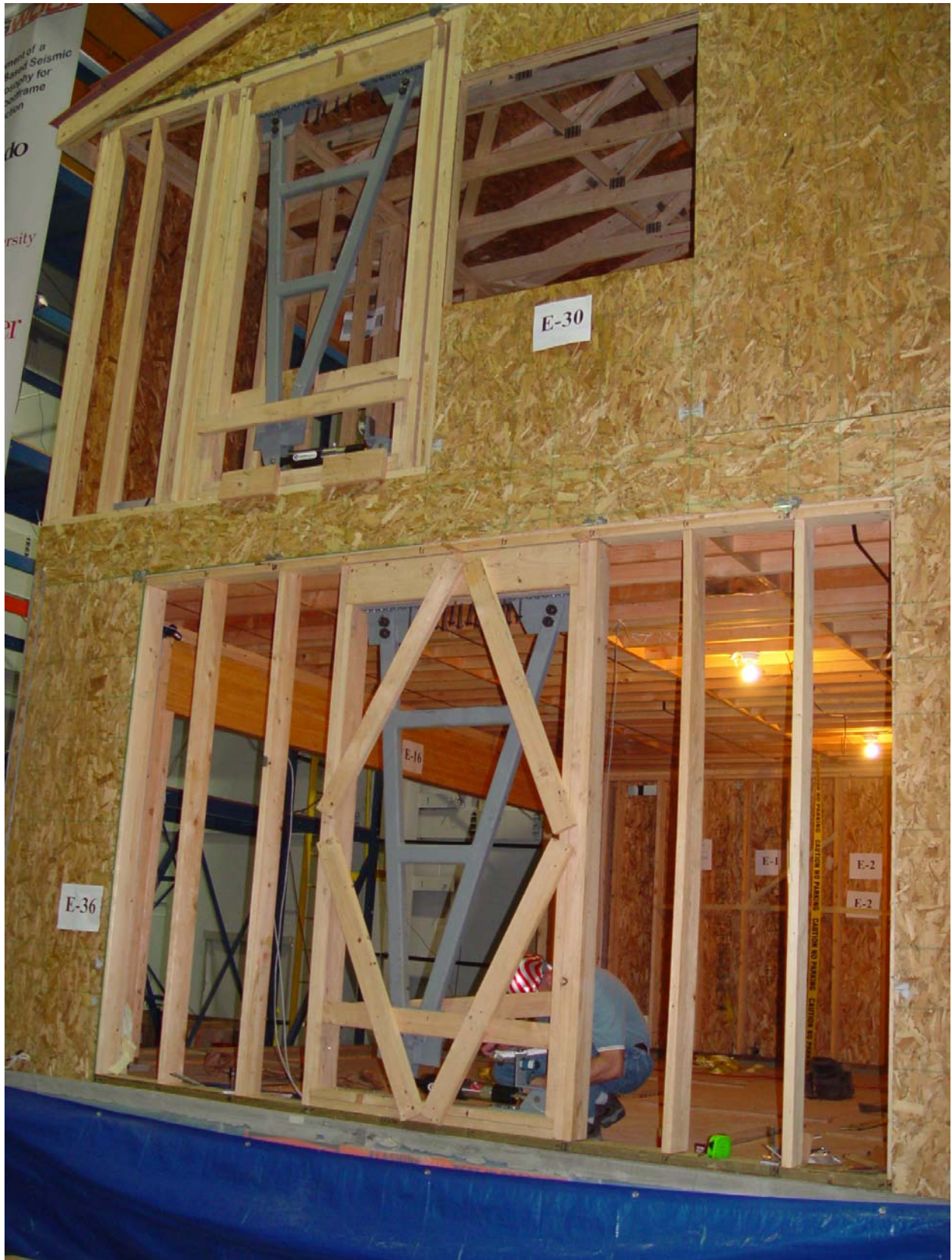
Figure 3.12: Installation of the damper-wall units on the south-west side of the structure
