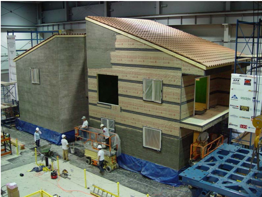
Figure 3.18: Application of the first coat of plaster on the test structure
