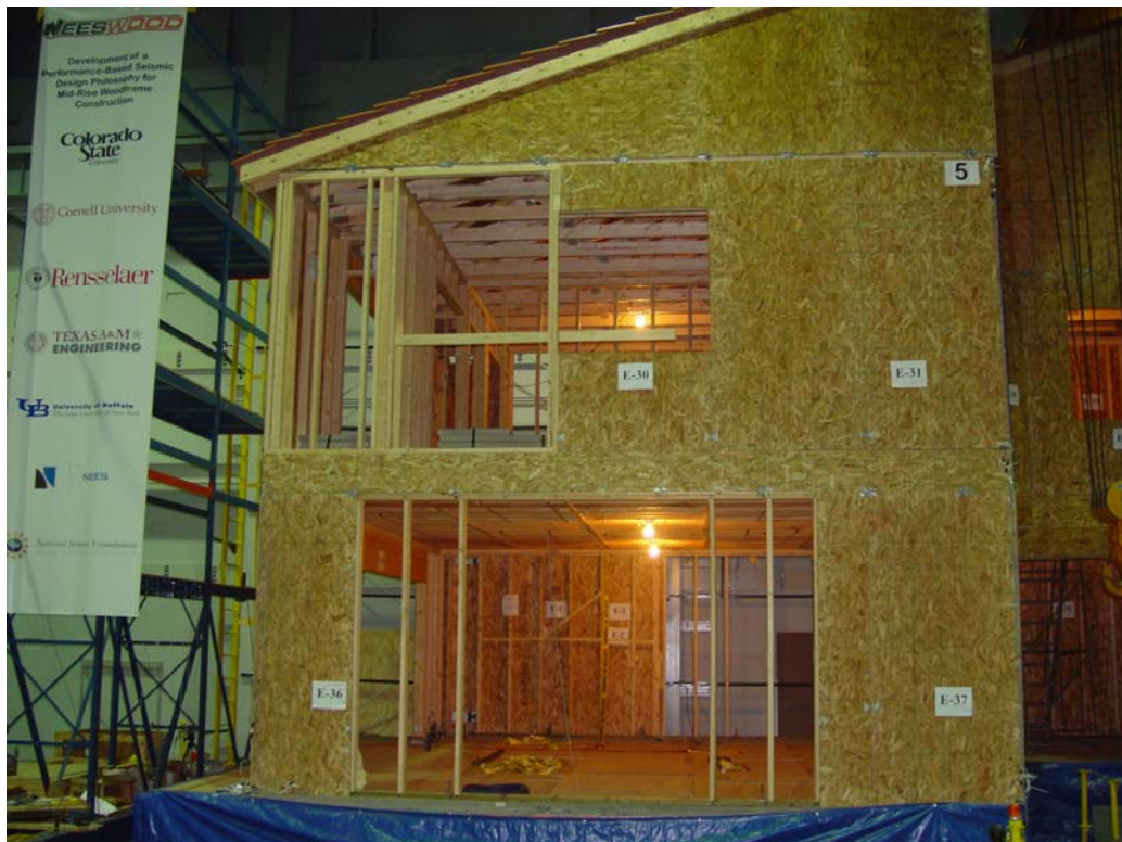
Figure 3.11: The benchmark structure before the installation of the damper-wall units
