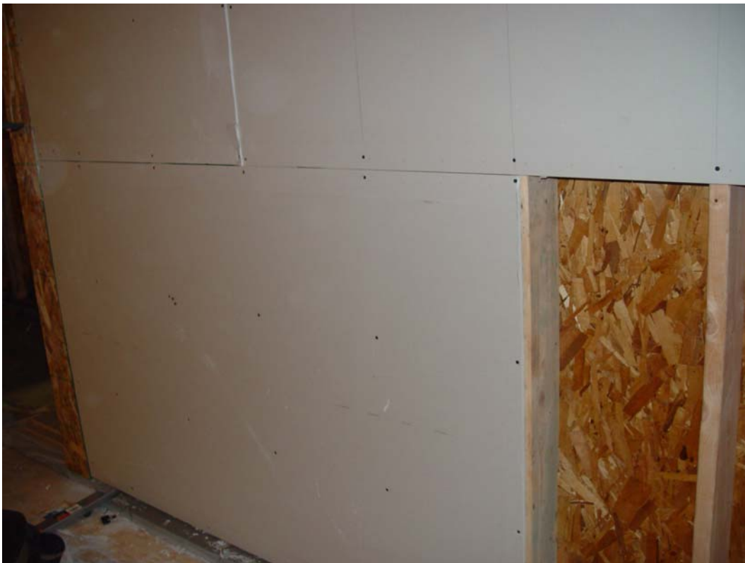
Figure 3.13: Installation of gypsum wallboard on interior surface of a shear wall
