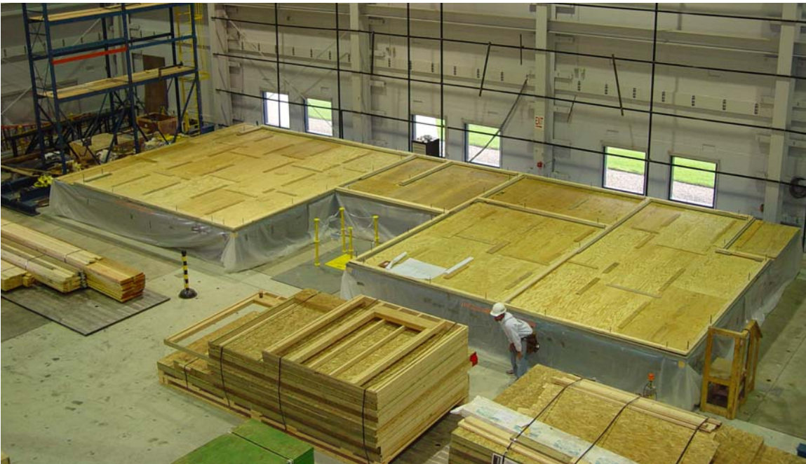
Figure 2.4: (a) Extension frame of shake tables connected by steel link structure, and (b) Foundation of Test Building under Construction
