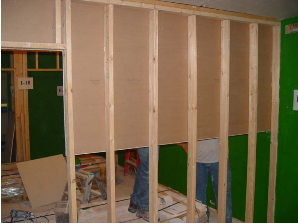
Figure 3.15: Installation of gypsum wallboard on an interior partition wall
