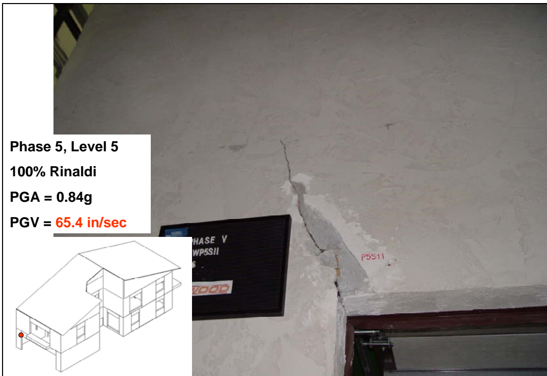
Cracking and spalling of stucco at corner of garage wall opening
