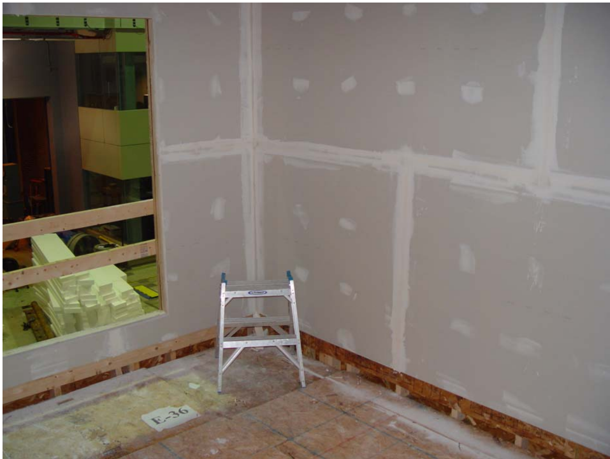
Figure 3.14: View of the interior wall finishes after mudding and taping
