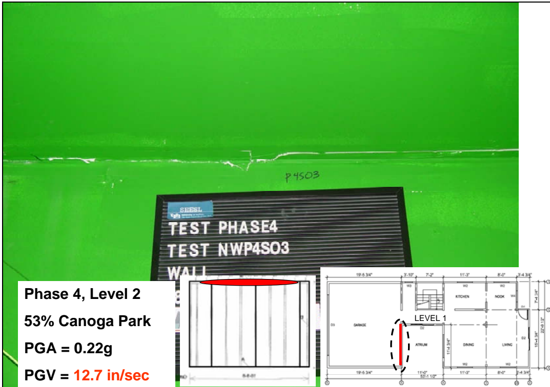
Cracking of gypsum wallboard at ceiling-wall connection
