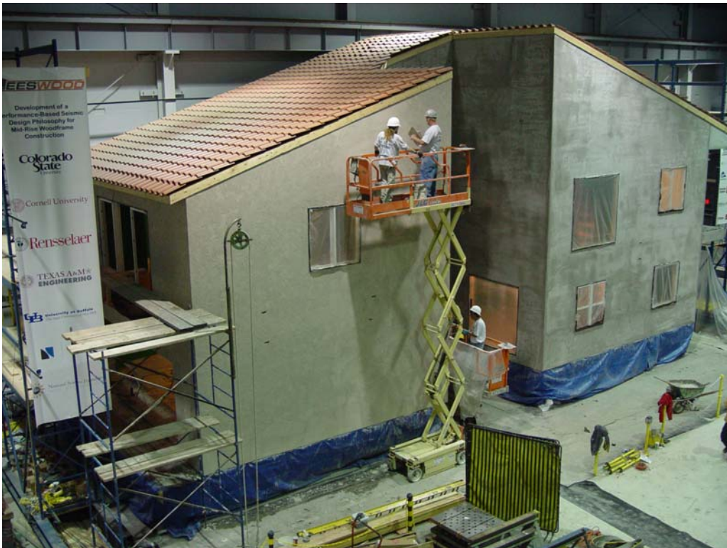
Figure 3.20: Application of the third coat of plaster on the test structure
