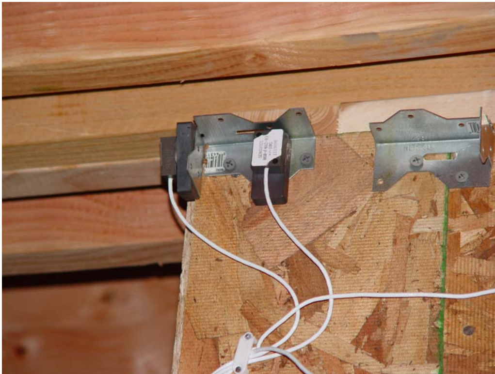
Figure 4.1: Two accelerometers at the top of a first floor wall measuring accelerations in the two horizontal directions
