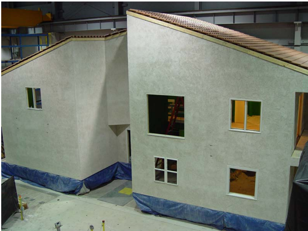
Figure 3.21: South-east external view of the benchmark structure after the installation of the exterior stucco finish
