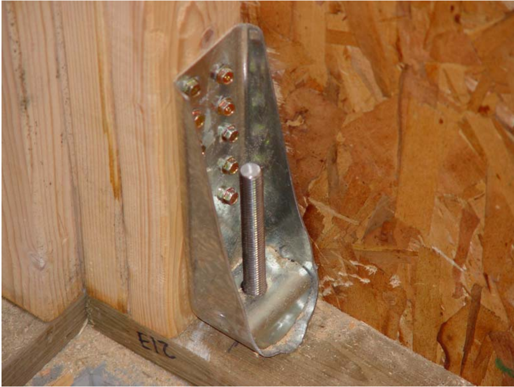
Figure 3.7: PHD2 Strong-tie Holddown installed at the bottom corner of a shear wall
