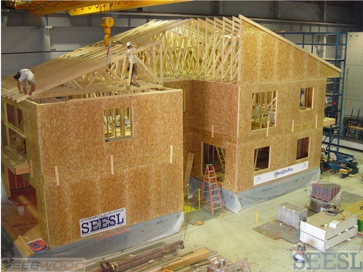
Figure 3.6: Installation of the roof trusses of the benchmark structure
