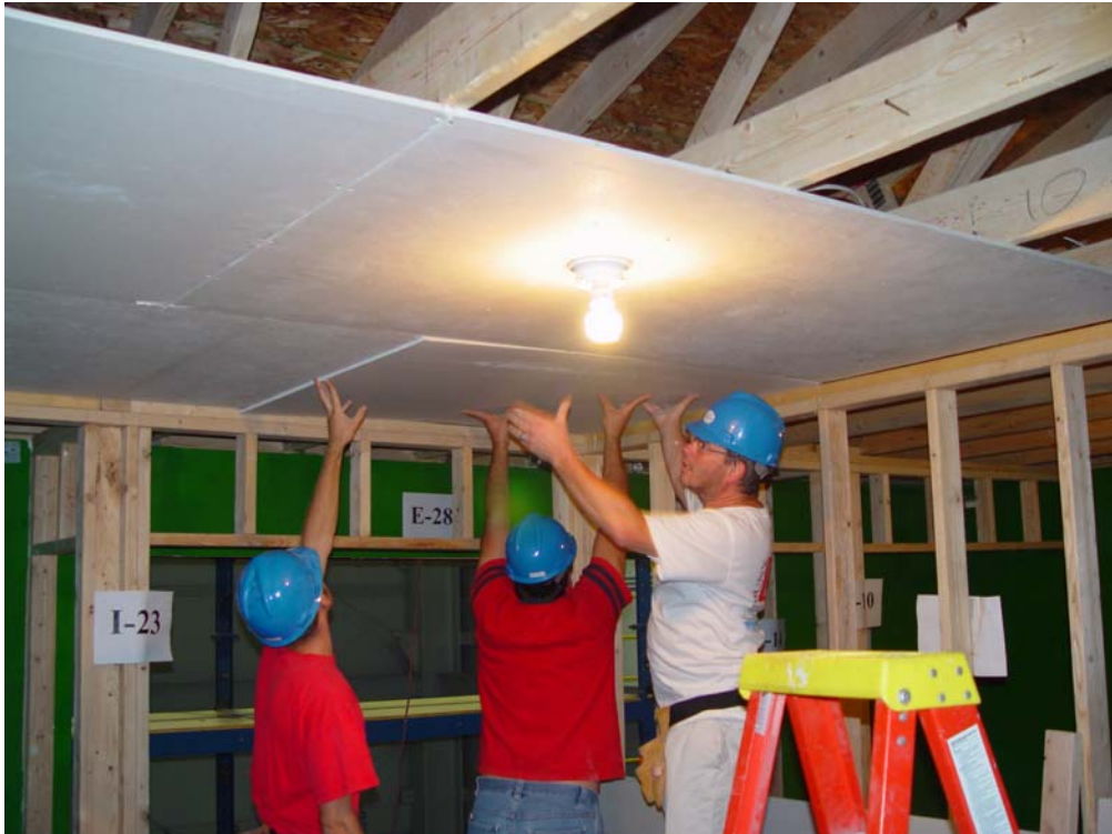
Figure 3.16: Installation of gypsum wallboard on the ceiling of the 2 nd floor
