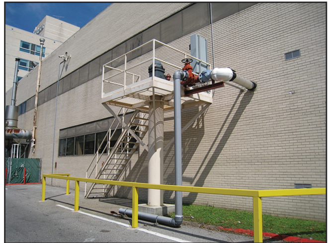
Figure 2. After Katrina, an additional well was drilled at the Ochsner Medical Center main campus in Jefferson Parish.
