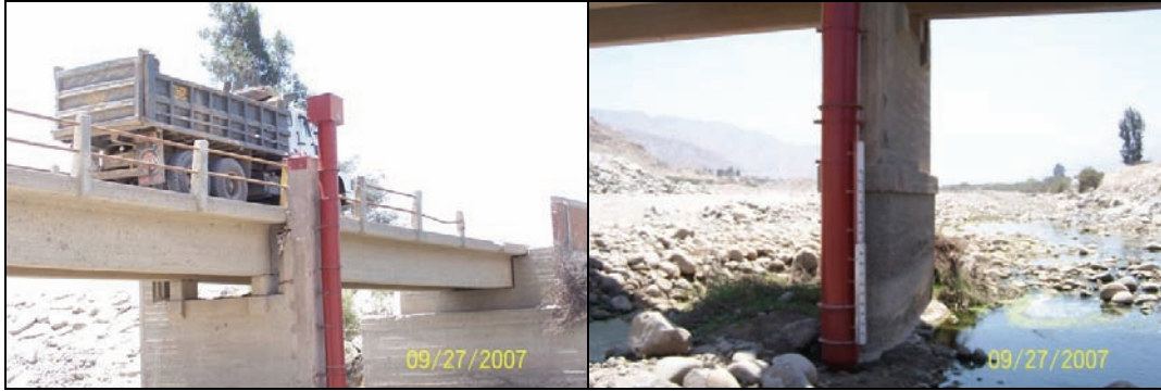
Figure 8-1. Scour Monitoring Device Mounted on a Bridge Pier to Supplement Visual Inspections
