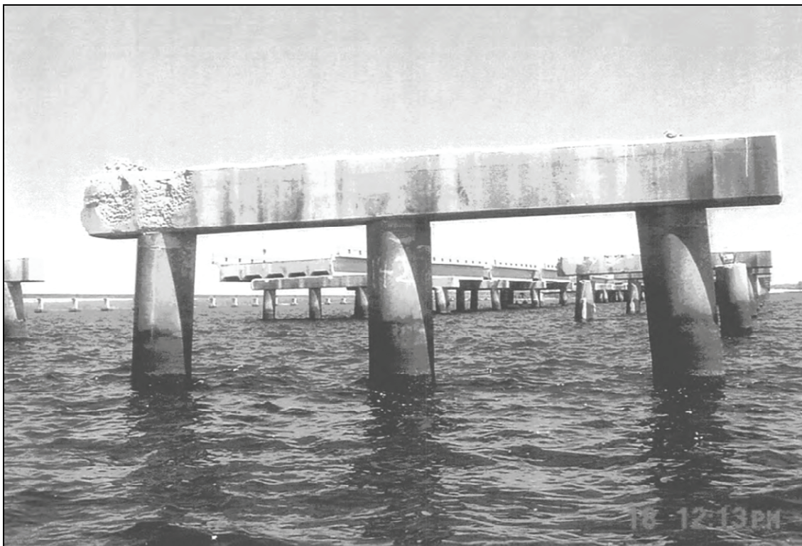
Figure 6-3. Collapsed Spans, I-10 over Escambia Bay, Florida, Hurricane Ioan
