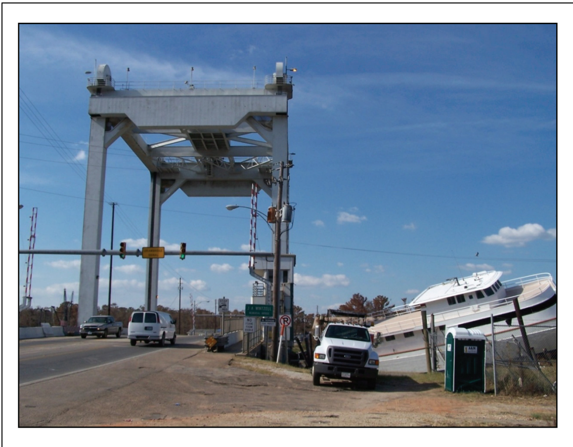
Figure 2-6. The boat on the right hit this lift bridge. The control room was also flooded.
