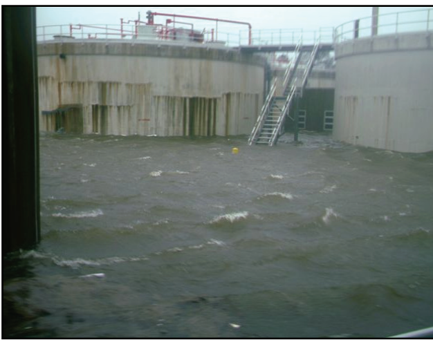
(q) A wastewater treatment plant.
