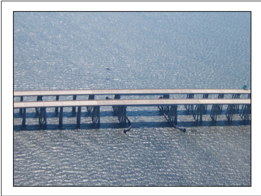
Figure 2-133. The highest spans of the I-10 bridges survived.
