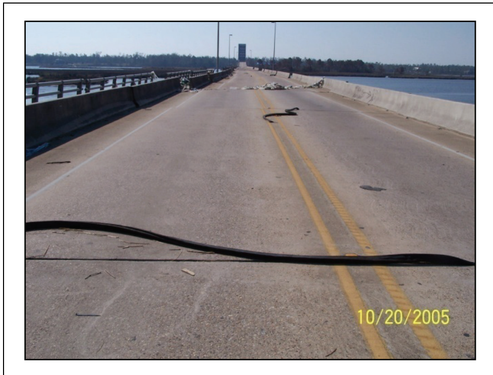
Figure 2-81. Several bridge joints had the seal blown out, indicating the possibility of pressure from entrapped air below the deck.
