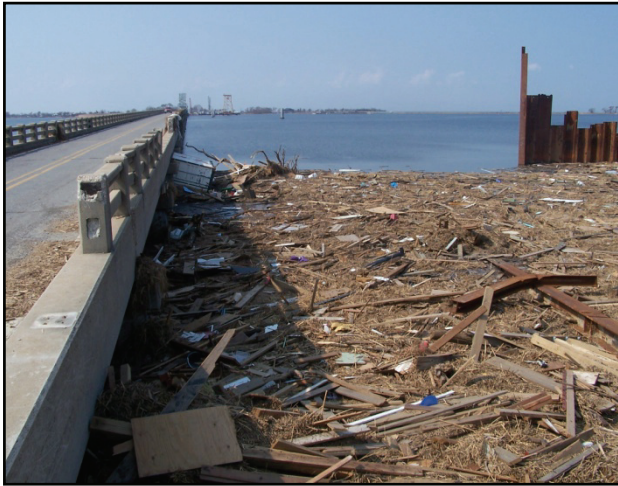
(g) Debris fields made walking hazardous.
