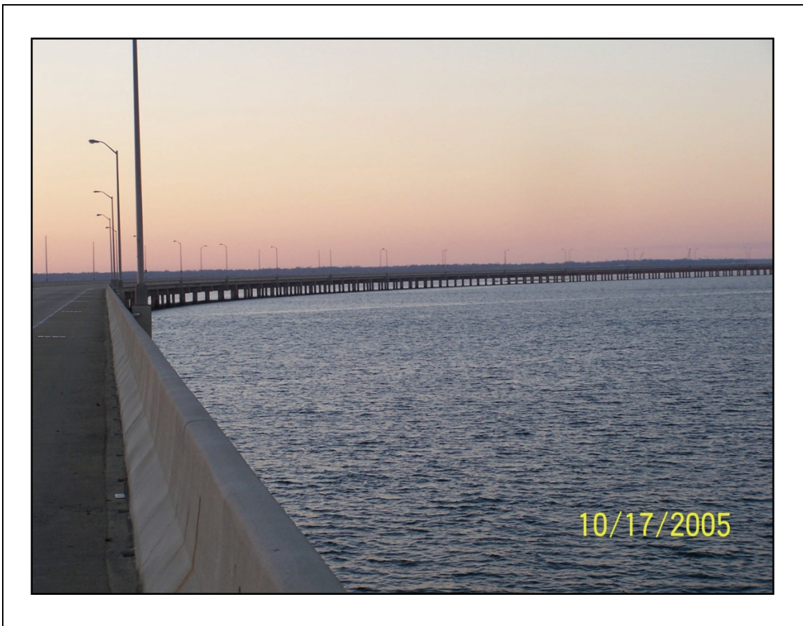
Figure 2-23. This bridge, connecting the Pascagoula Naval Station to the mainland performed well.
