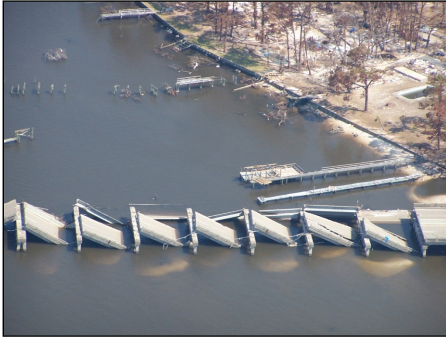
Figure 2-91. Eastern terminus of US-90 over St. Louis Bay, facing north. Lack of structural continuity contributed to the collapse of many spans in a failure pattern that is almost identical to that witnessed after earthquakes.
