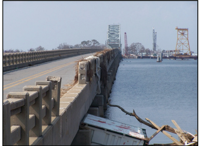
(b) Shipping containers hit bridges.
