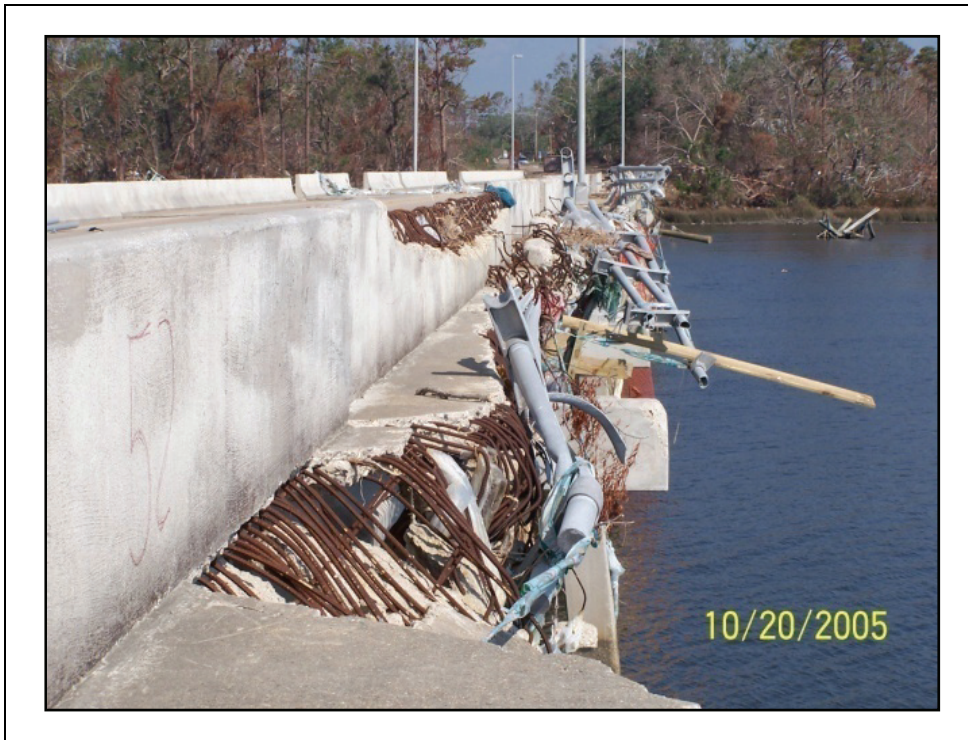
Figure 2-79. A debris dam pounding on the east fascia probably caused this damage to the concrete parapet.
