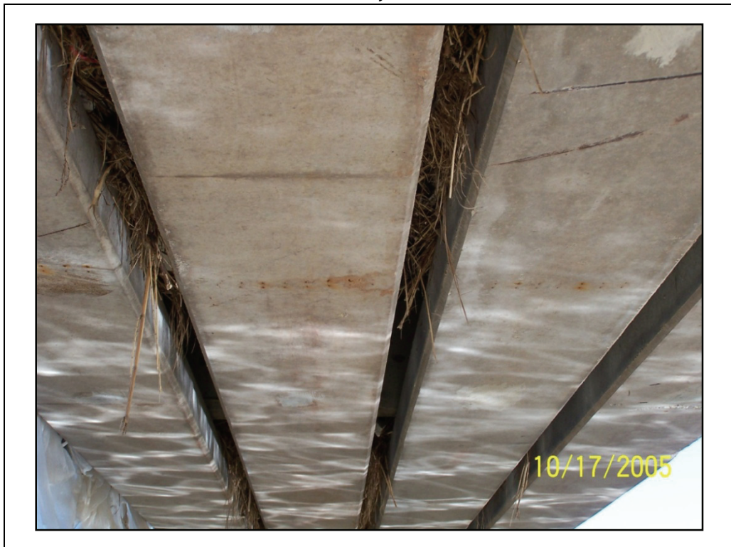
Figure 2-59. Tightly spaced prestressed beams with concrete diaphragms.
