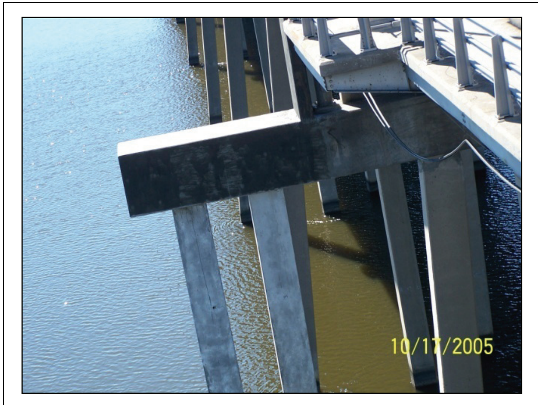
Figure 2-73. Repairs were made within a few weeks, allowing the bridge to be returned to full service.
