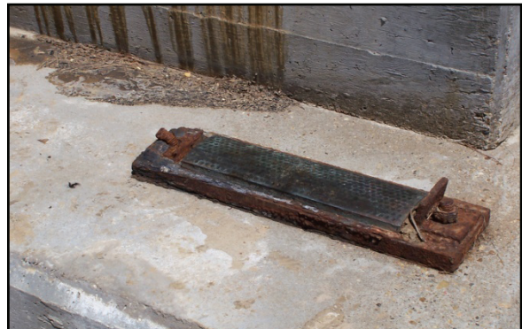
Figure 2-49. This bearing plate on the east abutment of US-90 over Biloxi Bay is typical of all bearings
