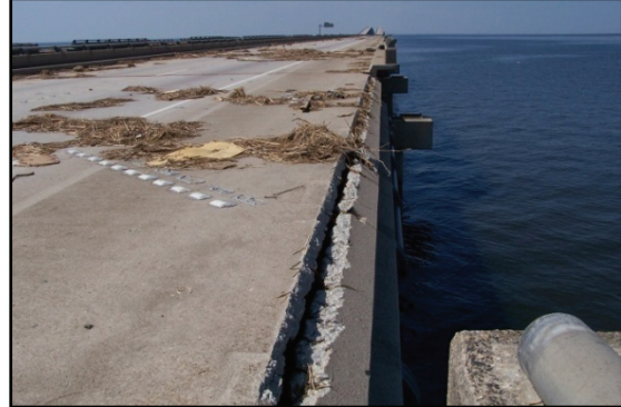
Figure 2-122. The north parapet broke off and is dangling down in the picture. Note uniform shift to the south.
