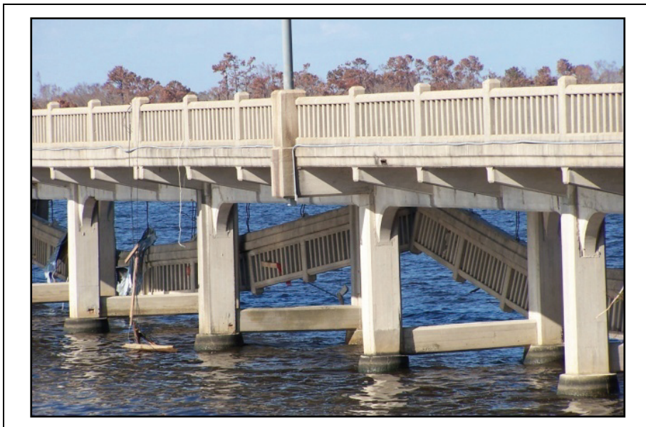
Figure 2-72. Elevation view looking NE at the old 110 over Back Bay which had been used for a fishing pier. Note the dangling concrete railing on the far (east) side.
