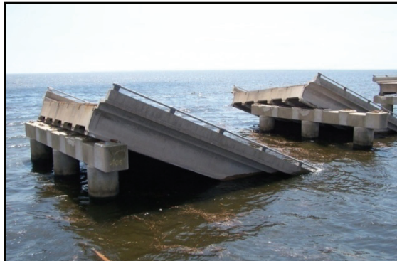
Figure 2-126. Span units of the EB bridge dropped.
