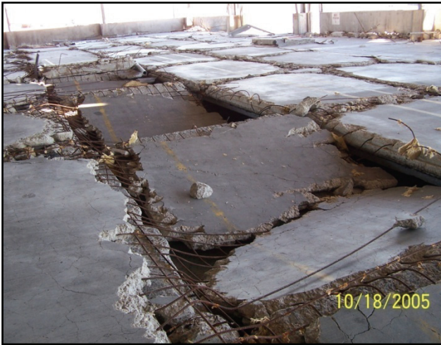
(o) Warehouse slab at the Port Authority.
