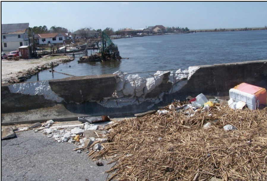
Figure 2-149. The north side of the approach barrier was hit.
