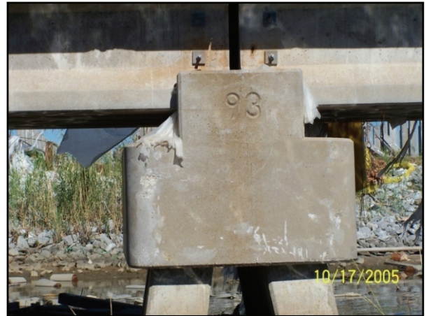
Figure 2-61. A simple concept, like permanently inscribing the pier number in the concrete, makes for positive identification and clear communication. This undoubtedly served the owner well when during repair operations as well as being useful during reconnaissance surveys.
