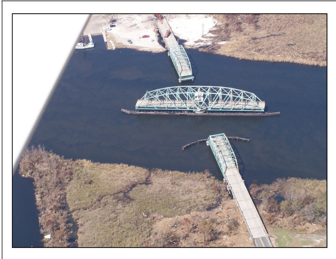
Figure 2-106. US-90 at East Pearl River; facing west.
