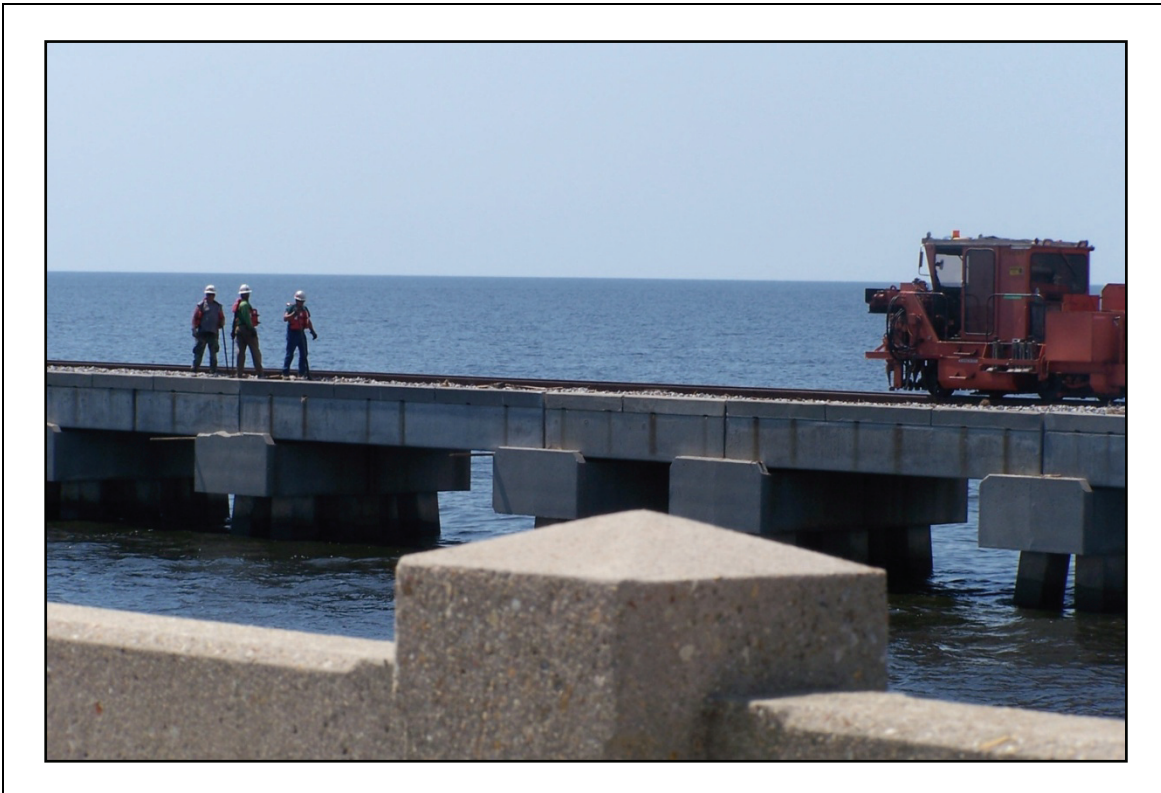
Figure 2-138. Norfolk-Southern had a crew relaying track about a week after the storm.
