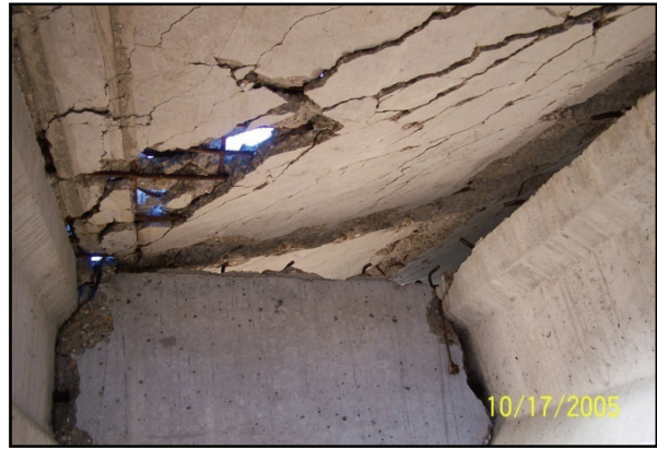
Figure 2-45. A view of the deck underside.
