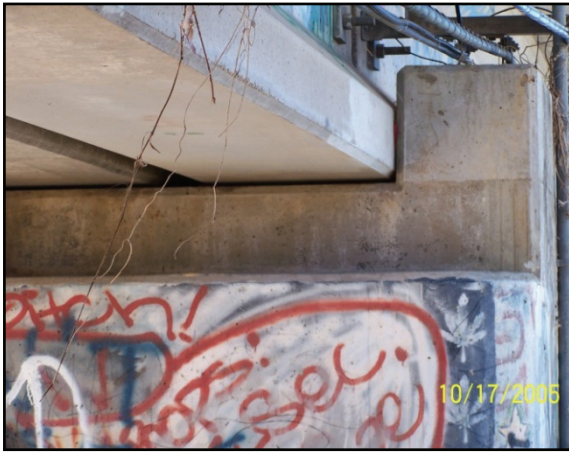
Figure 2-60. Massive shear blocks on each side of the superstructure successfully restricted horizontal forces imposed by wind and waves.
