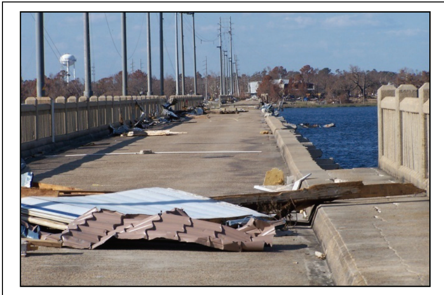
Figure 2-71. Looking north onto old 110 over Back Bay. Note the missing sidewalk and railing on the east side.
