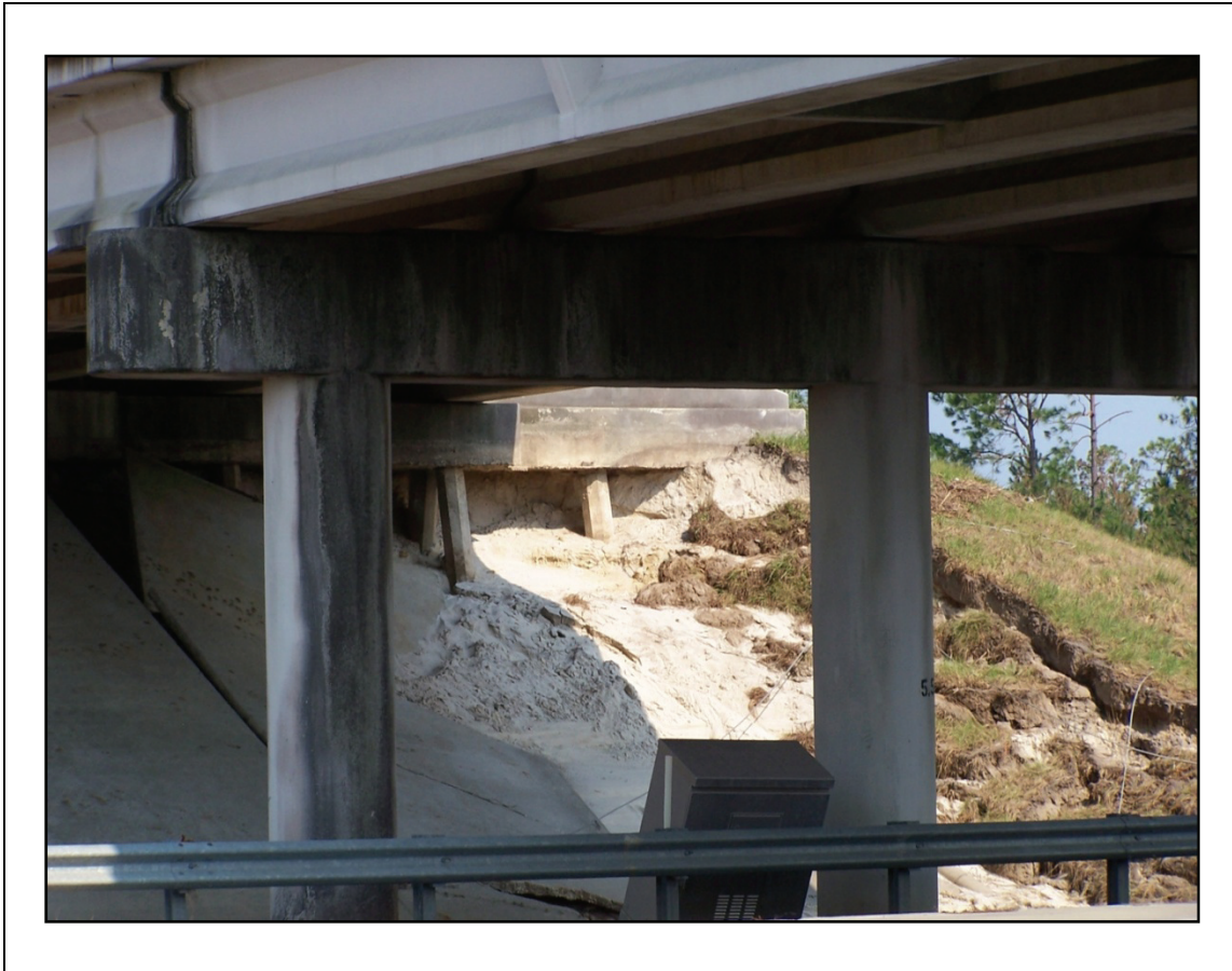
Figure 2-85. Scour is usually associated with water crossings, but this bridge over a road saw scour.
