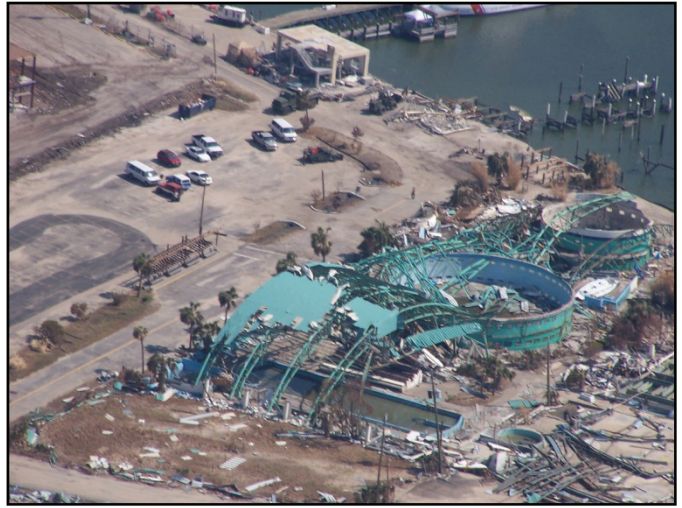
(n) Destroyed buildings.
