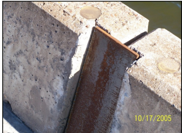
Figure 2-63. Though not anchored into the concrete, the tight-fitting steel joint plate probably acted as a shear key to resist relative horizontal displacement and restrain rotation between spans.
