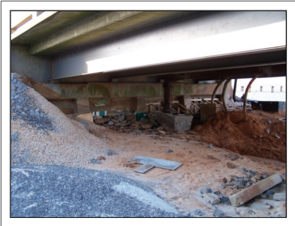
Figure 2-12. Erosion at the west abutment.
