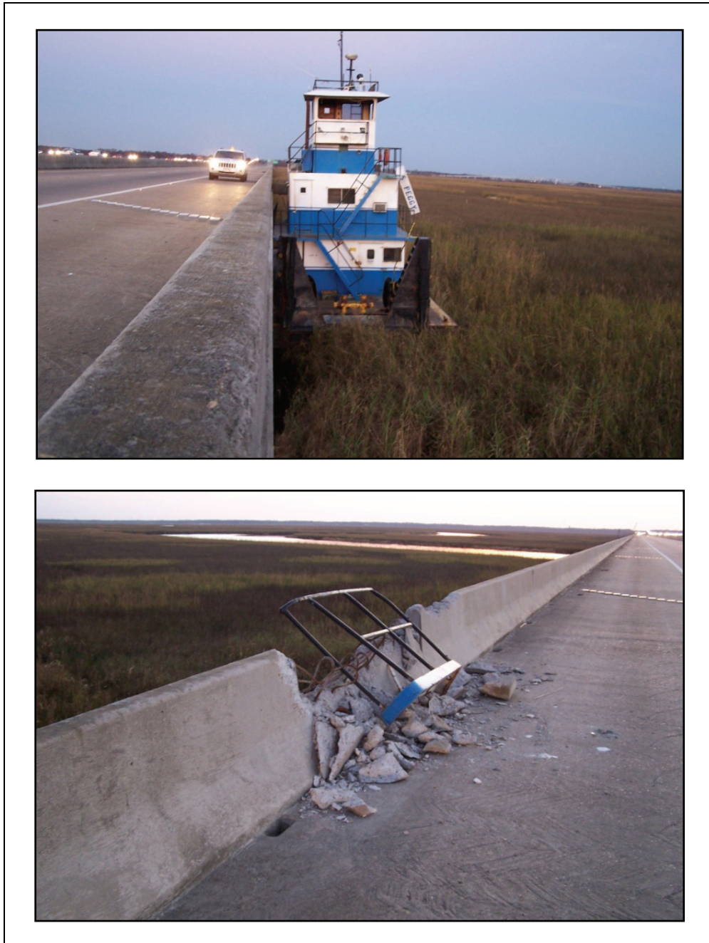
Figure 2-29. I-10 EB suffered multiple hits.
