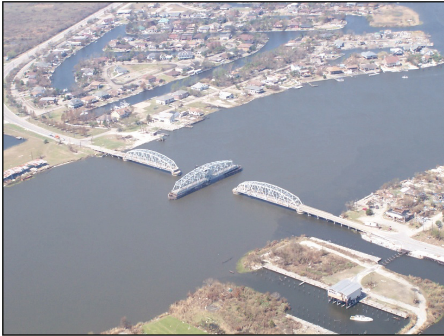
Figure 2-148. Facing NW. The swing span became inoperable.
