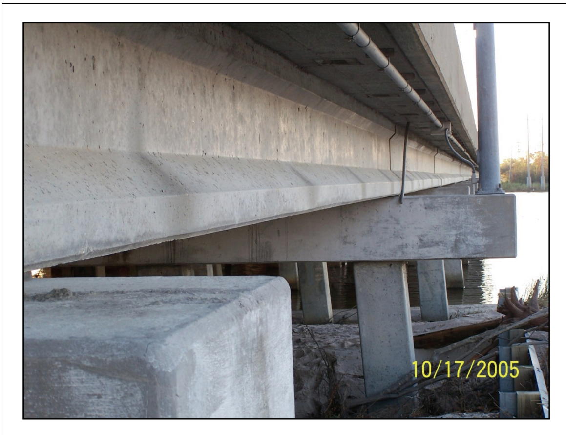
Figure 2-21. P/S concrete beams on concrete piers.
