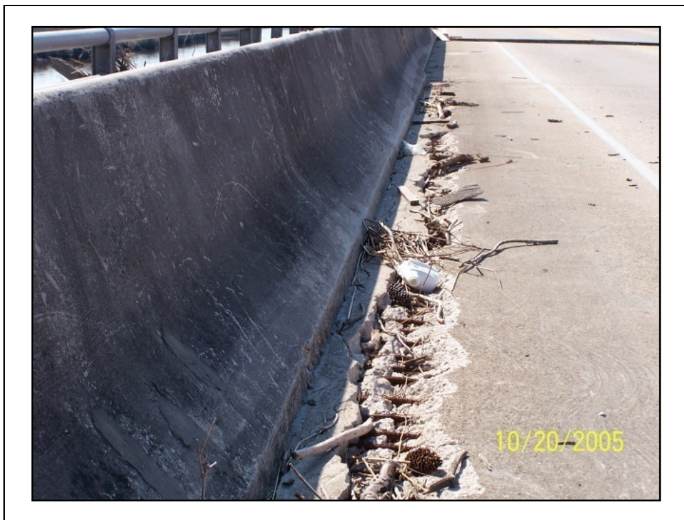
Figure 2-78. Hydraulic pressure on the backside of this barrier probably caused the spalling found at its toe. This photo is along the east fascia of the bridge.
