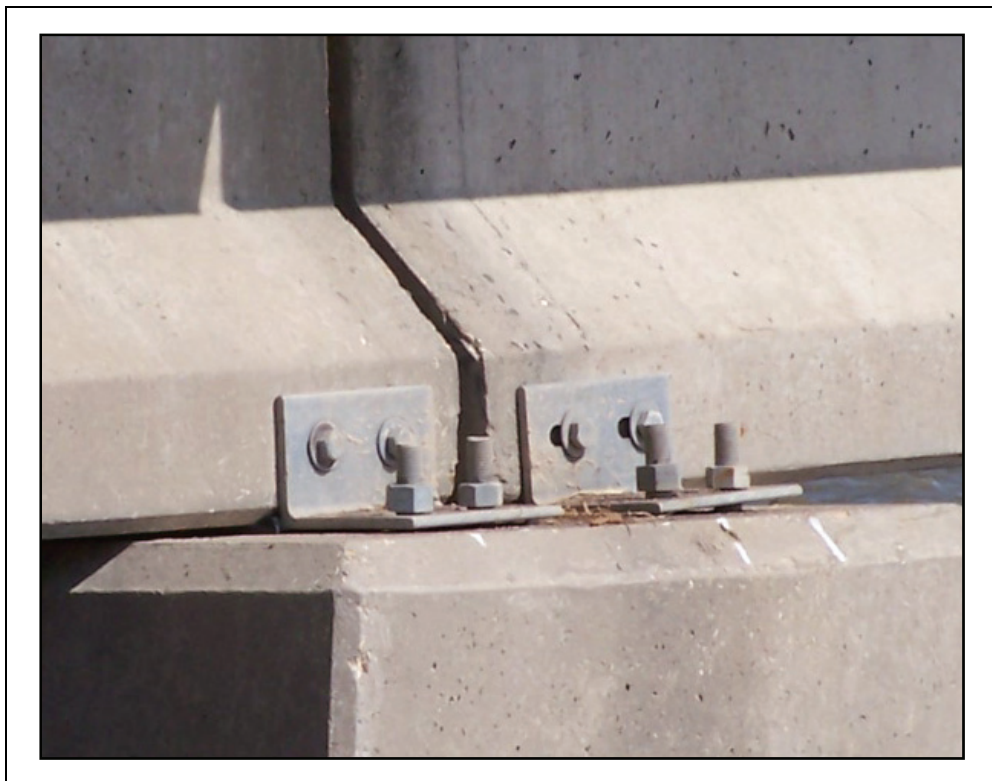
Figure 2-5. Tie down detail between the P/S beams and pier cap.
