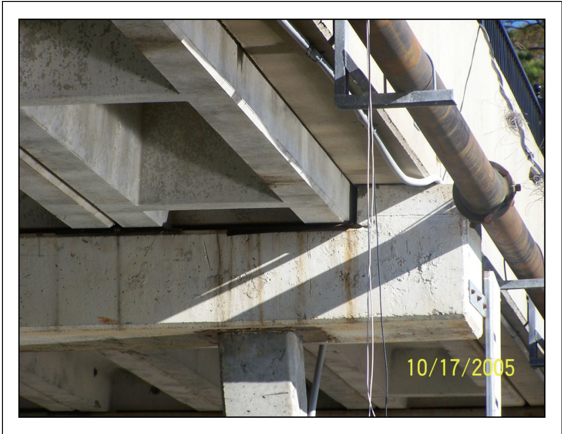
Figure 2-66. The shear block at the end of the pier cap restrained the precast superstructure units.
