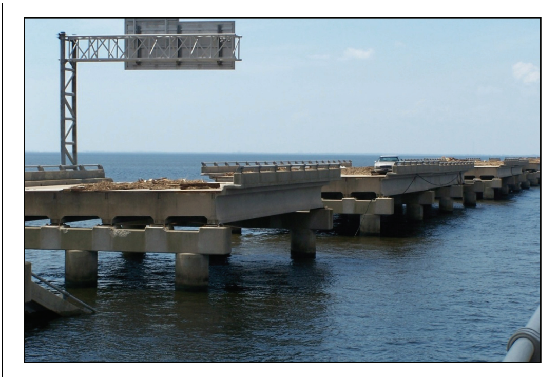
Figure 2-120. I-10 EB facing west.
