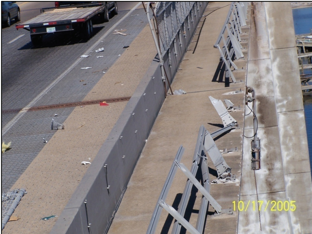
Figure 2-74. The metal railing on the east fascia of the span that carries I-110 over the navigation channel of Back Bay of Biloxi was damaged by boats or debris carried by the surge.
