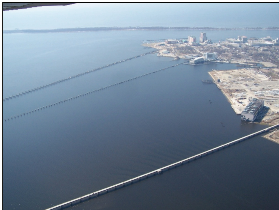
(b) Biloxi Bay, facing south toward the City of Biloxi. From top to bottom, the bridges are US-90, old route 90, and the CSX railroad.
