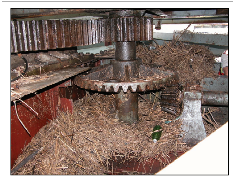
Figure 2-152. Typical debris buildup in the gear mechanism of a moveable bridge.
