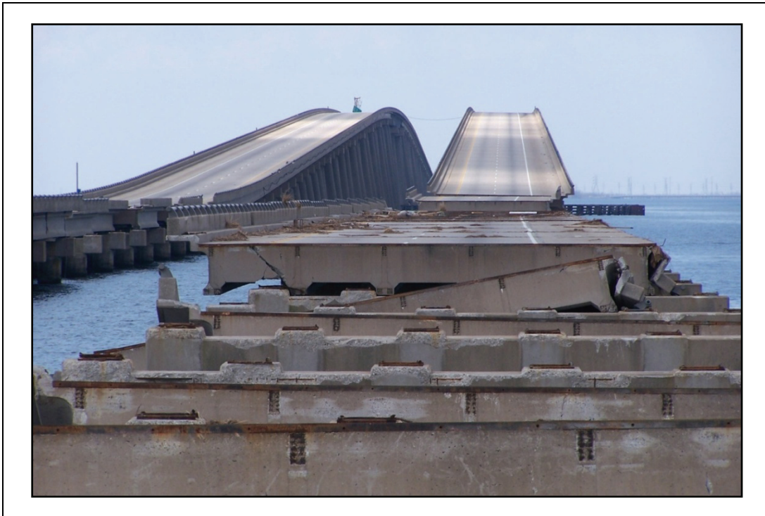
Figure 2-119. I-10 WB, facing west to the high-rise spans over the navigation channel. Note the scrape marks on the pier caps, caused by the falling spans.
