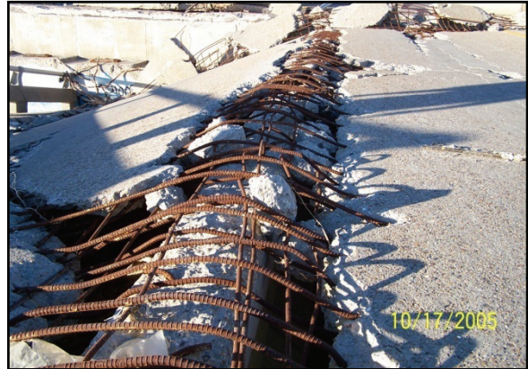
Figure 2-47. Steel reinforcing bars is all that remains of the concrete deck above the concrete girder. This photo was taken at the west end of the US-90 bridge.
