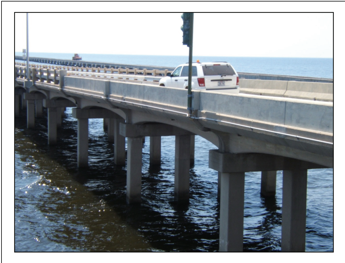
Figure 2-135. Though older and lower, US-11 performed better than I-10.
