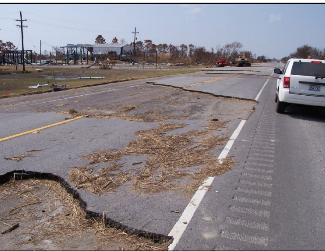
(e) Courses of asphalt pavement peeled up.
