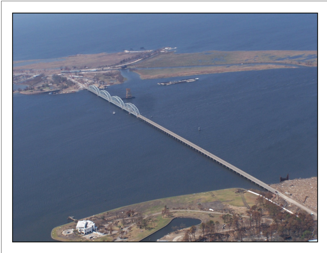
Figure 2-146. Rigolets Bridge carries US-90 This photograph was taken facing west.
