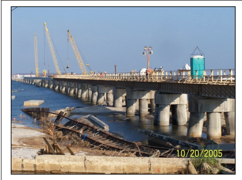
Figure 2-99. By October 20, repairs the CSX bridge had already begun. In the foreground, on the north side of the bridge, the tracks that had been washed off can be found.
