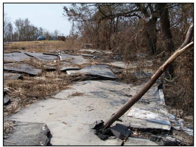
(f) Layers of pavement moved 50-100 feet.
