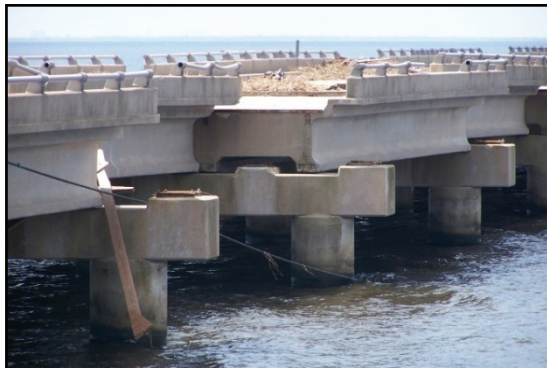
Figure 2-132. Span units are relatively intact.
