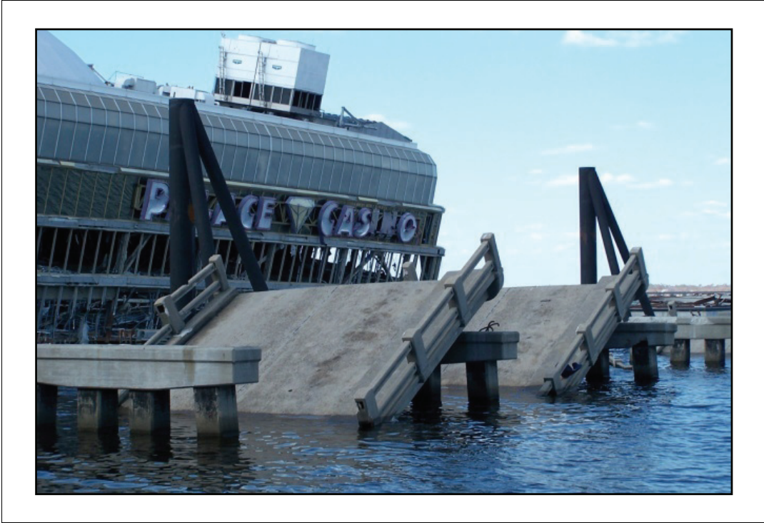
Figure 2-51. Looking east from the west end of old route 90.
