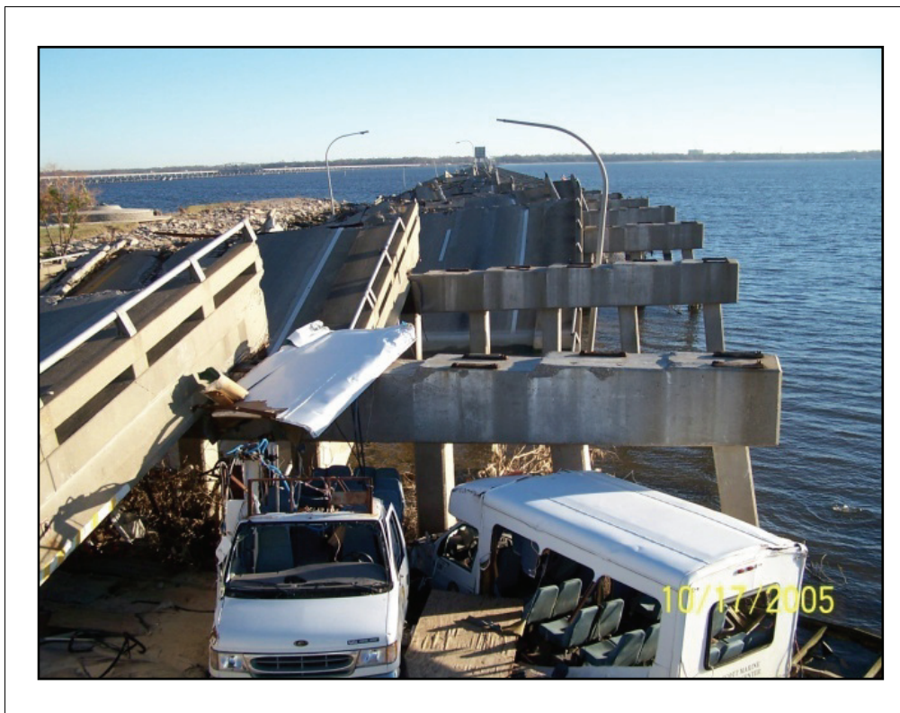
Figure 2-40. Floating debris such as vehicles and shipping containers also caused damage to bridges. This photo was taken at the west end of the US-90 bridge.
