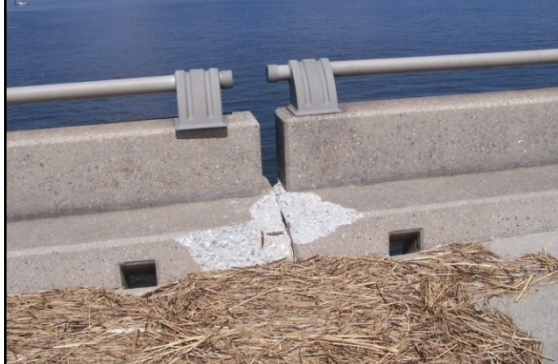
Figure 2-124. The wave action exerted on the spans must have been violent as evidenced by the spalled concrete resulting from longitudinal pounding between spans.
