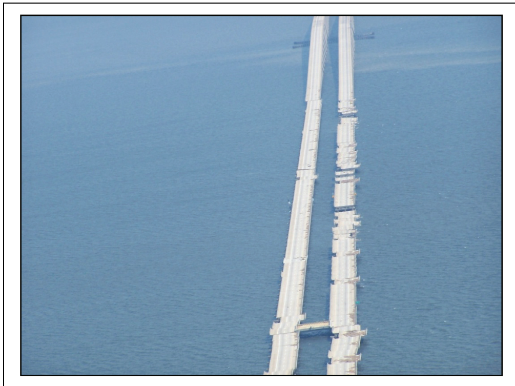
Figure 2-116. I-10 WB & EB, showing numerous displaced spans.
