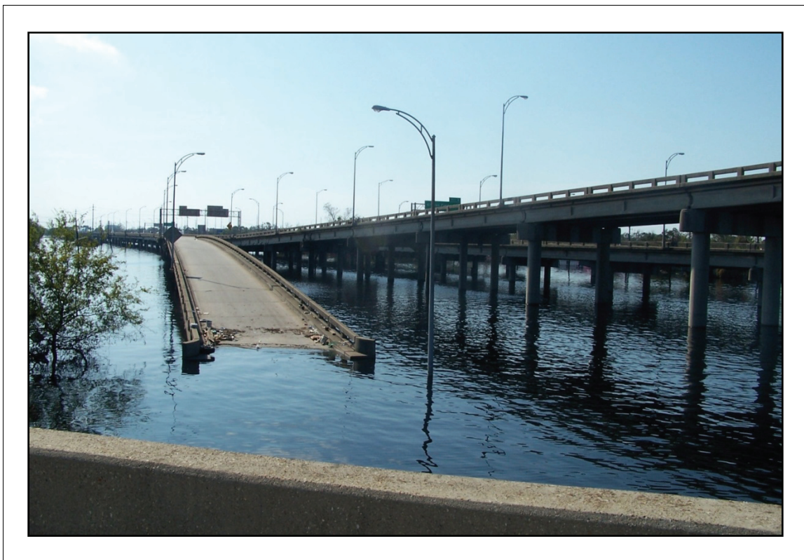
Figure 2-139. On the date of this photo (September 8, 2005), many ramps in the city of New Orleans were flooded and not useable except as a boat launch.
