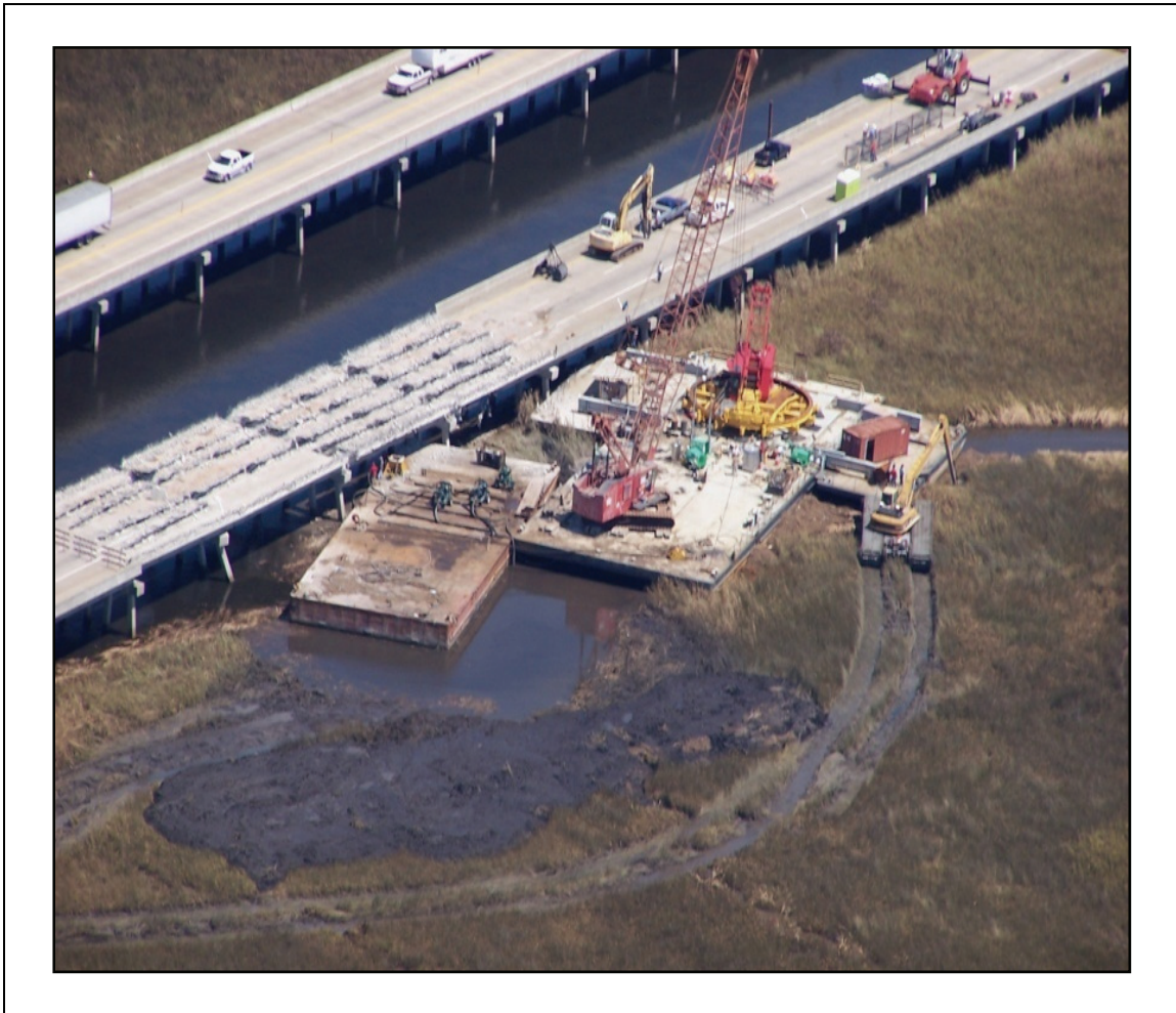
Figure 2-26 The concrete deck was being removed from the I-10 EB bridge on September 11, 2005.
