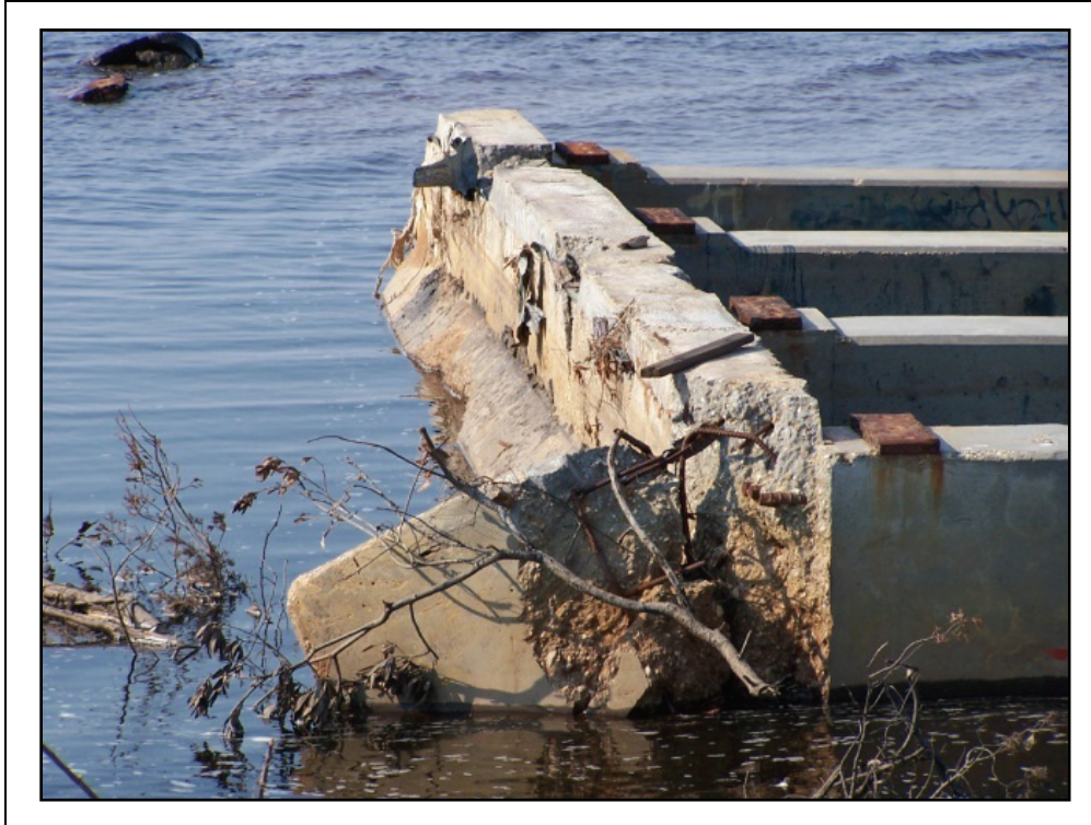
Figure 2-96. The north side of the westernmost span was flipped over and thrown 100 feet.
