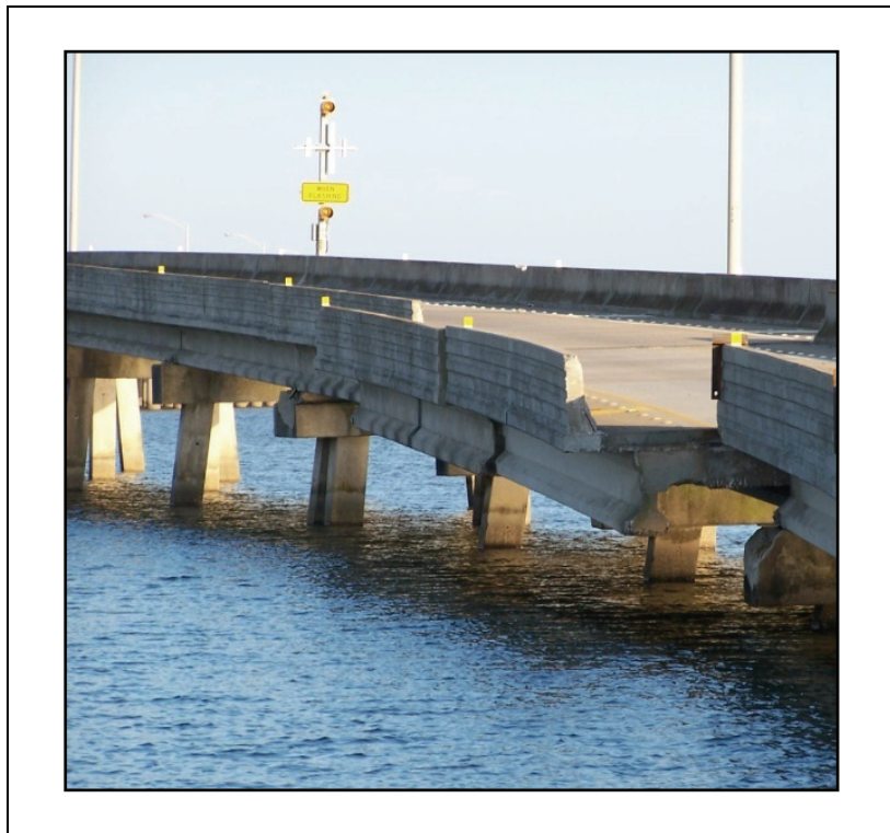
Figure 2-16. Facing east toward spans that were pushed to the north.
