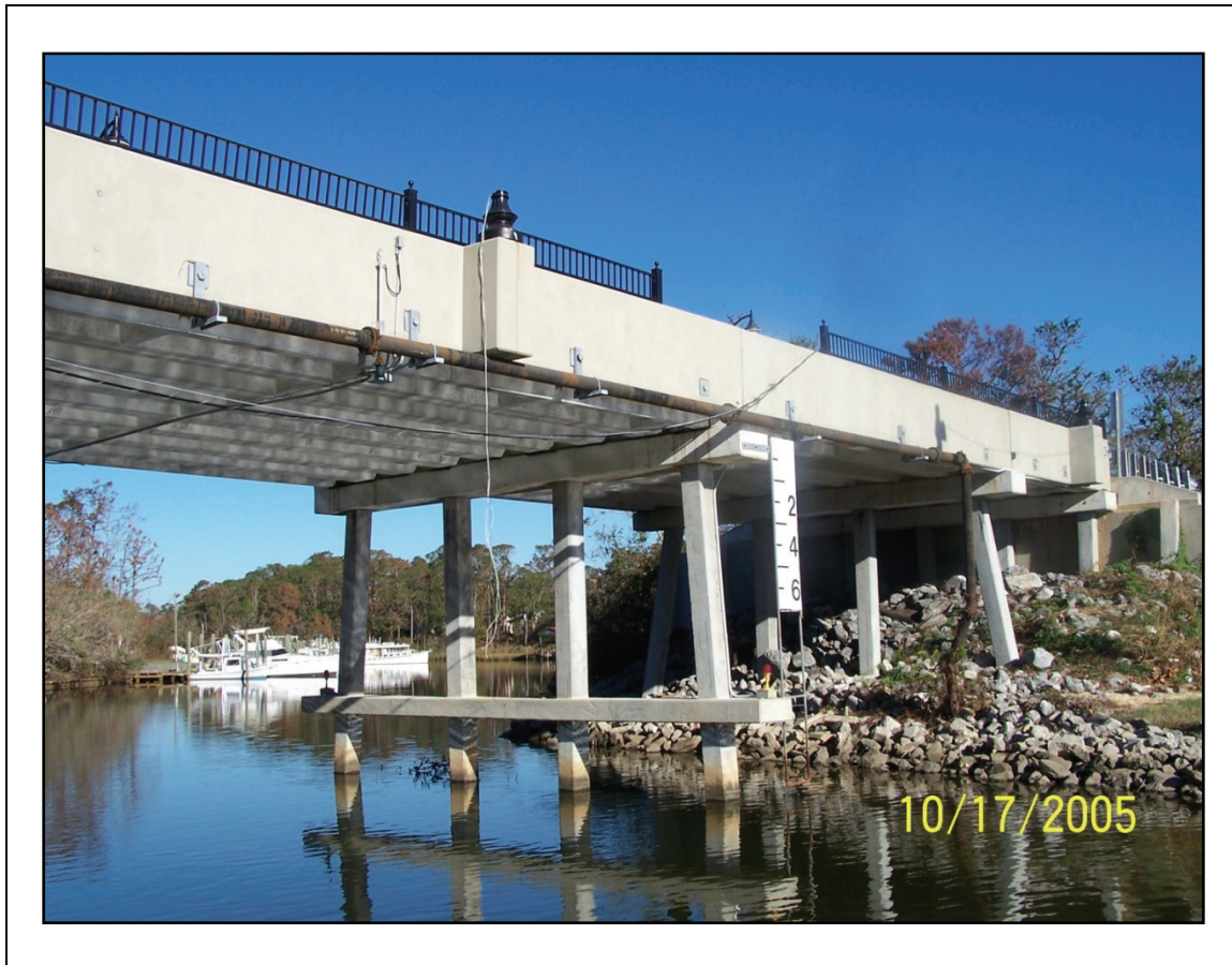
Figure 2-64. The Shearwater bridge is very close to Biloxi Bay and was submerged under water.
