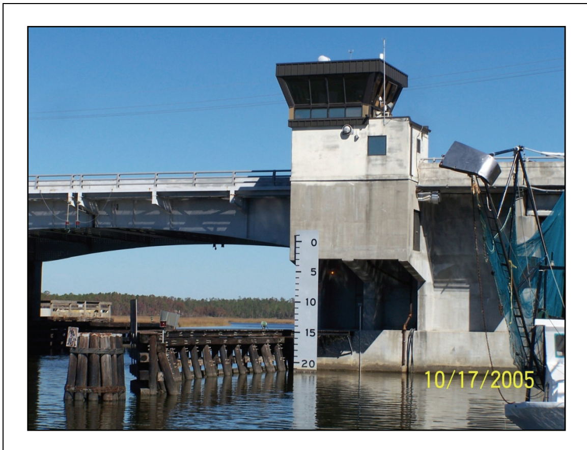
Figure 2-67. The mechanical room of this moveable bridge flooded, making the bridge inoperable.
