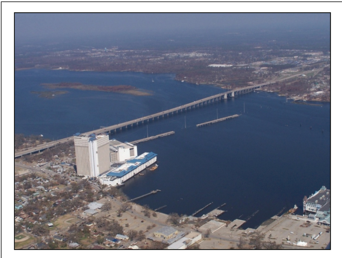
Figure 2-69. This photograph was taken facing NW. A hotel and floating casino are shown in the foreground. Near it is the bridge referred to as old route 110, with several sections missing. I-110 at the top of the picture was hit by a barge and debris but remained functional.
