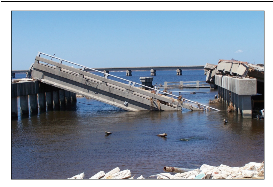
Figure 2-36. Although both were subjected to essentially the same conditions, there was a remarkable difference in performance between the US-90 (foreground) and CSX bridges (background).
