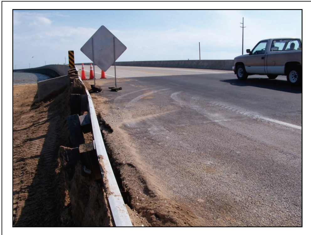
Figure 2-4. Approaches had been partially washed out.
