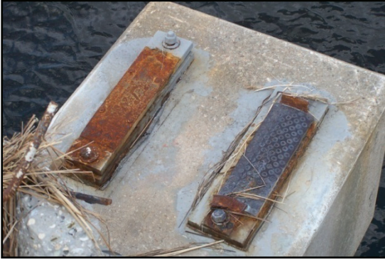
Figure 2-121. Bearings were not designed to provide resistance to uplift or lateral loads.
