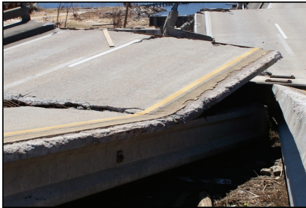
Figure 2-46. The 7 inch CIP composite deck has been peeled away from the P/S concrete beam and has broken transversely, exposing its steel reinforcement. This photo was taken at the east end of the US-90 bridge.
