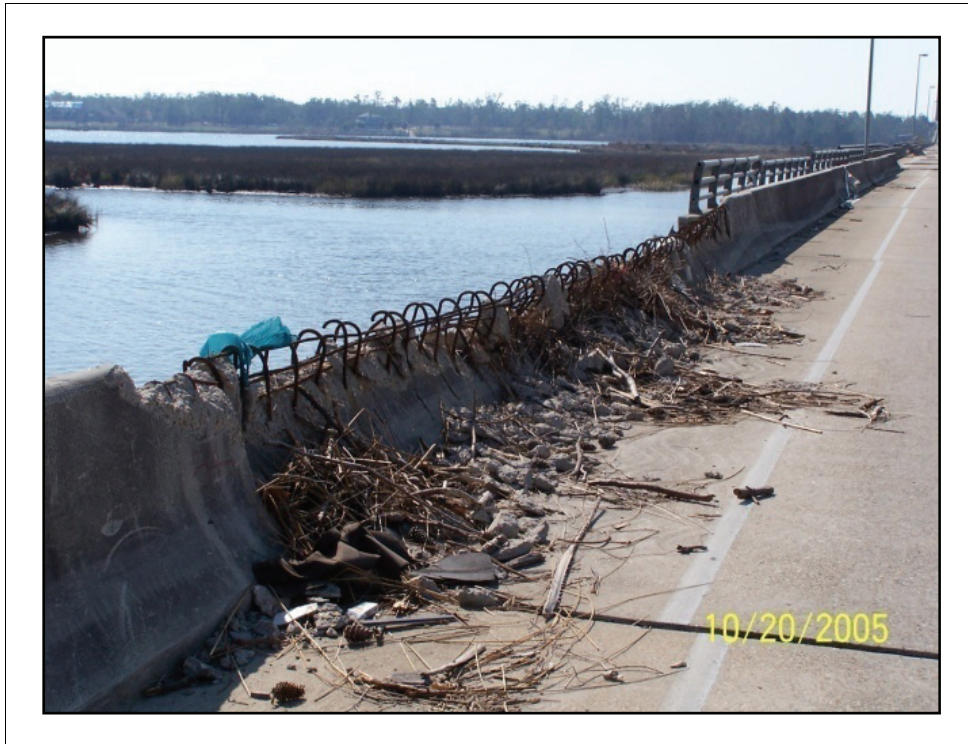
Figure 2-79. A debris dam pounding on the east fascia probably caused this damage to the concrete parapet.
