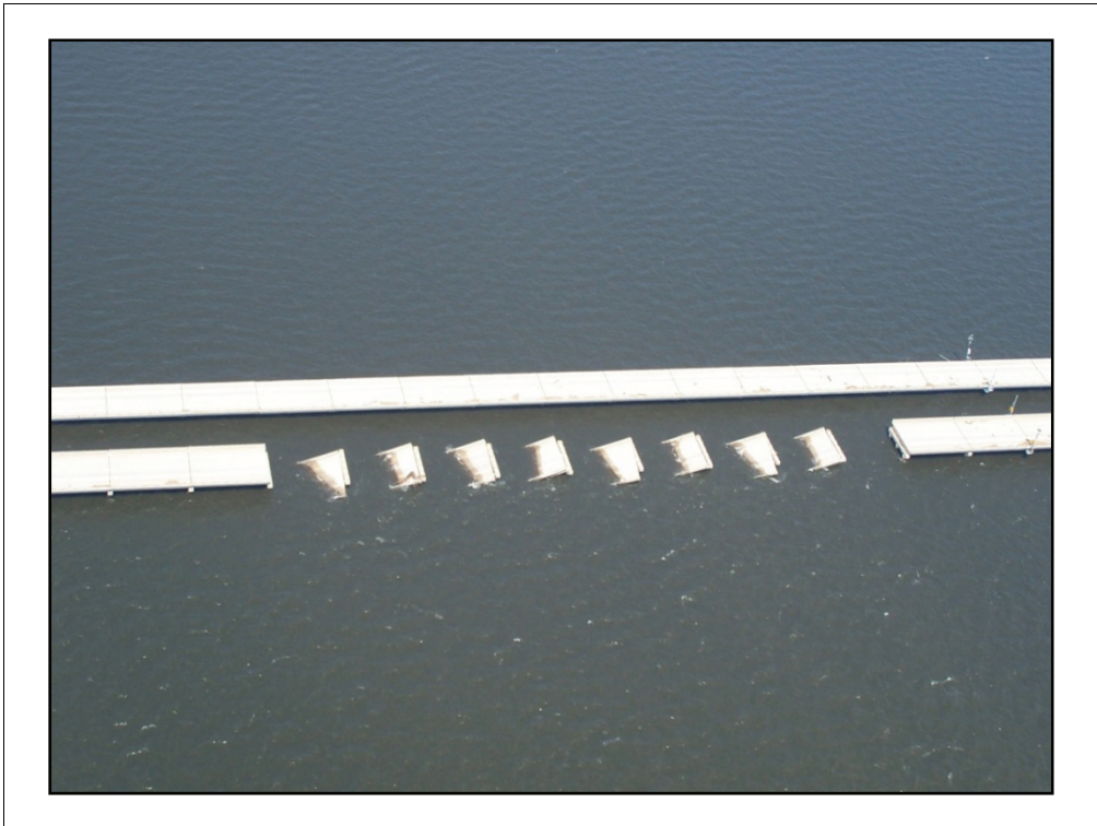
Figure 2-118. The missing span on the far right seems to have slid out, causing the others to topple.
