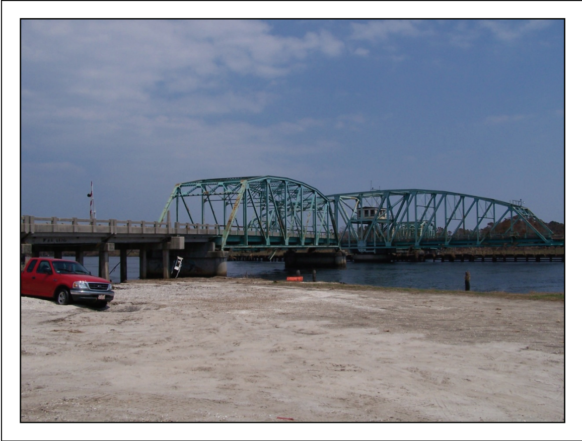
Figure 2-107. US-90 over East Pearl River
