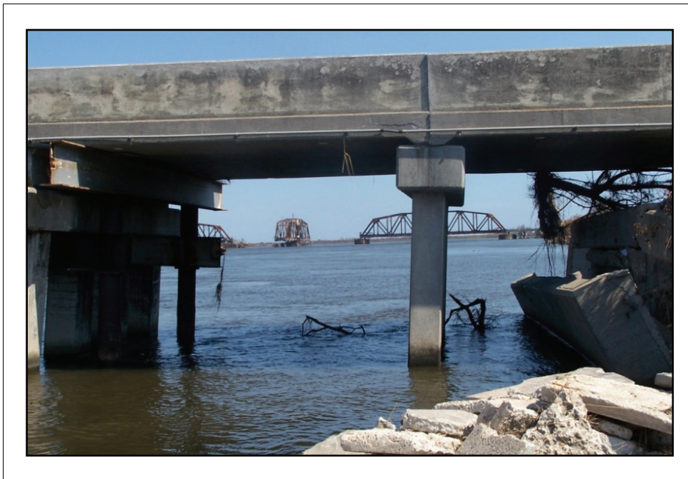
Figure 2-151. A tipped pier indicates that scour has occurred.
