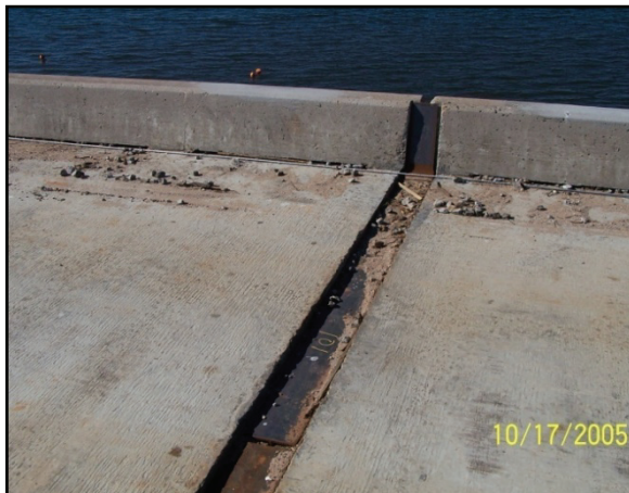
Figure 2-62. This steel plate prevents debris from falling through the joints between spans but also tightens up the superstructure assembly to restrict movement.
