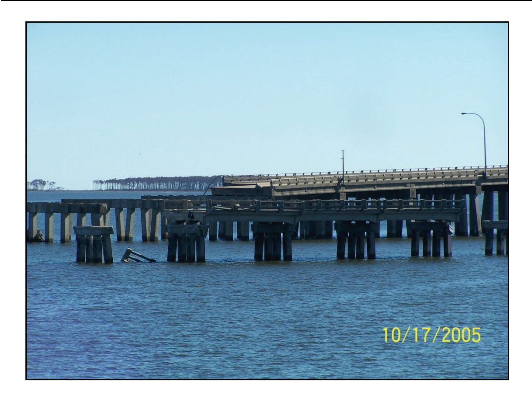
Figure 2-52. Facing south at old route 90 with the higher spans of US-90 near the navigation channel behind it.
