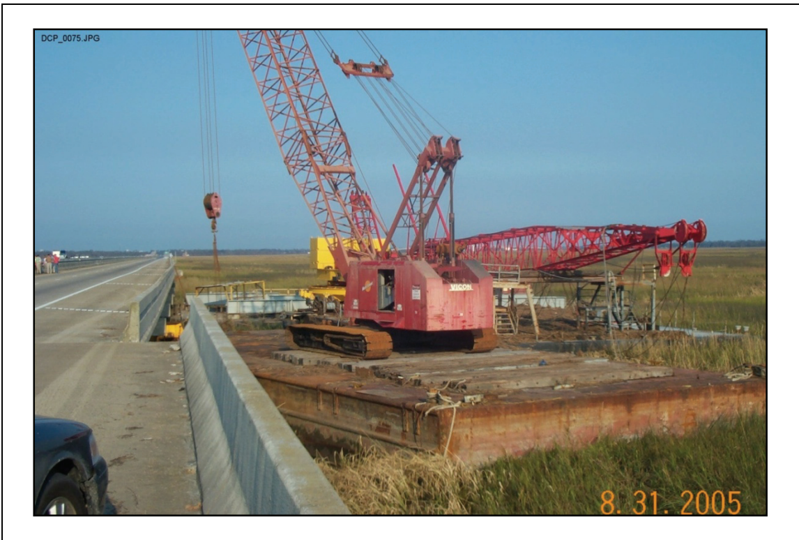
Figure 2-28. I-10 EB was hit by this barge and pushed four feet to the north.
