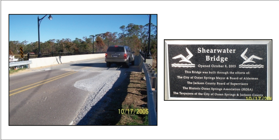
Figure 2-65. Approach erosion was easily repaired.
