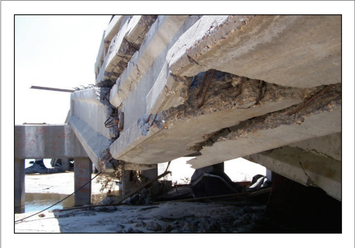
Figure 2-43. Uplift forces probably helped destroy this beam.
