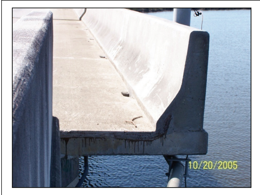
Figure 2-77. Spans shifted horizontally on the pier caps as much as three feet. This photo was taken looking south at the west fascia.
