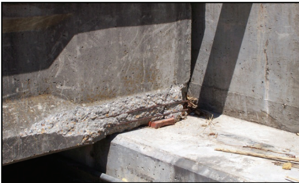
Figure 2-48. Note the bearing plate under the end of the P/S concrete beam. This beam slide to the north (left), bending down the retainer angle and anchor bolt seen in Figure 2-49.
