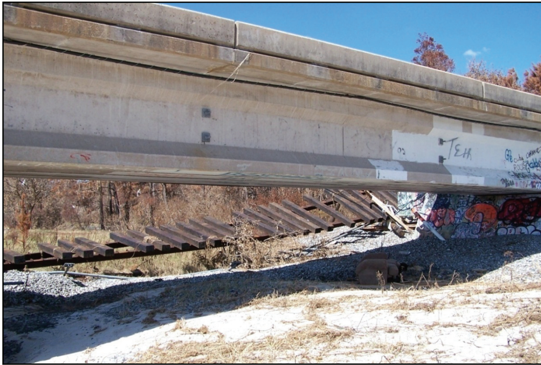
Figure 2-55. The tracks near the east end are upside down on the north side.
