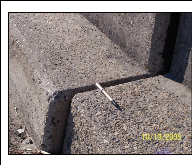
Figure 2-108. There was minor misalignment of the curb on the east side of the bridge.
