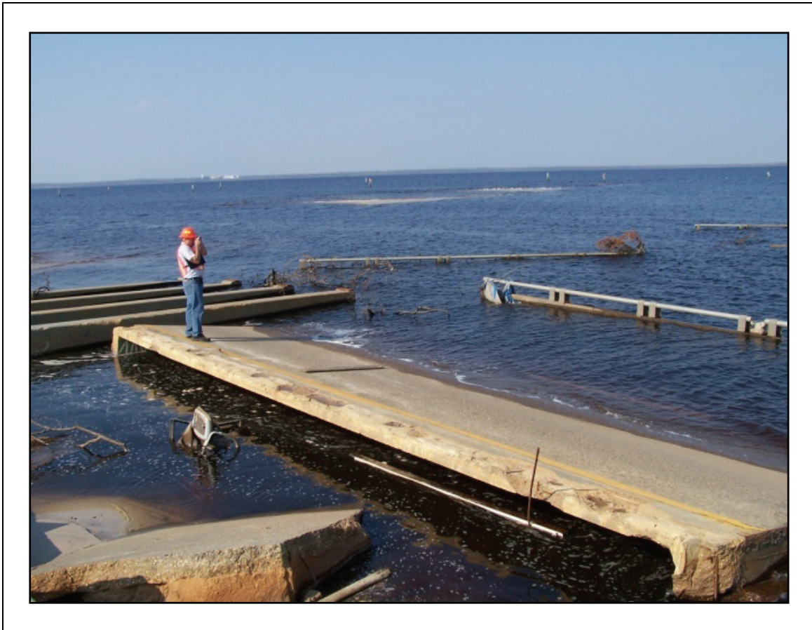
Figure 2-95. This precast span unit was tossed off the pier and rotated 90 degrees.
