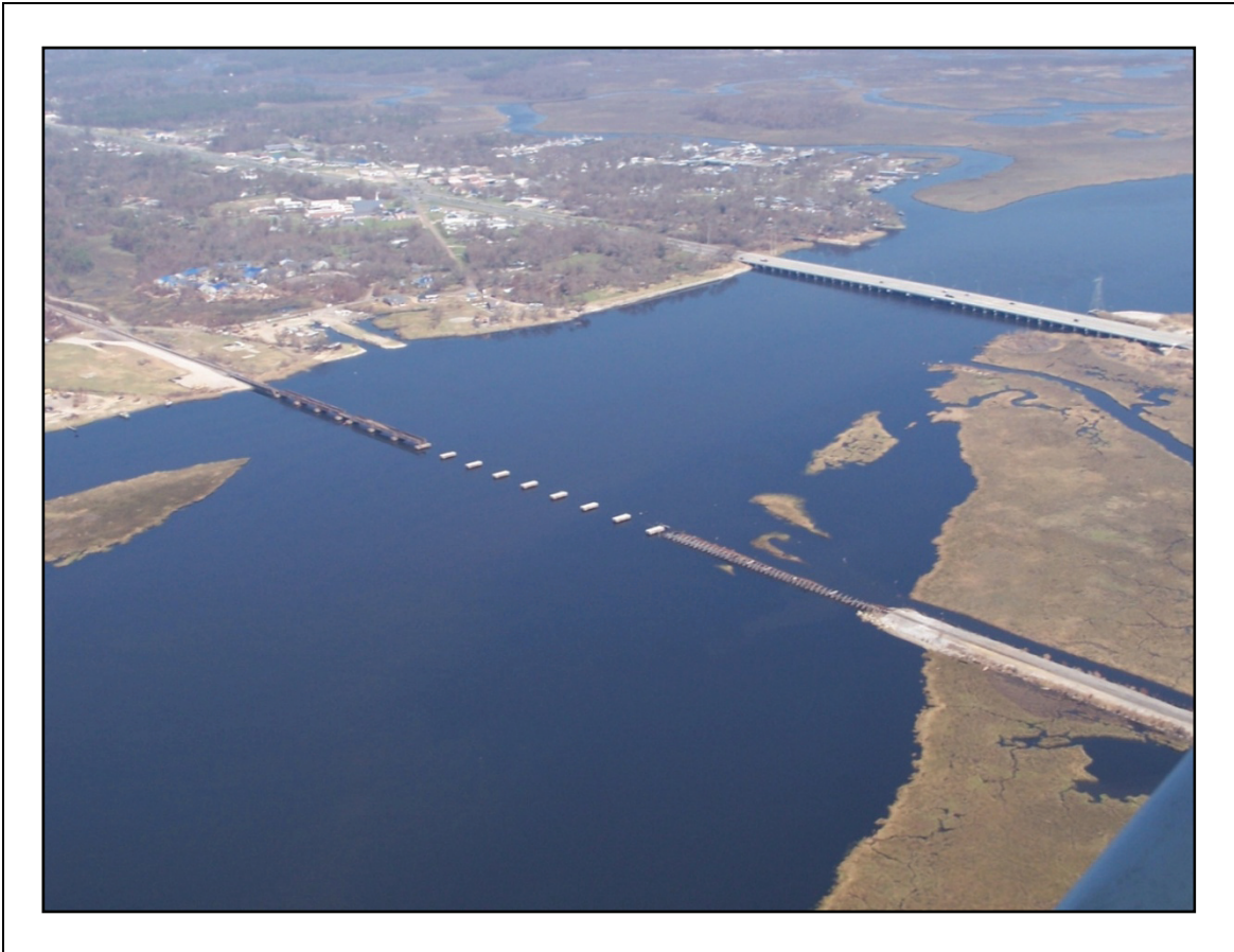
Figure 2-22. CSX railroad bridge lost the tracks and superstructure. US-90 is in the background.
