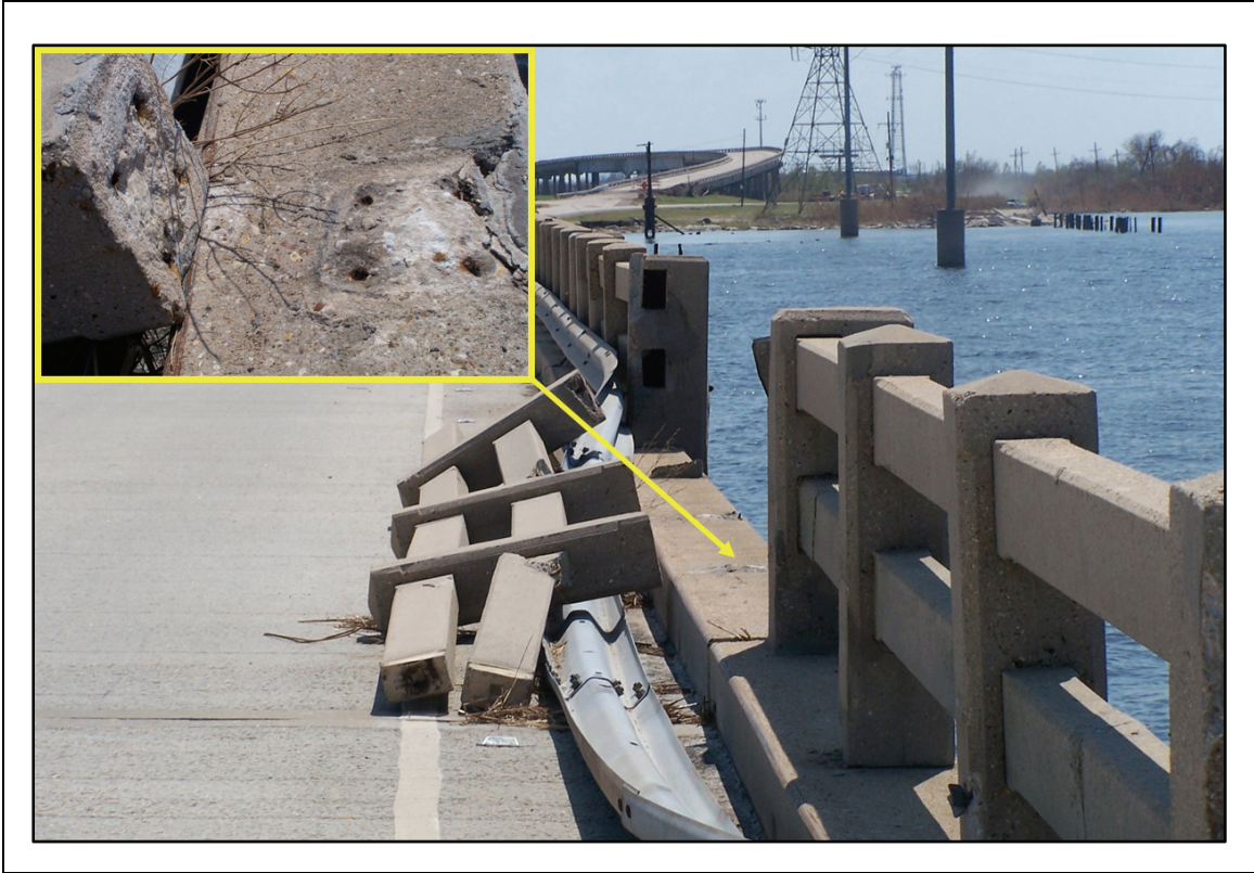
Figure 2-137. This section of concrete parapet on US-11 failed from wave force but was already in a weakened state from corrosion prior to the storm. Corrosion in the concrete barrier contributed to its failure from wave action. A subsequent investigation by LADOTD led to plans for replacement of all of this barrier.
