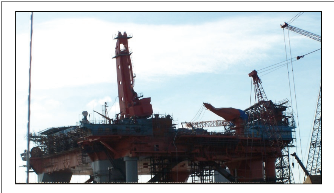
Figure 2-9. 13,000 Ton oil platform PSS Chemul
