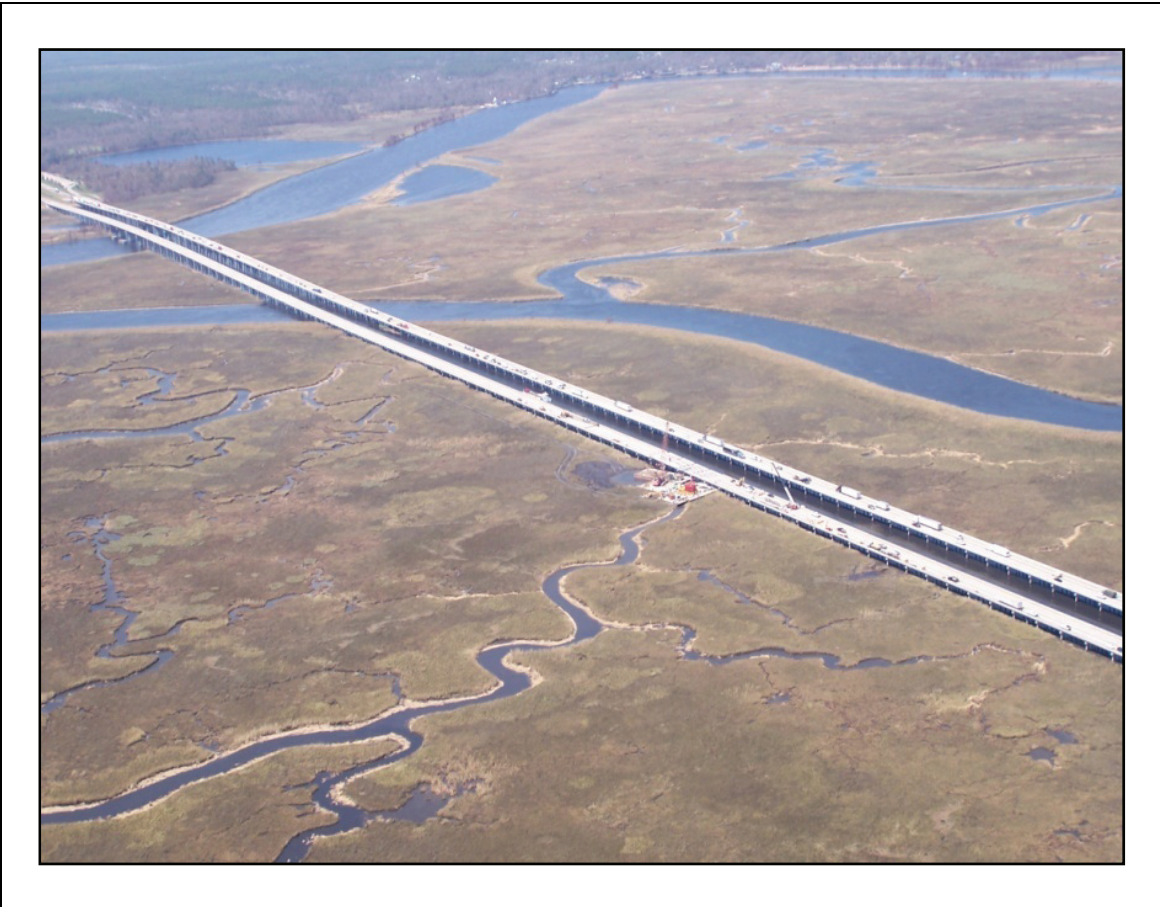
Figure 2-25. I-10 traverses a large salt bayou near Moss Point. It was hit and damaged by a stray barge.
