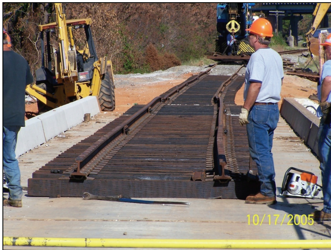
Figure 2-57. Modular sections of track were used to restore the line to service.
