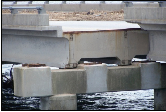
Figure 2-127. Lateral movement may have been restricted by the short pedestal (riser).
