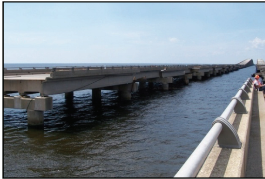
Figure 2-130. This view is looking SW from the deck of the WB bridge. Spans not dropped into the water completely were displaced to the south.
