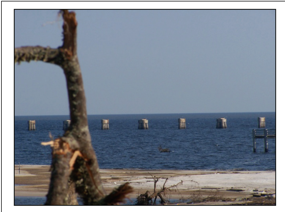
Figure 2-100. Piers from the CSX railroad bridge remain but the superstructure has been lost.
