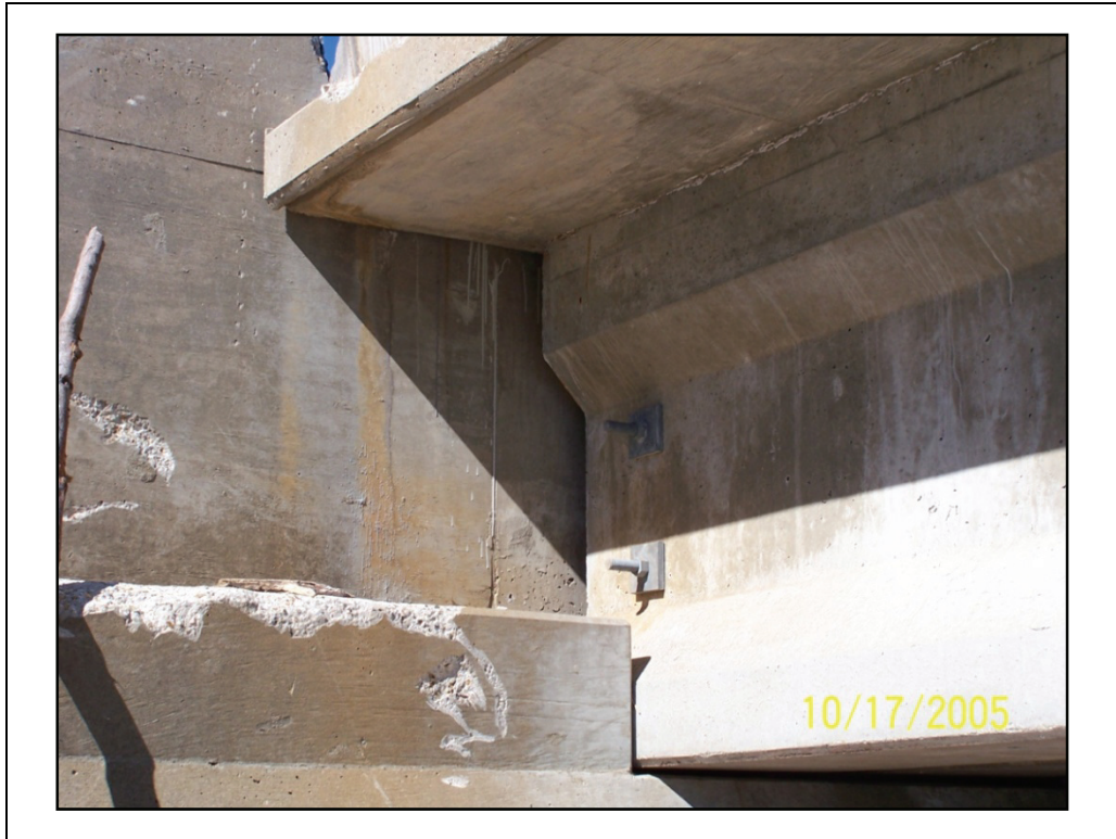
Figure 2-58. Lateral restraint blocks at the west abutment. Note the scars from debris.
