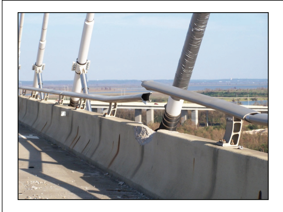
Figure 2-10. From the topside, damage to the railing and concrete barrier can be seen. A cable is wrapped to prevent moisture ingress, suggesting that it also was struck by the part of the oil platform. Note the silver damping devices on the other cables. These are commonly used on this type of structure to control wind vibration.
