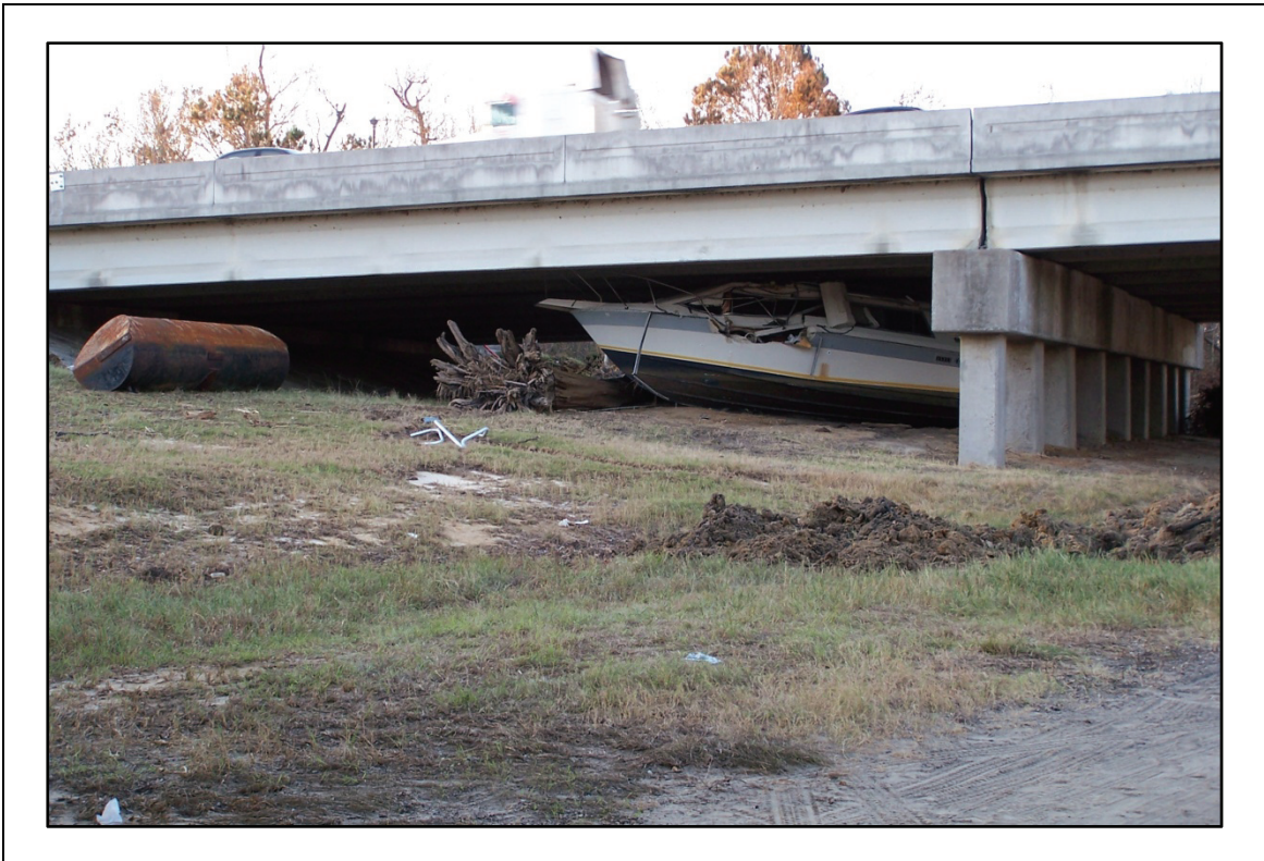
Figure 2-30. Large debris was lodged under the WB lanes of I-10 (a boat, tank, and a log).
