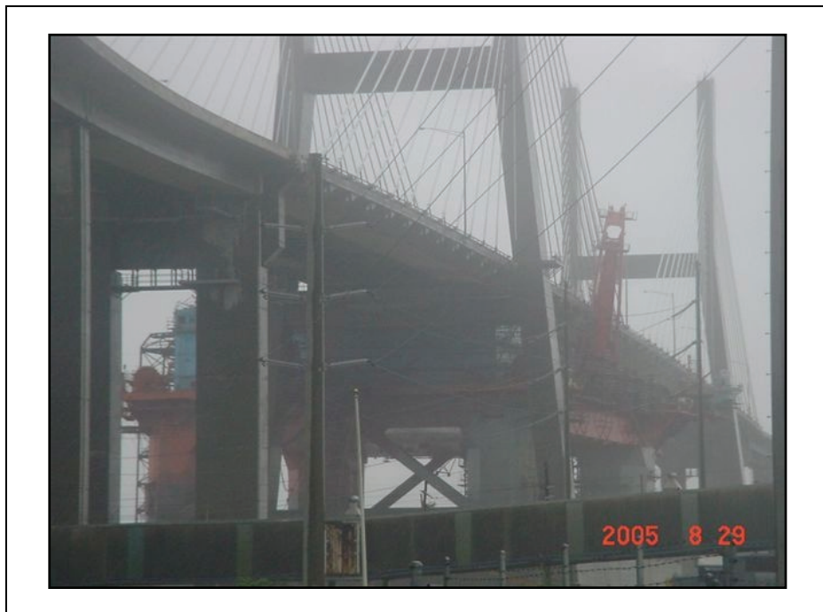
Figure 2-7. An oil platform lodged up against the Conchrane-Africatown USA Bridge.
