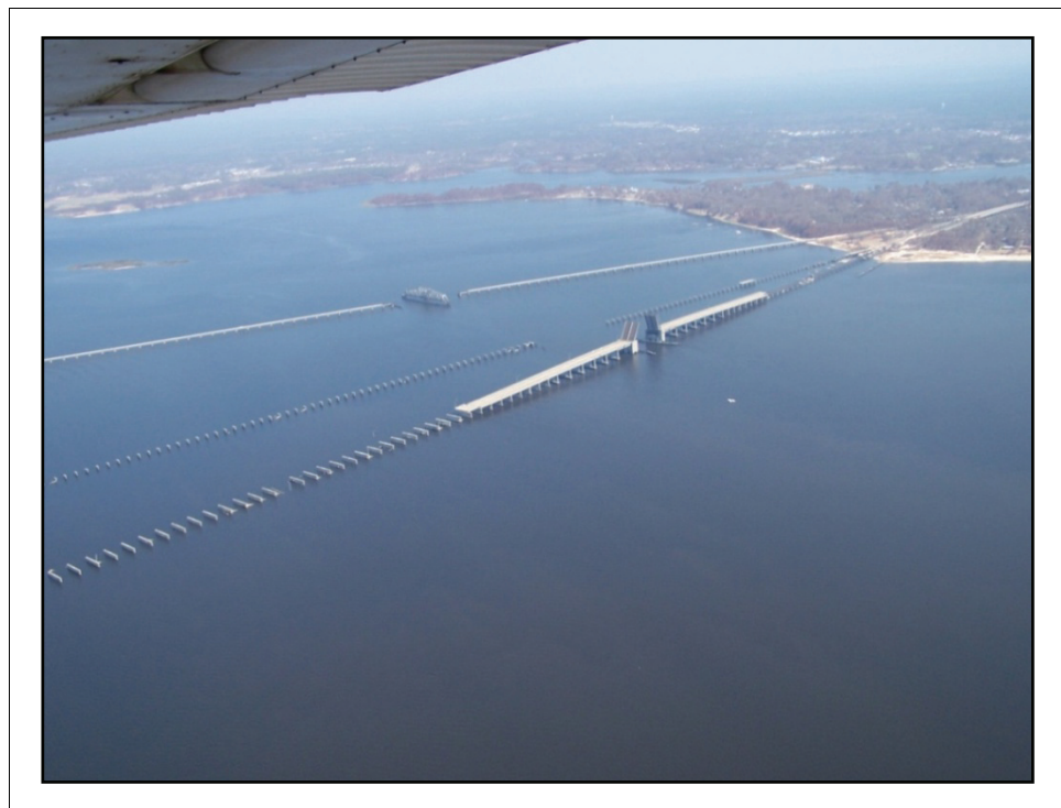
Figure 2-33. This Post-Katrina photograph (taken 9/11/05) shows the three bay crossings from Biloxi facing east toward Ocean Springs. Many spans are missing.
