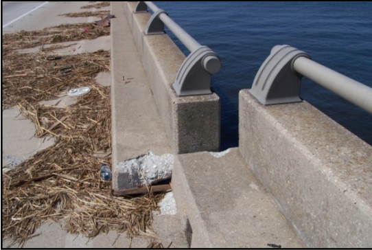
Figure 2-123. Relative displacement between spans.
