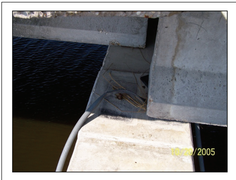
Figure 2-82. A look down at the top of a pier cap shows that the span on the left moved to the west by as much as four feet.
