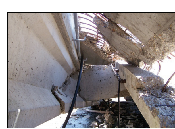
Figure 2-44. The beam, deck and diaphragm failed under surge loading.
