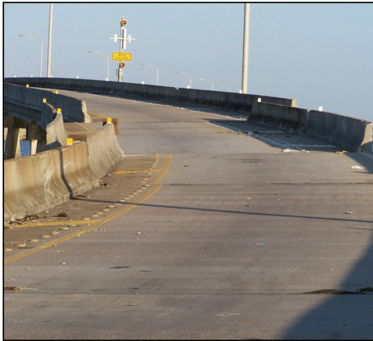
Figure 2-17. Looking east at the displaced spans.
