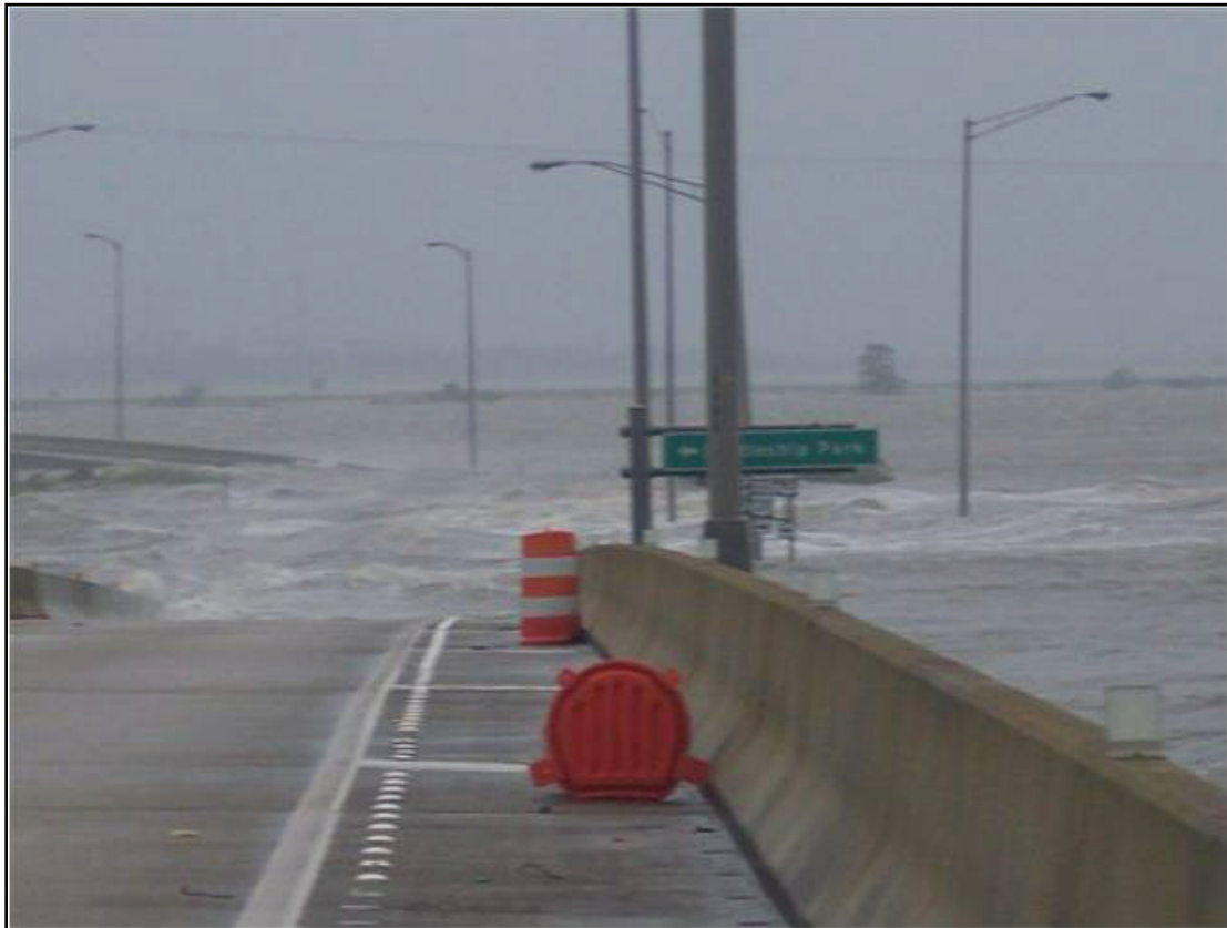
Figure 2-14. Several spans washed out the day of the storm. This photo faces east.
