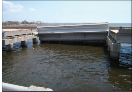
Figure 2-128. This EB span worked its way out laterally even as the adjacent spans stayed on the pier cap.
