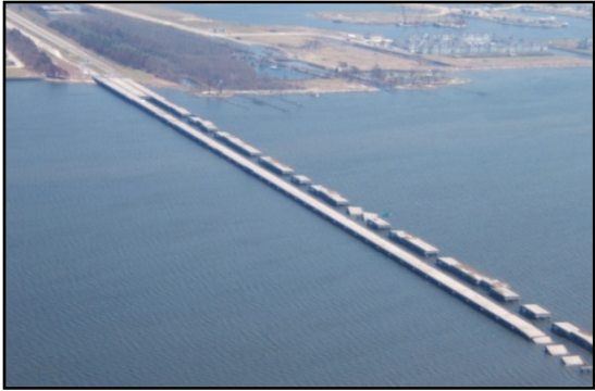
Figure 2-129. This view is looking SE so the EB bridge is on the far side. On this section of the bridge, the EB side lost many more spans.
