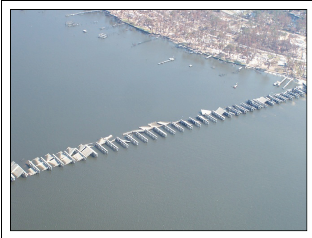
Figure 2-97. This photograph was taken facing NE at the east end of the US-90 bridge.
