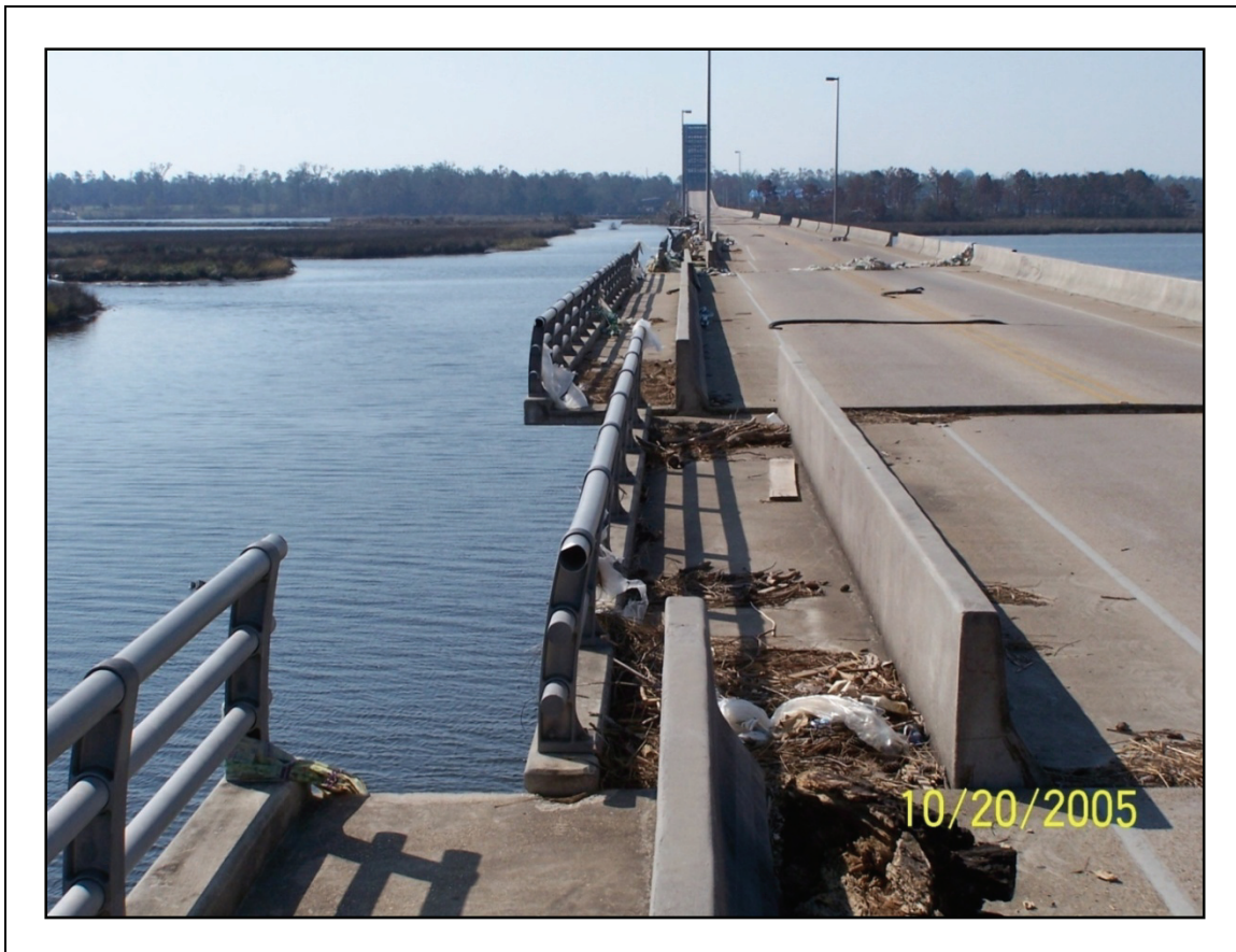
Figure 2-75. Numerous prefabricated spans were shifted to the west. None tipped over into the water. Note the black joint strip seal on top of the deck.
