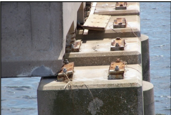
Figure 2-131. Seat length has been an important consideration in earthquake designs.
