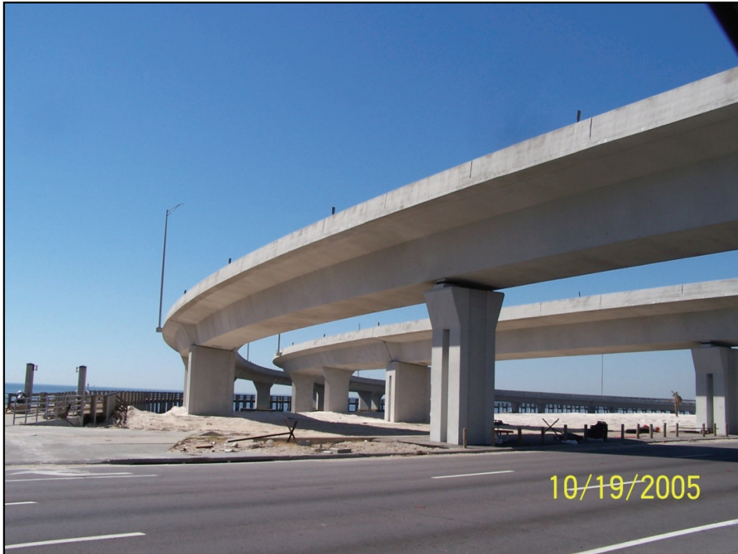
Figure 2-83. Southern terminus of I-110, with the Gulf in the background.
