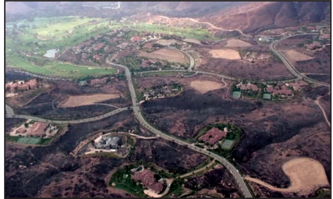
Figure 8. Good vegetation clearance practices helped to avoid house destruction.
