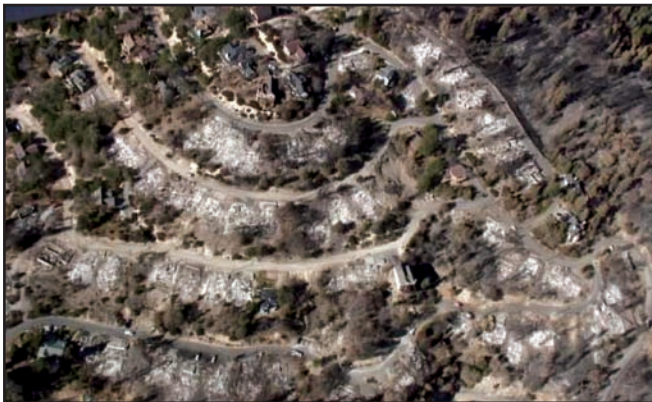
Figure 23. Destruction of houses in the Grass Valley area.
