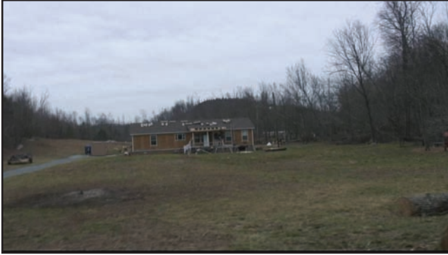
Figure 19. An example of minor roof damage in Hickman County. The degree of damage is somewhat uncertain in this case because construction efforts were already started.
