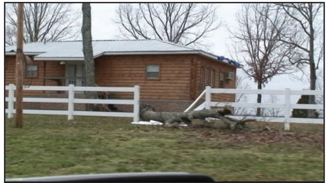
Figure 16. A log home with minor roof damage in Hickman County.
