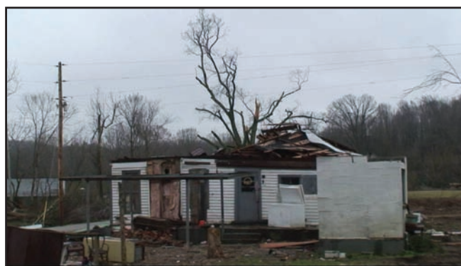
Figure 14. An example of likely substandard construction with higher degree of damage than surrounding structures in Faxton, TN (Benton County).
