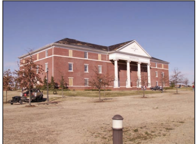
Figure 22. Minor damage to windows and roof shingles at Jennings academic hall. Residence halls in previous pictures are in the background.
