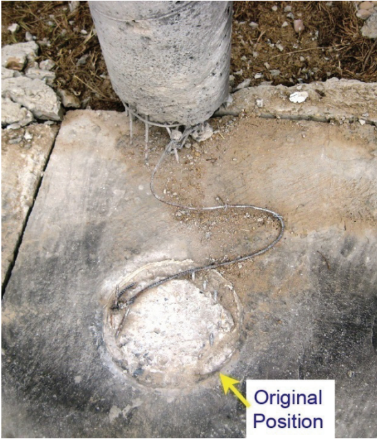
Figure 3-32 Column RC1 at Bottom (Test 1)
