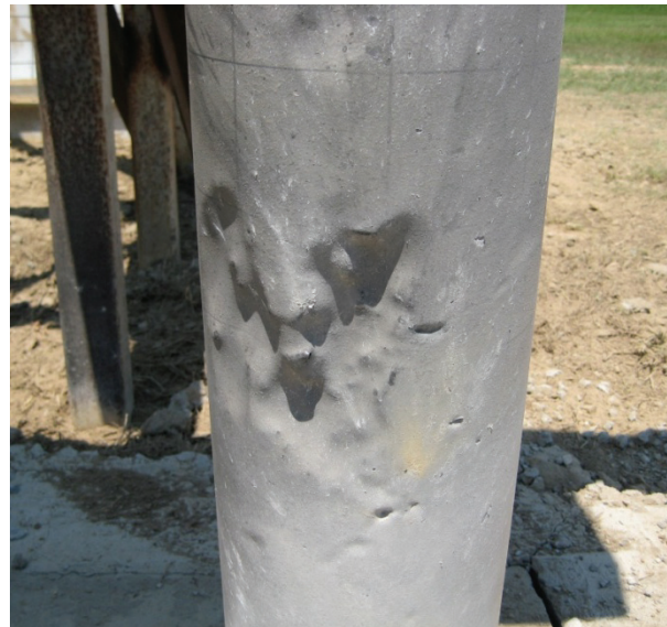
Figure 3-56 Void at Column SJ2 after Test 3
