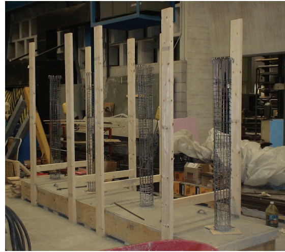
(b) Column Reinforcement after casting footing concrete
