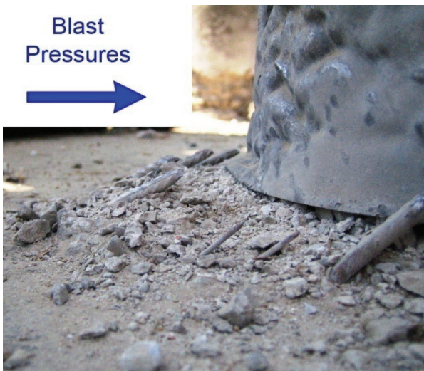
Figure 3-59 Fractures of Longitudinal Bars Column SJ2 at Bottom (Diagonally Front View, Test 3)
