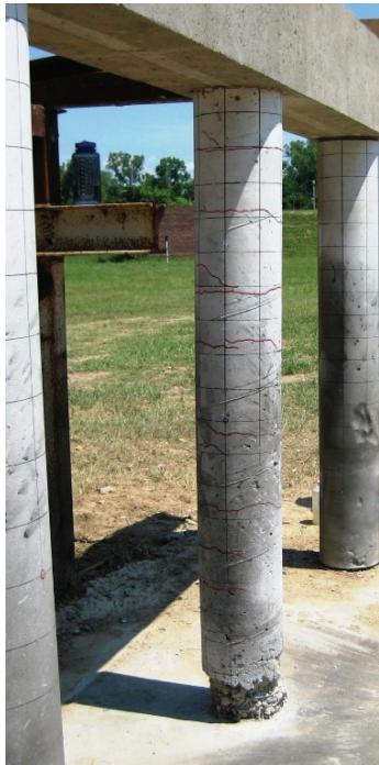
Figure 3-44 Front Diagonal View of Column RC2 (Test 2)
