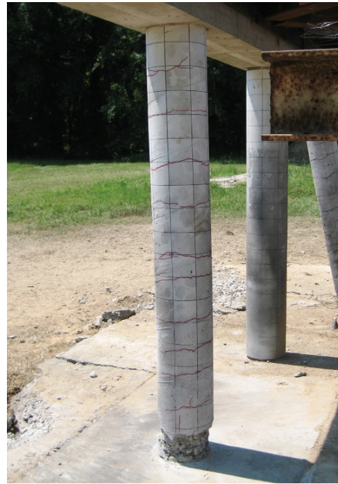
Figure 3-45 Back Diagonal View of Column RC2 (Test 2)
