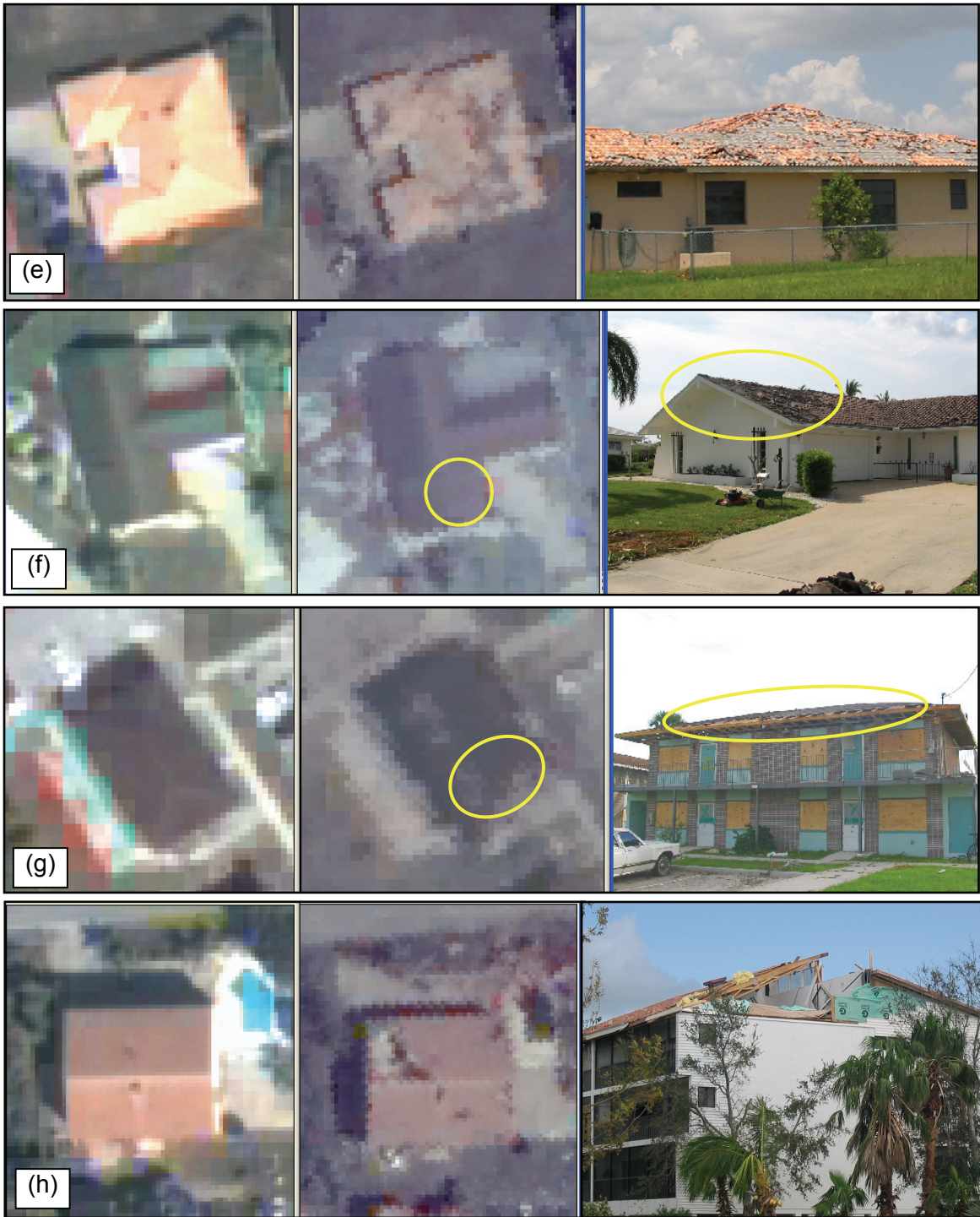
Figure 3-8 (continued) Examples of Windstorm Damage to Residential Buildings: Pre- and Post-Storm Quickbird Satellite Images and Ground-Truthing Photos. Credit: DigitalGlobe, Inc. < www.digitalglobe.com >.
