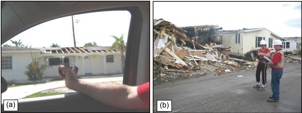
Figure 2-5 Deployment of the VIEWS™ Field Reconnaissance System in Hurricane Charley for Field Data Collection (a) from Moving Vehicle and (b) on Foot
