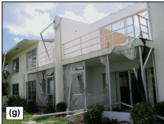
Figure 2-7 (continued). Comparison of Pre- and Post Storm Building Conditions in Satellite Images, Along with Ground-Survey Photos. Ground-Survey Photos Demonstrate: (c) Partial Roof Deck Failure (Combined Internal And External Pressures); (d) Shingles Partially Removed but Deck Intact; (e) Scoured Roof Gravel (Not Visible from Ground Survey); (f) Partial Roof Structure Failure; (g) Severe Roof Structure Failure; (h) Windborne Debris from Nearby Building Deposited on a Parking Lot, Roadway, and Tennis Court. From Womble (2005).
