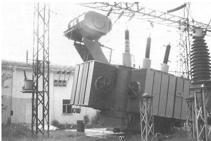
Figure 1-6 Damage to a Transformer Foundation [EERI, 1999]
