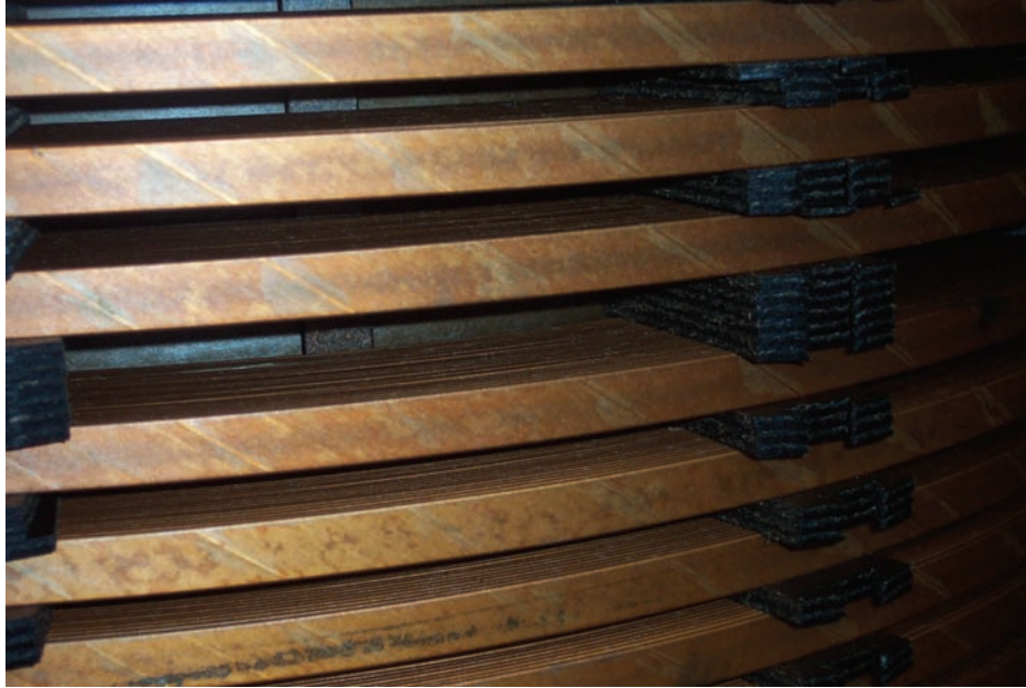
Figure 7-16 Key Spacers Separating Different Layers of Winding.
