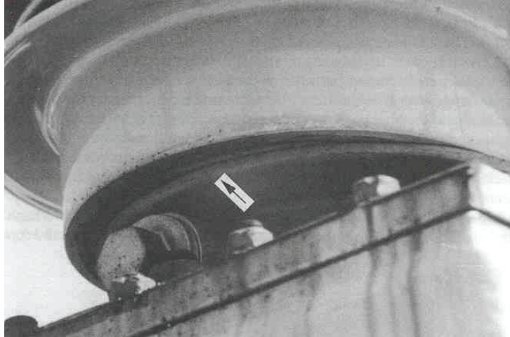
Figure 1-7 Bushing Failure at the Flange [ASCE, 1999]
