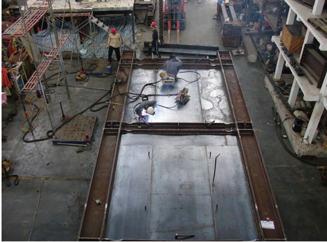
FIGURE 3-12 Welding Infill Panels to Boundary Frame (Photo Courtesy of C.H.Lin and K.C.Tsai, NCREC)
