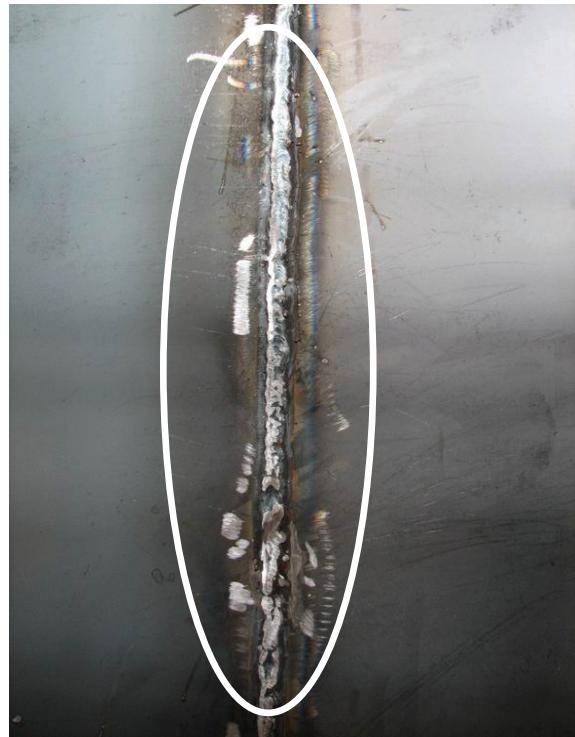
(b) Final Continuous Welds
