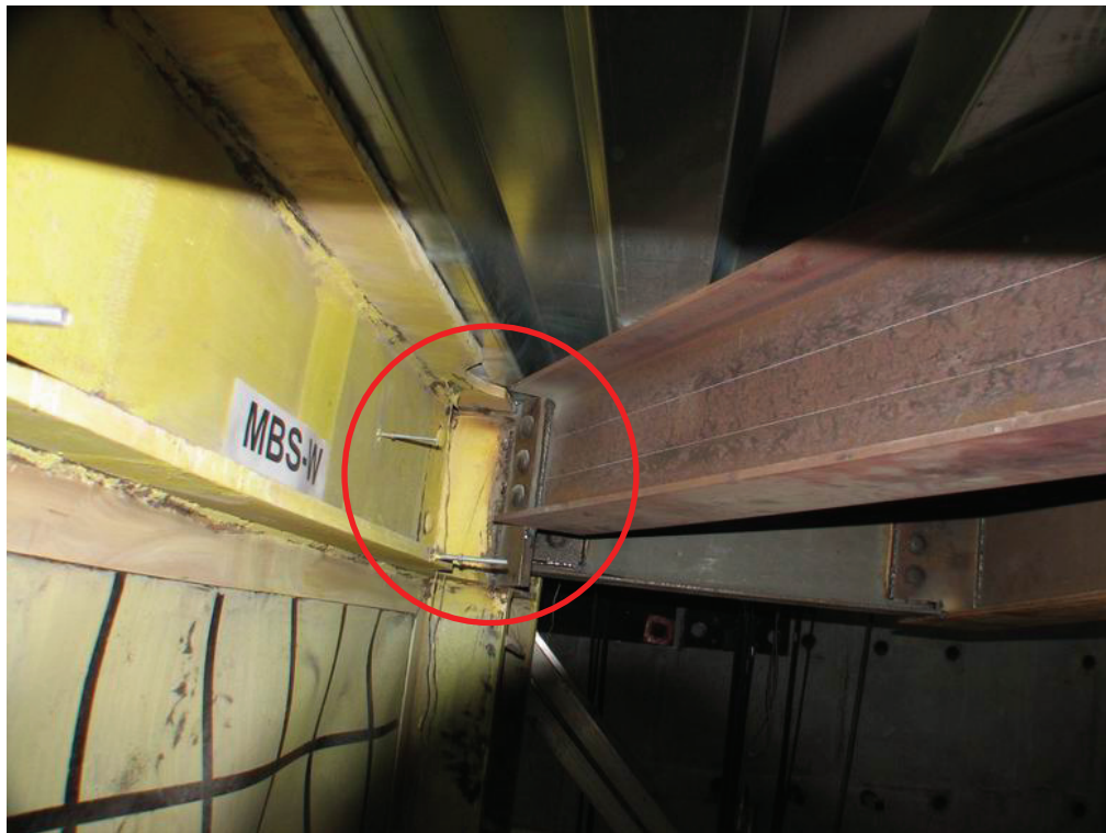
FIGURE 4-12 Typical Floor-Truss-Member-to-Intermediate-HBE Connection
