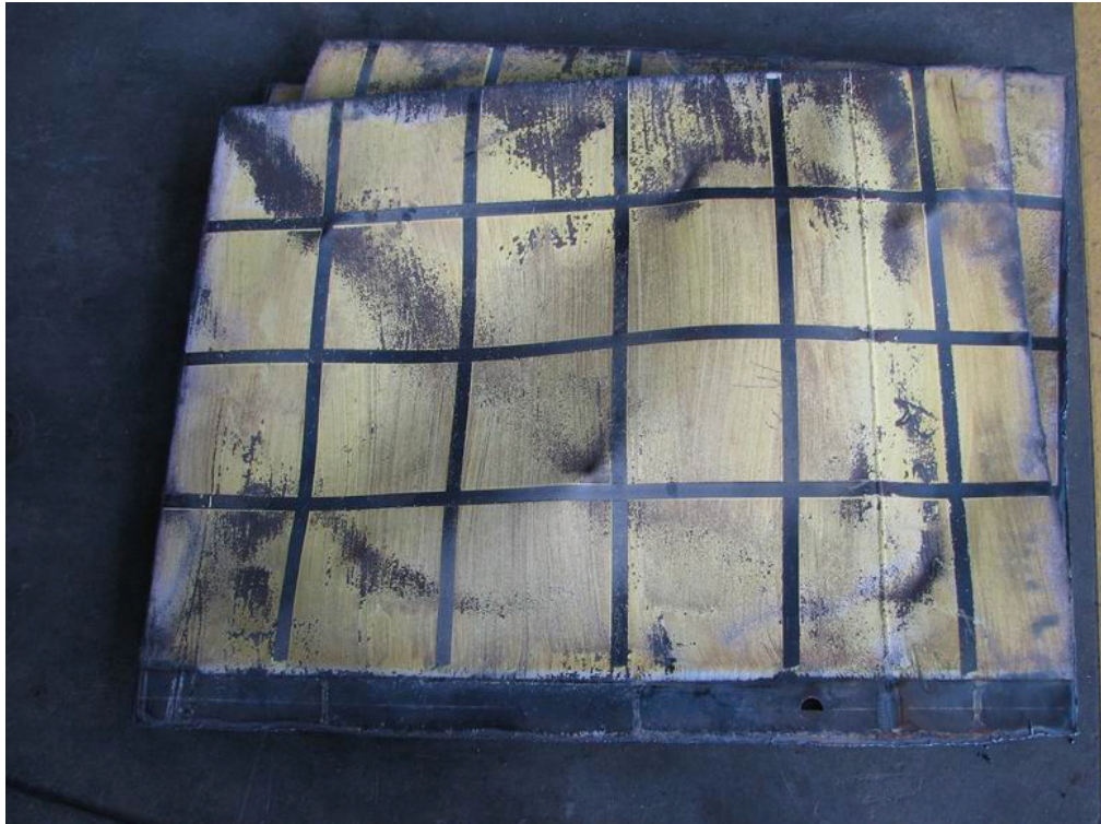
FIGURE 4-27 Cutout Buckled Panels
