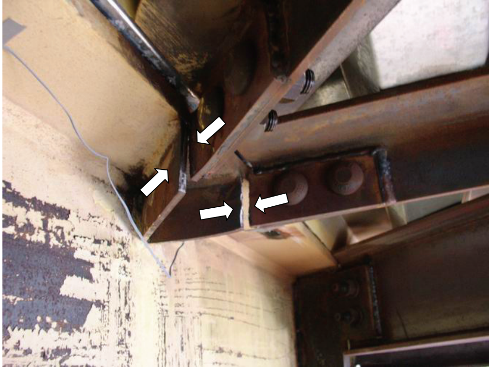
(a) Fractures of the Truss Members Connected to the Middle of the Top HBE
