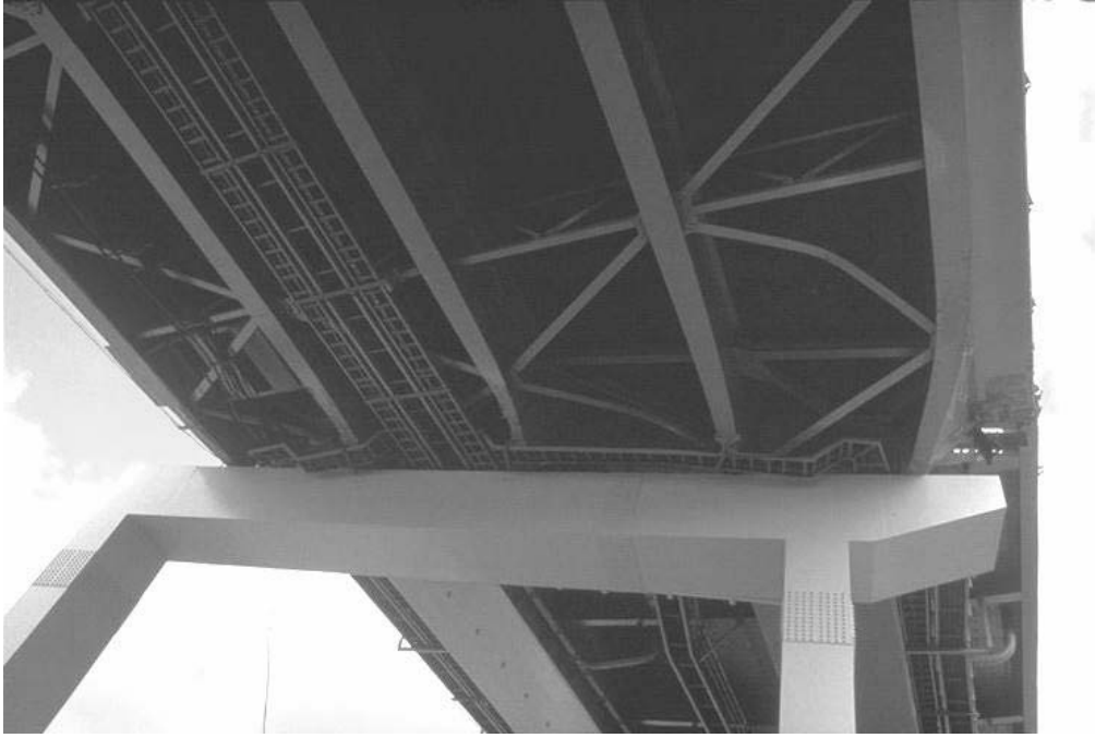
FIGURE 1-5 Damage to girders and bracing of Hanshin Expressway during 1995 Hyogen-Nanbu (Kobe) earthquake
