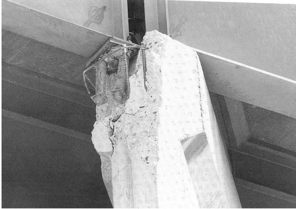
FIGURE 1-1 Damage to bearing assembly of Santa-Clara River bridge during 1994 Northridge earthquake (Astaneh-Asl, 1994)
