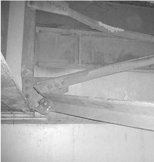
FIGURE 1-6 Fractured lateral bracing and buckled cross frame in Capitol Arch bridge during 2001 Nisqually earthquake (WSDOT, 2001)
