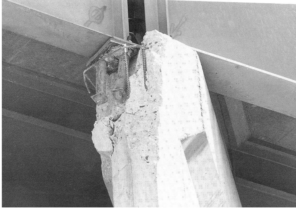
FIGURE 1-2 Damage to bearing assembly of Santa-Clara River bridge during 1994 Northridge earthquake (Astaneh-Asl, 1994)
