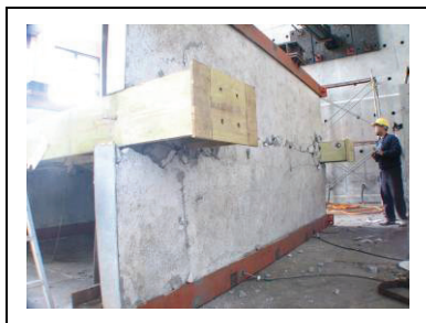
Figure 6. Crack at the top slab
