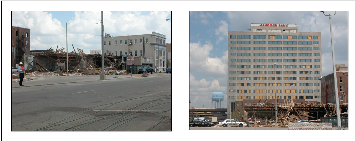
Figure 4-1. Left: partial collapse of unreinforced masonry bearing-wall building, downtown Gulfport MS. Debris from this building may have impacted a high-rise building downwind, causing extensive wind damage (right).
