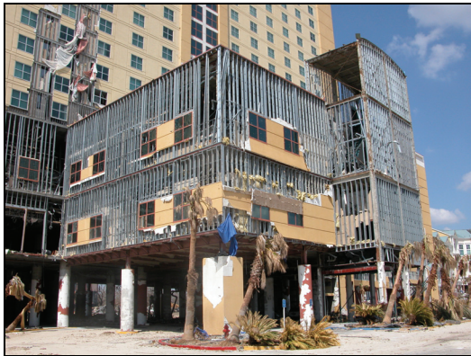
(a) Exterior Damage
