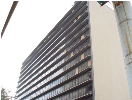
(a) Boarded Windows
