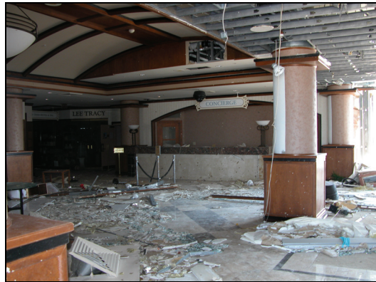
(b) Interior Damage
