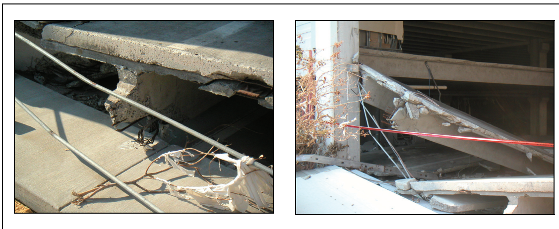
Figure 4-11. Shear failure in deck-beam shear keys.
