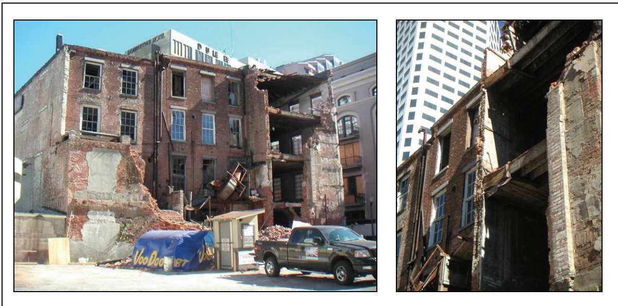
Figure 4-2. Partial collapse of New Orleans unreinforced masonry bearing wall building.
