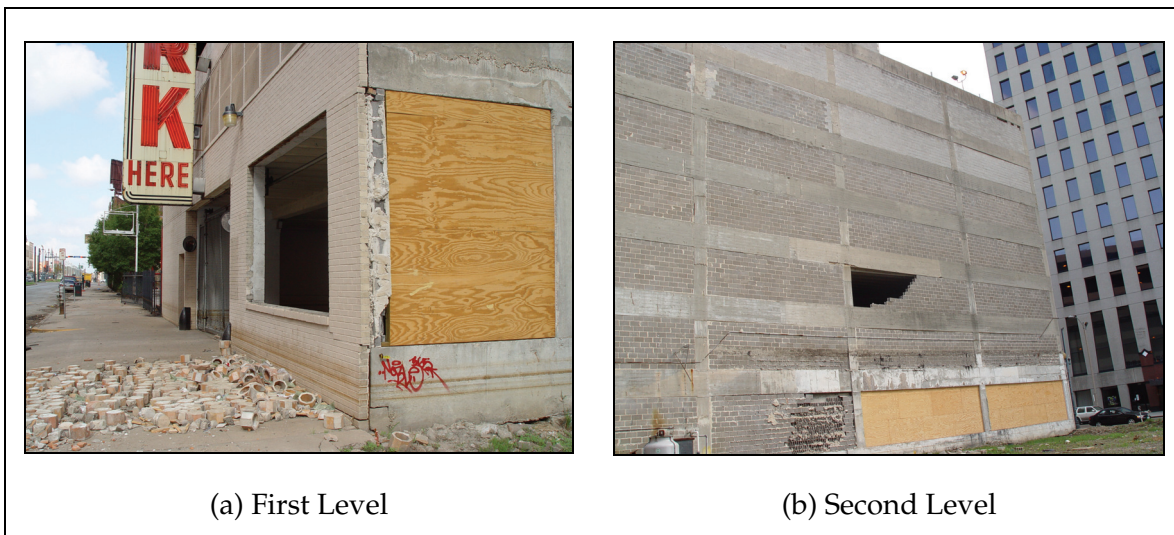
Figure 4-4. Masonry infill damage.
