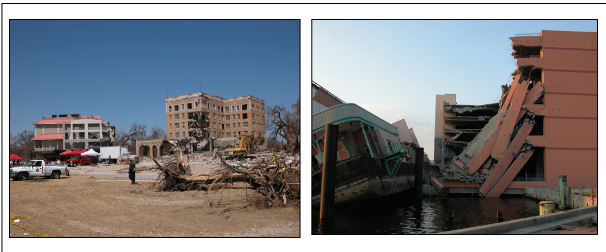
Figure 4-5. Structural damage resulting from surge-borne debris.
