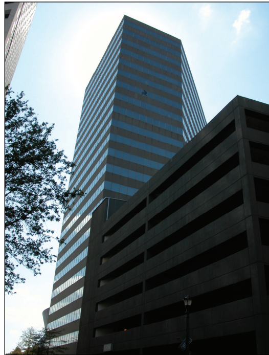
(b) North Facade
