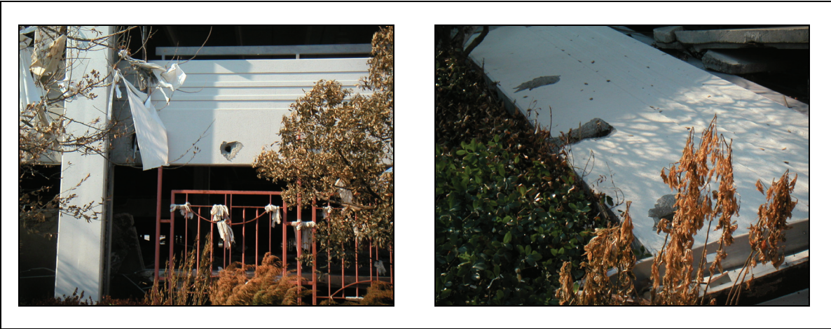
Figure 4-6. Evidence of horizontal pounding by waves. Deck-beam shear key appears to have punched holes in the spandrel beam.
