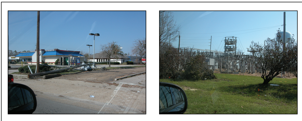
Figure 5-1. Downed power pole with poletop transformer; exposed substation equipment in Biloxi, MS, replaced by October 7.
