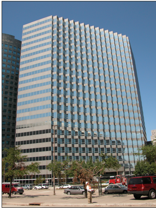
(a) South Facade
