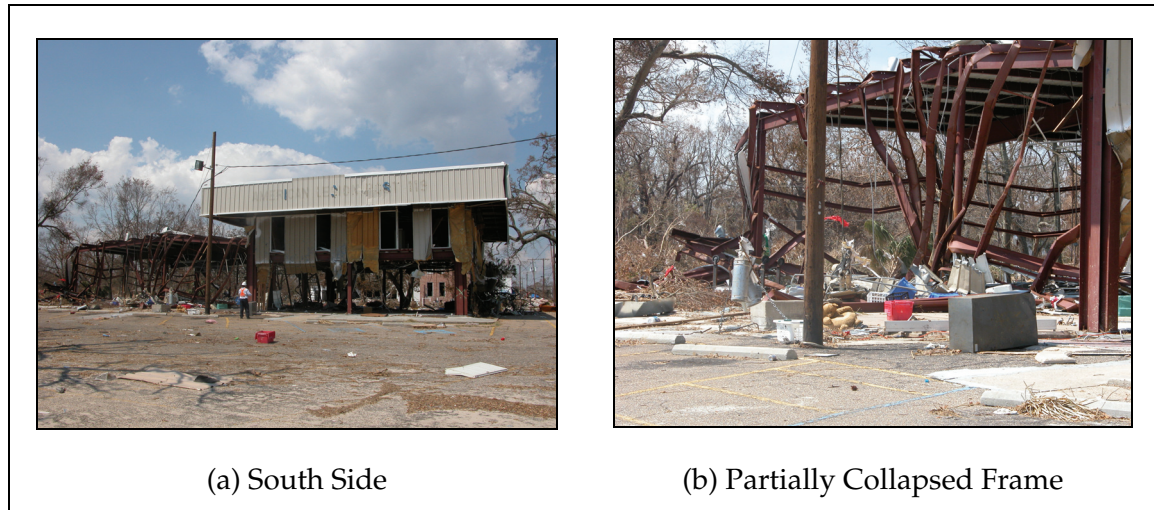
Figure 3-17. Damage to steel building in Gulfport coast.
