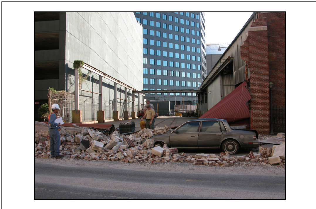
Figure 4-3. Collapsed unreinforced masonry wall.
