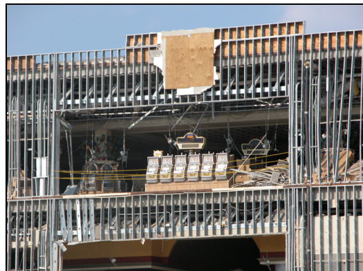
(b) Damage to Barge
