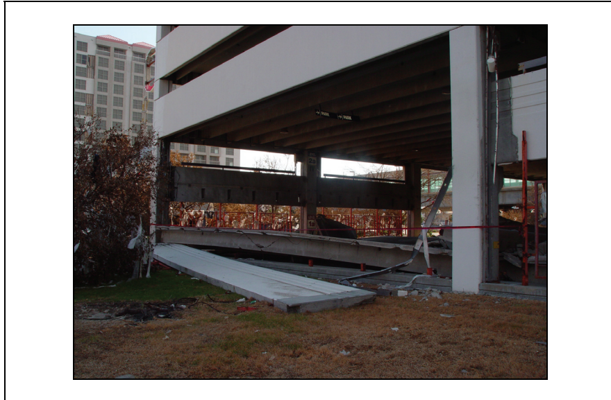
Figure 4-10. Flexibility of spandrel beams.
