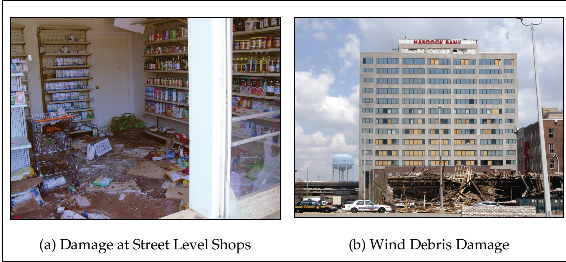
Figure 3-14. Flooding and wind damage in downtown Gulfport.
