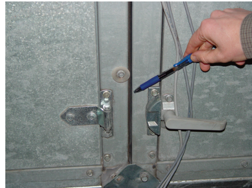
(b) Separation of Modules Resulting from Damage to Connection Plates between Base Rail and Test Specimen Housing
