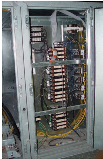
(c) Electric Heat Coil Module
