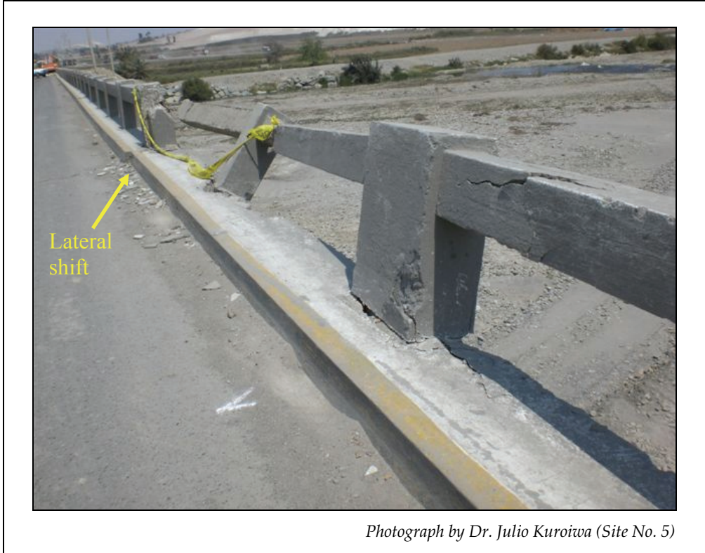
Figure 5-23. Broken railing and shift in curbside resulting from lateral movement of the span. Corrosion probably played a role in failure of the barrier.
