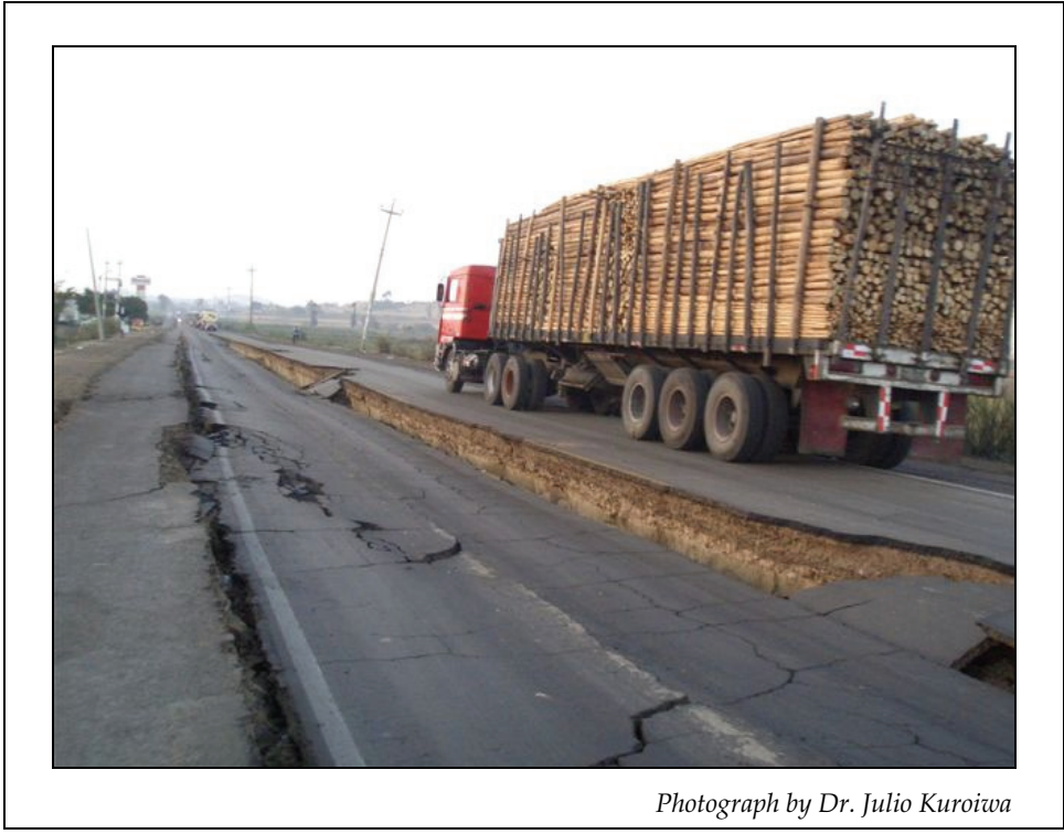
Figure 5-14. Pan-American Highway near San Clemente Approximately km 220.
