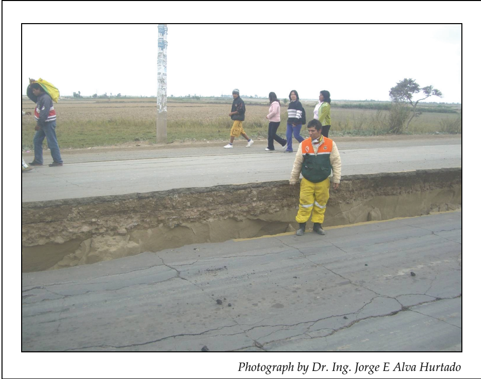
Figure 5-13. Pan-American Highway Near San Clemente Approximately km 220.
