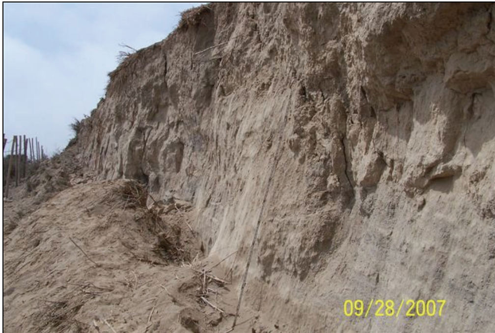
a. Three meter (10') escarpment remaining at Sunampe after coastal shelf slid toward the ocean
