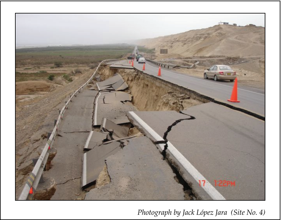
Figure 5-6. Embankment and roadway failure at km 190. The picture was taken facing north. Note the Pacific Ocean in the top left of the photo. The damage was caused by amplification of the ground shaking. Liquefaction of the wet coastal silts and sands led to lateral spreading and the embankment failure.
