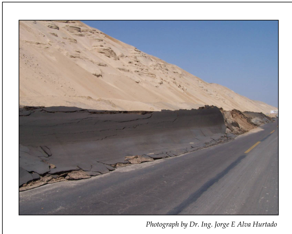
Figure 5-2. East shoulder of Pan-American Highway at km 178 pushed up onto sand dune after lateral displacement of roadway during liquefaction and “sloshing” of supporting ground.
