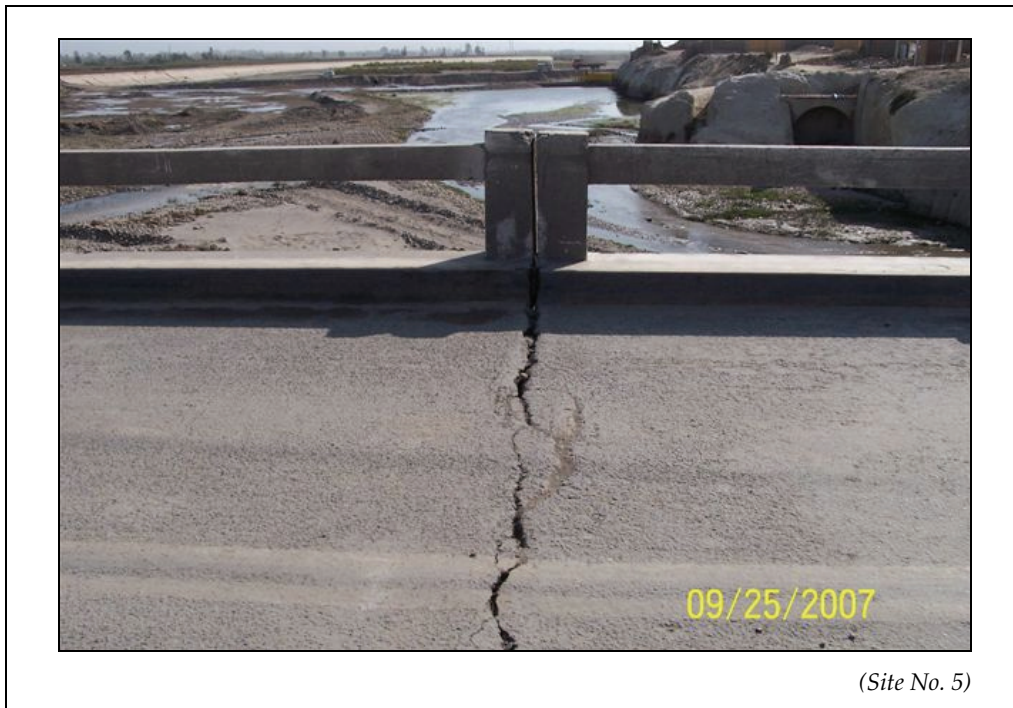
Figure 5-22. Cracked deck due to horizontal movement of the span.
