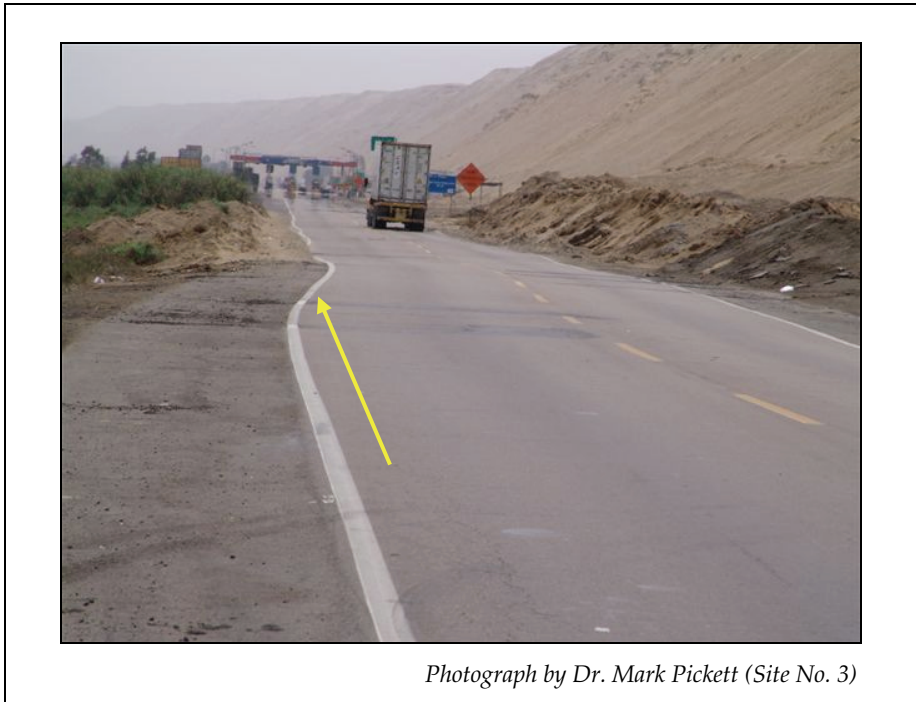
Figure 5-4. Note the white edge line. This is evidence of lateral displacement of the roadway at km 188 due to liquefaction at the toe of slope and reflection of seismic ground waves against the more rigid sand dune on the east side of the highway.
