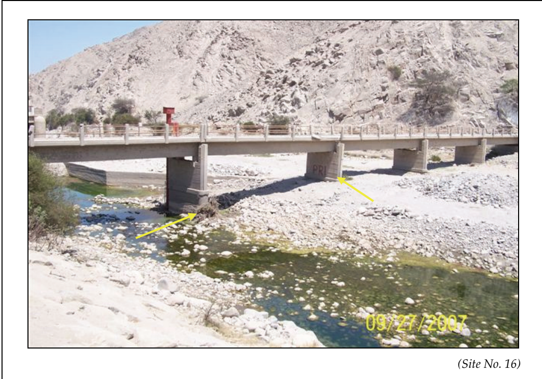
Figure 5-39. Puente Los Molinos. Note the pre-existing scour (>2m or 6') at Pier No. 1 (as identified from left to right) (see arrow) and tipped Pier No. 2 shown with the arrow on the right.
