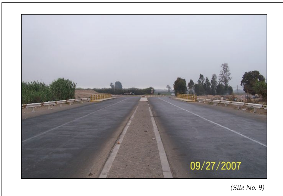
Figure 5-50. Concrete bridge near the epicenter that performed well.
