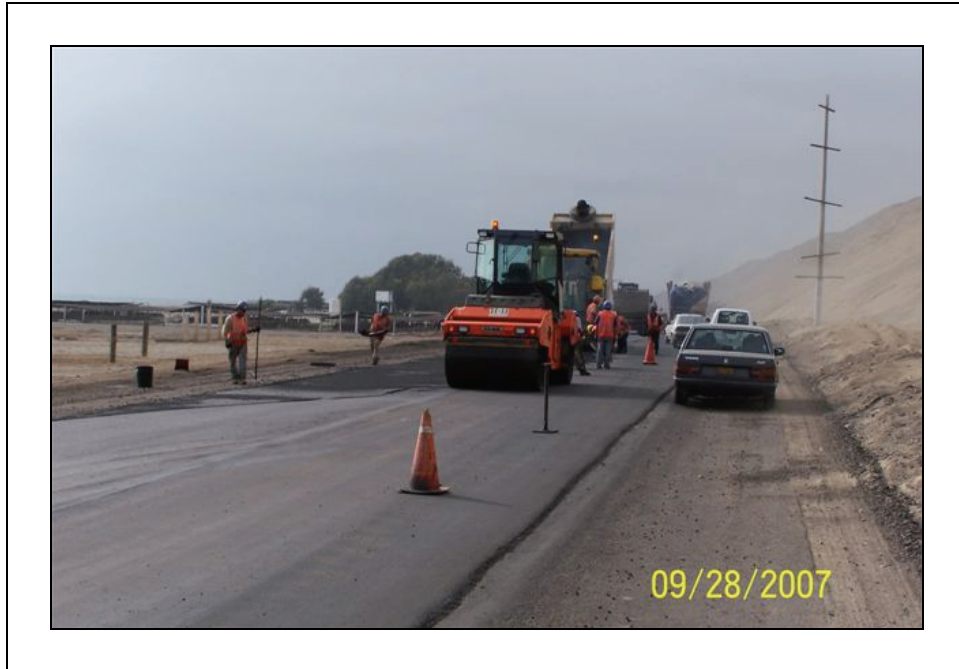
Figure 5-15. This is one of the many sections of the Pan-American Highway that needed pavement repairs after the earthquake. Paving was still going on six weeks after the event.
