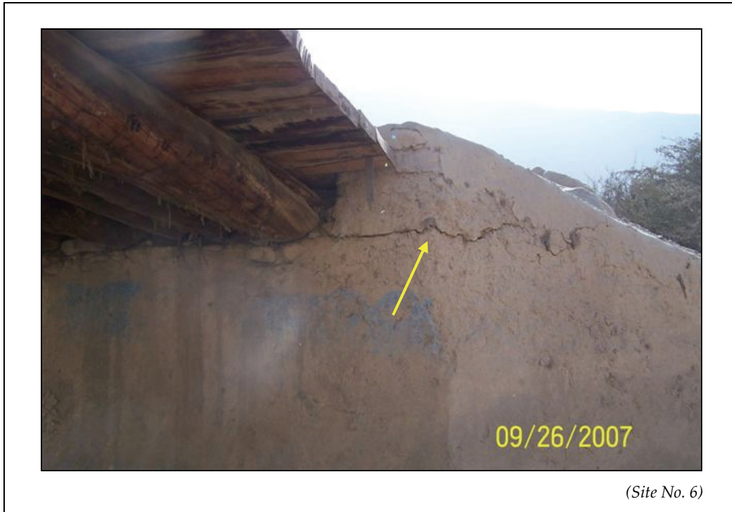
Figure 5-33. Slight cracking may have been from horizontal loads imposed by the superstructure.
