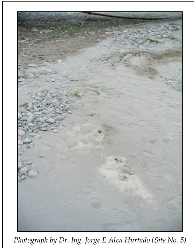
Figure 5-19. Sand boils in the stream bed at the Huamani Bridge indicate that the soil liquefied.
