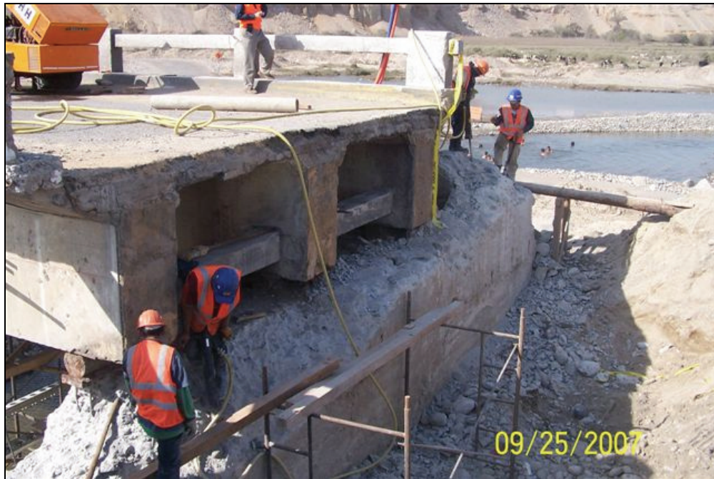
b. Ongoing reconstruction of South Abutment
