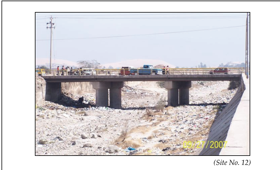
Figure 5-51. Concrete bridges like the Puente Socorro within the City of Ica performed well.
