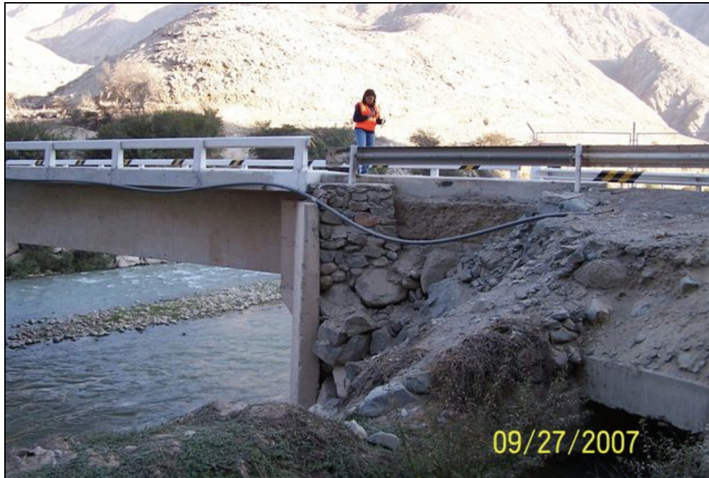
a. Loss of rock wingwall and backfill at the left side of the abutment, possibly aggravated by the earthquake
