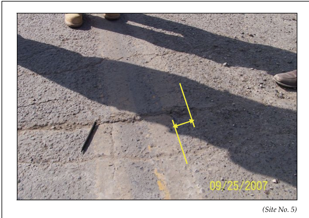
Figure 5-21. Horizontal displacement of the superstructure is evident by the shift in the centerline at a joint
