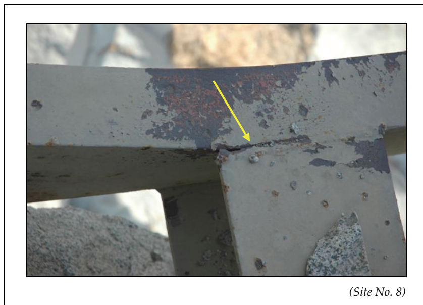
Figure 5-38. Cracked weld along bottom chord resulting from distortion of the channel after impact from debris. There is potential for this type of crack to propagate into the primary member and cause sudden failure.
