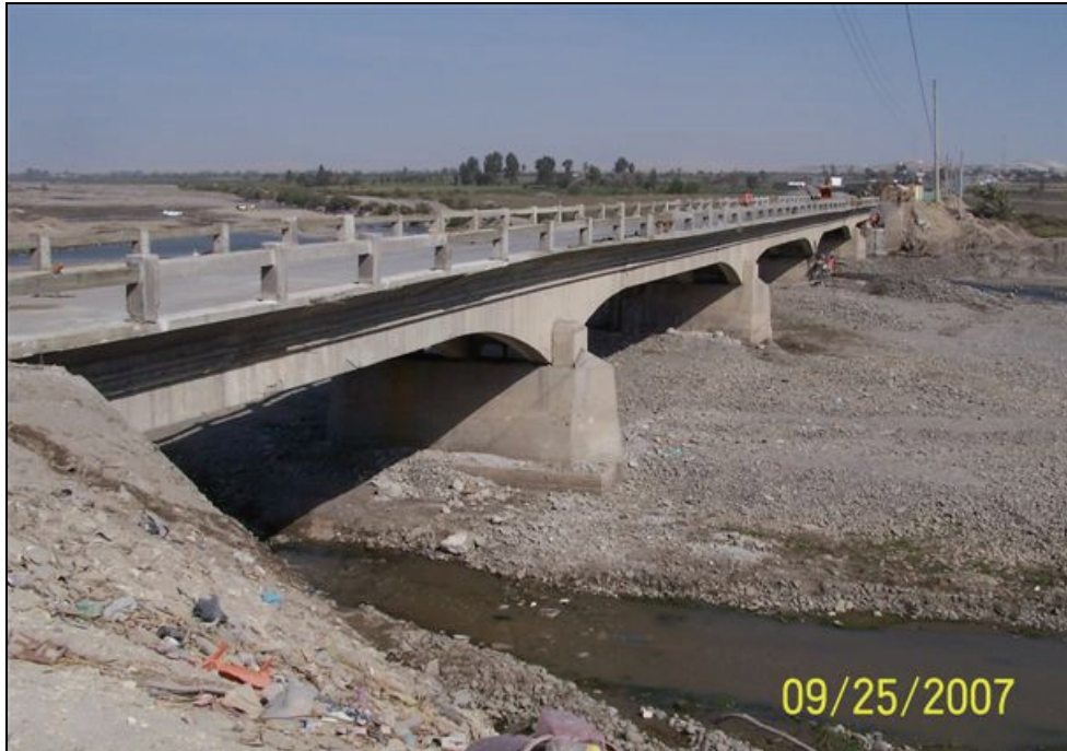
a. This bridge was still closed for repair five weeks after the earthquake
