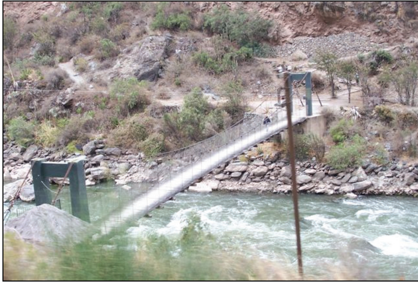
Figure 5-58. In the mountainous Andean highlands, several pedestrian suspension bridges survived the earthquake without damage.
