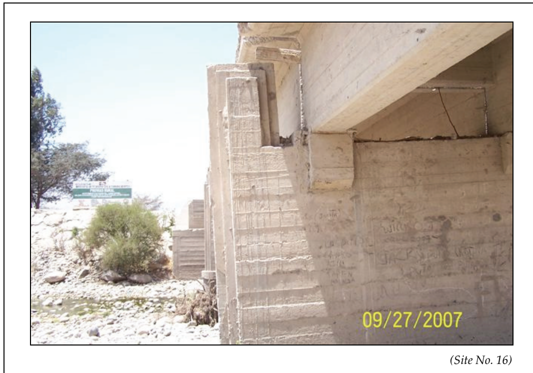
Figure 5-40. Tipped pier resulting from El Niño flooding of 1998.
