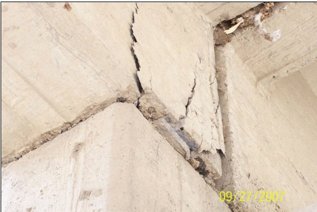
b. Another serious shear crack probably caused by earthquake-induced lateral motion
