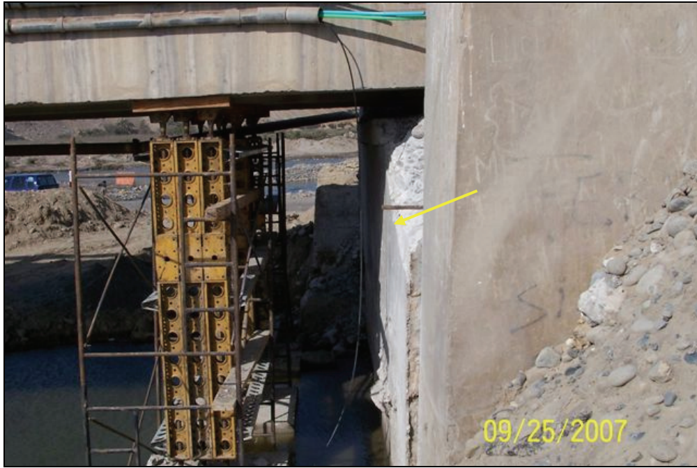
a. South end of span is supported while tipped abutment is replaced
