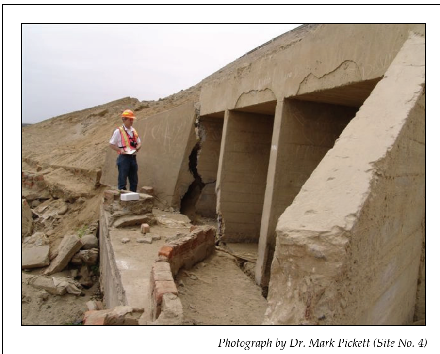
Figure 5-8. Outlet end of failed box culvert at km 190.
