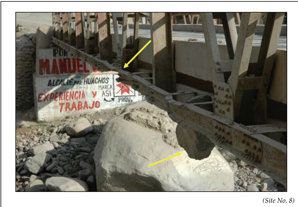
Figure 5-36. Puente Huachinga at km 39. This steel truss bridge has suffered severe damage to the bottom chord from presumably previous debris impact (top arrow). There is a large granite boulder jammed between the two channels of the bottom chord that has fallen from the adjacent mountain from this earthquake (bottom arrow).
