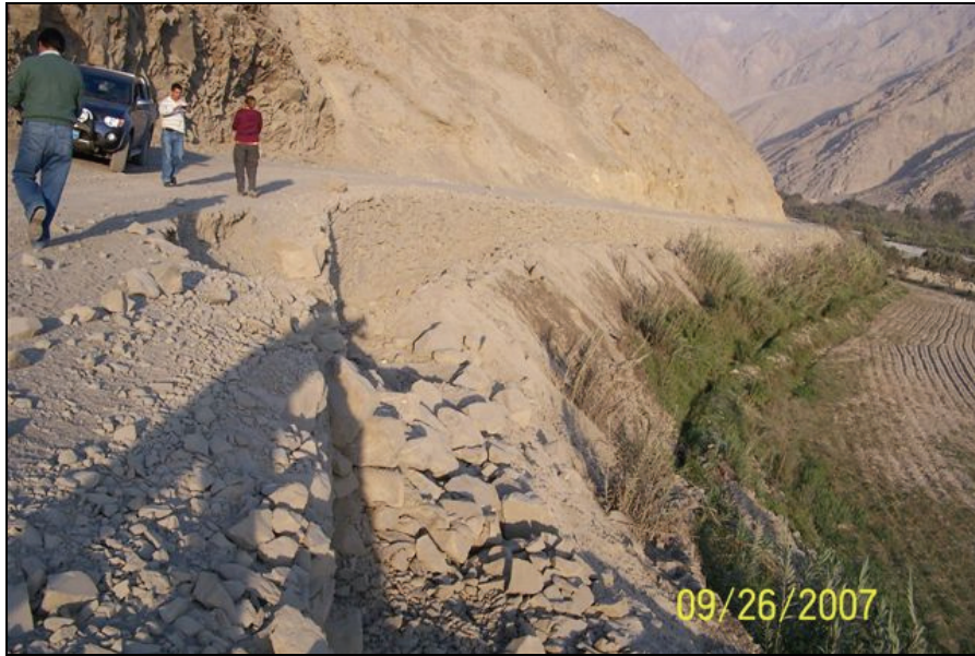
a. Failed retaining wall
