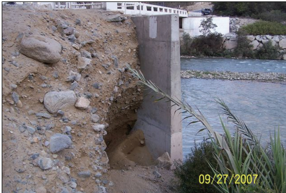
b. Erosion at the right side of the same abutment. Round rocks in the gravel make the site more susceptible to loss of material
