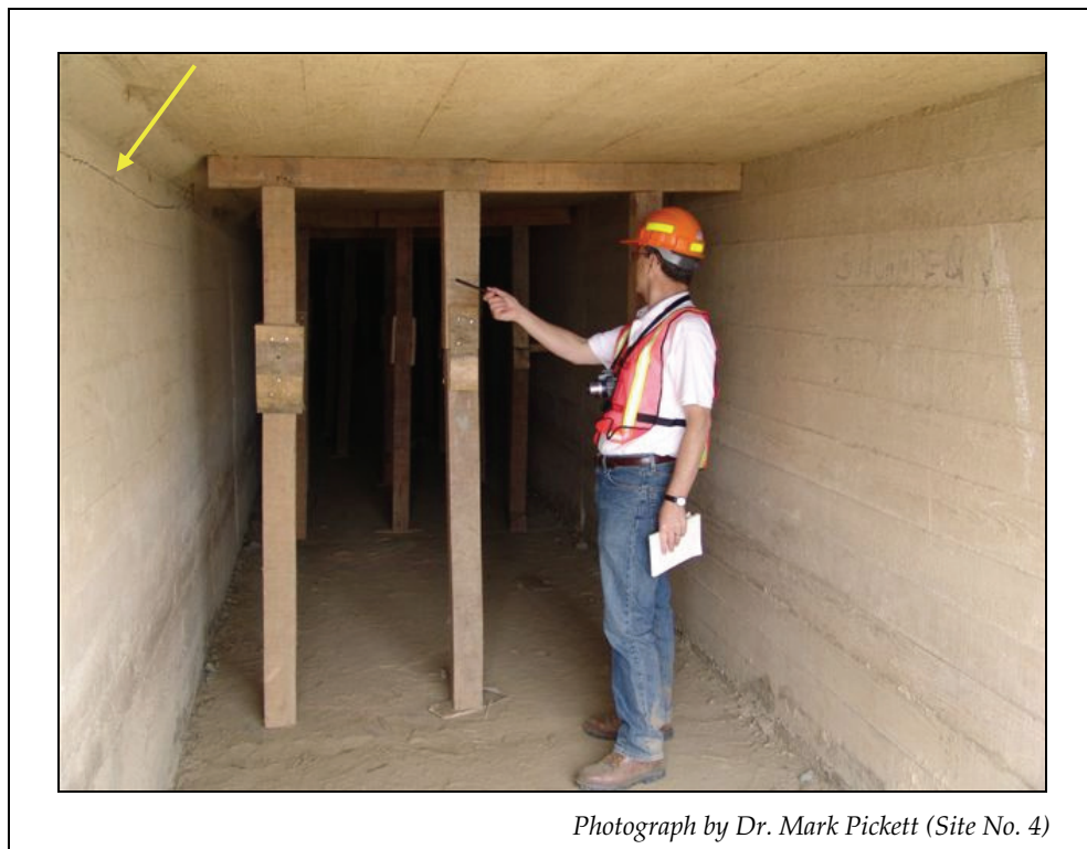
Figure 5-10. Timber shoring and a horizontal crack in a concrete box culvert km 190.
