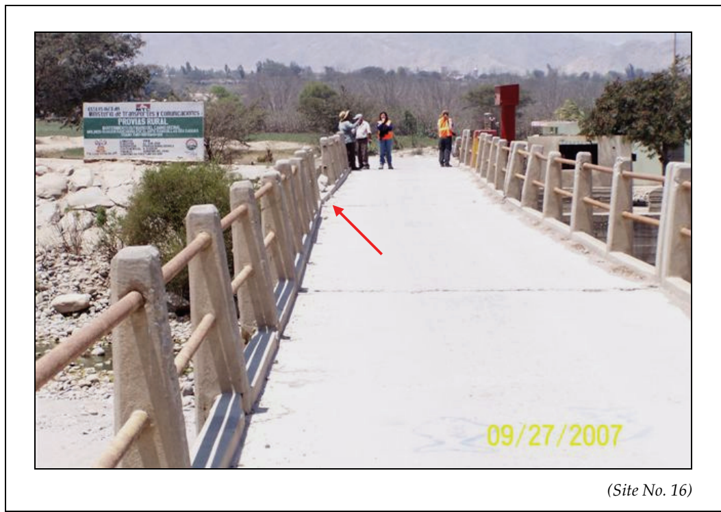
Figure 5-45. Lateral shift of the superstructure.
