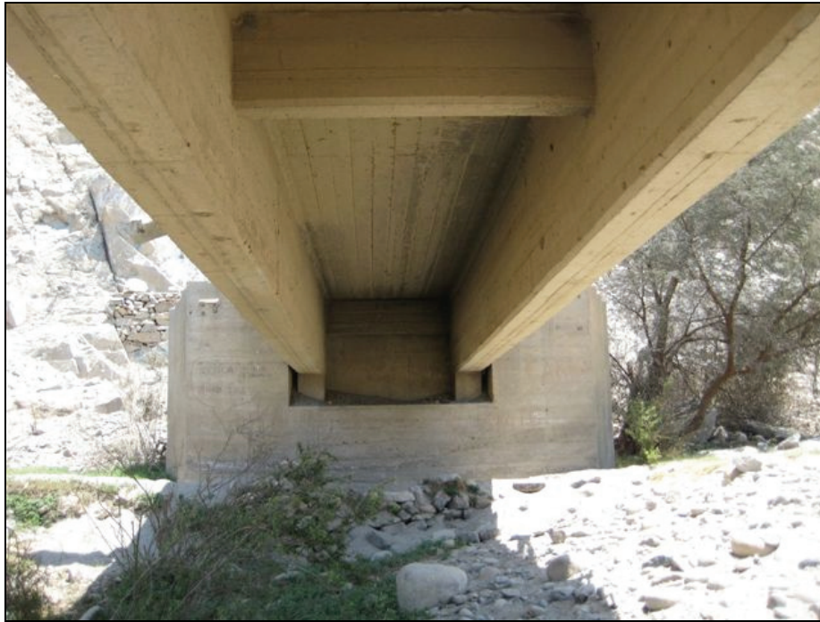
Photograph by Lucero Mesa (Site No. 16)
