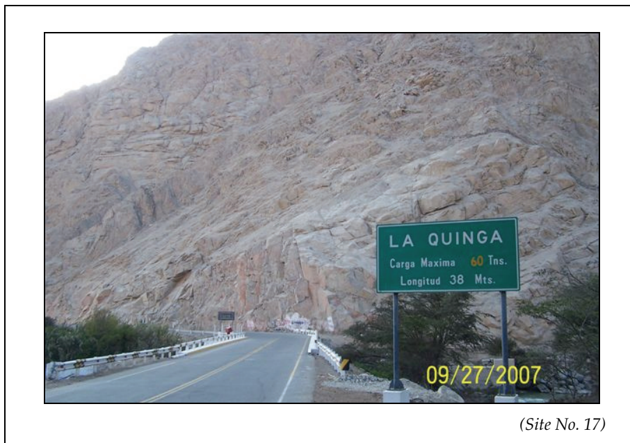
Figure 5-47. The rocky terrain above Puente Quinga presents a danger of impact from boulders. The bridge showed evidence of slight lateral motion that resulted in minor cracking of the approach curbing.
