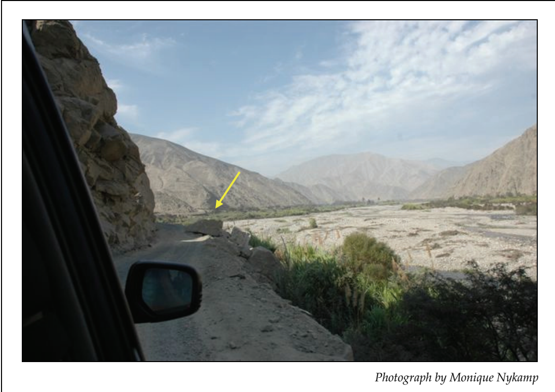
Figure 5-28. Typical terrain along Departmental Route 100. The road tracks the mountain on the left and is subject to rockfalls as is seen in this photo.
