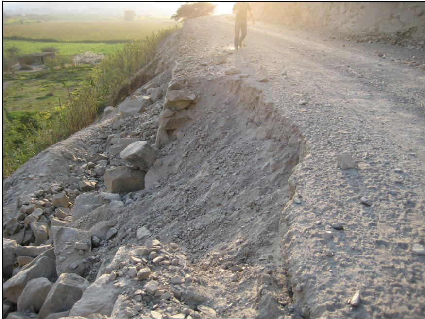
b. Road damage from failed retaining wall
