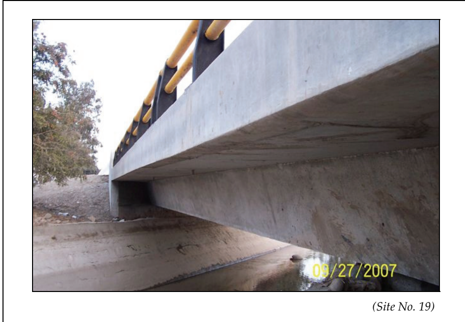
Figure 5-49. This example of newer bridge construction performed well.
