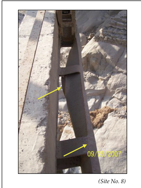
Figure 5-37. Puente Huachinga at km 39. It is uncertain whether this bottom chord damage was caused by falling boulders from this event or whether it remains from a previous hazard, such as El Niño effect flooding that last occurred in 1998. This deformation can limit the capacity of this tension member and put additional stress in the undamaged channel. Figure 5-38 shows a close-up of the crack that the lower arrow is pointing to.
