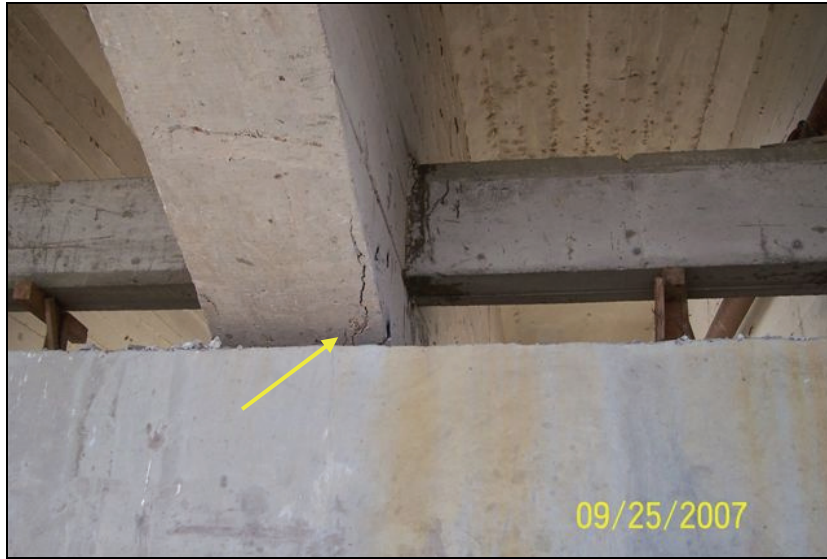
a. Interior beam
