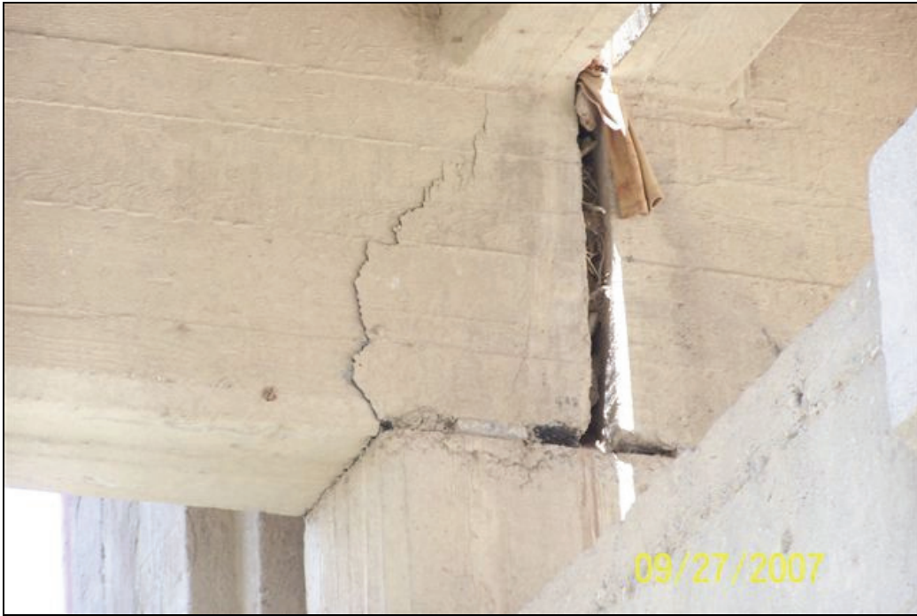
a. What appears to be a fresh shear crack in concrete beam at Pier No. 1 pedestal
