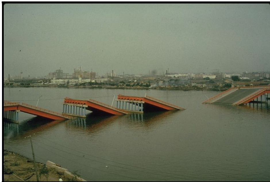
Figure 1.4: Collapse of Showa Bridge during the 1964 Niigata earthquake (after Iwasaki, 1973)
