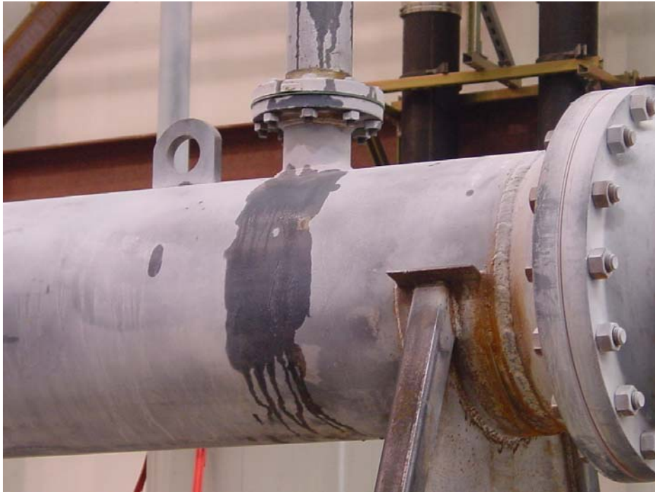
Figure 3-61 Heat Exchanger Leakage
