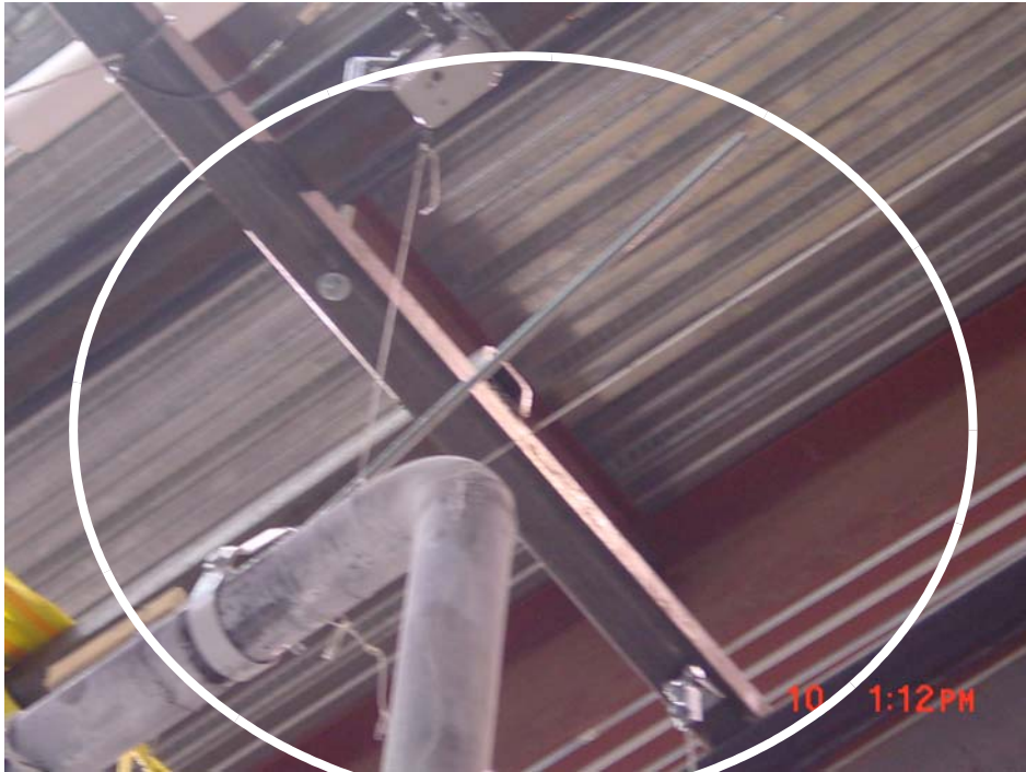
Figure 3-28 Failure of Hanger B2
