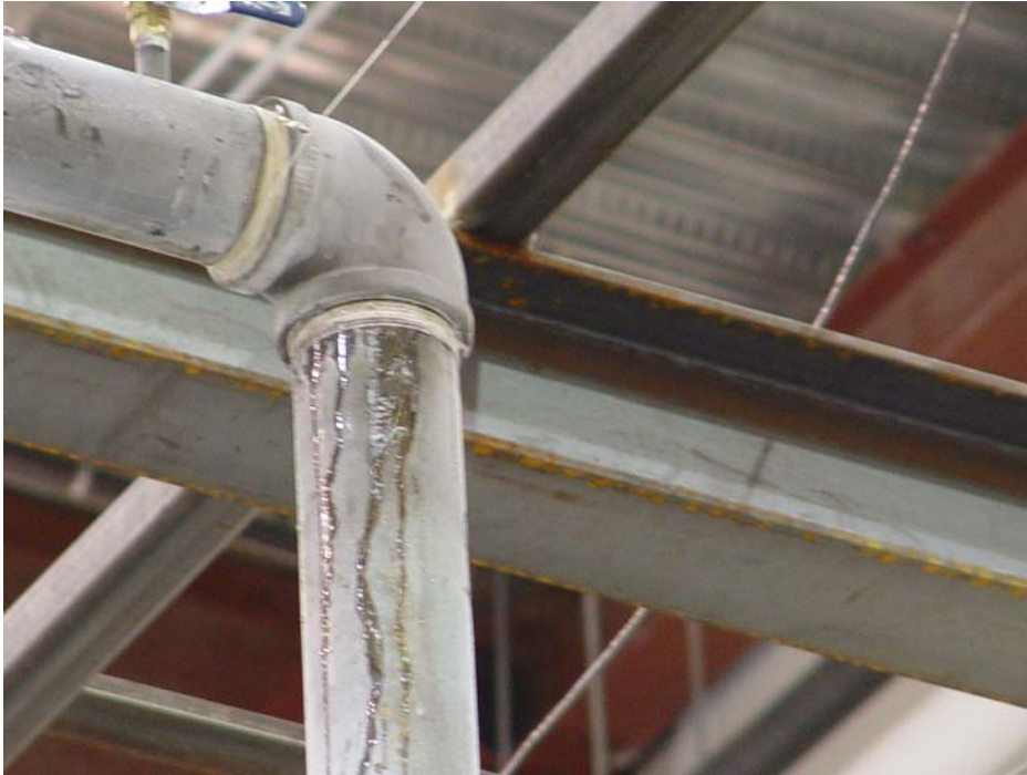
Figure 3-44 Leak Above Heat Exchanger
