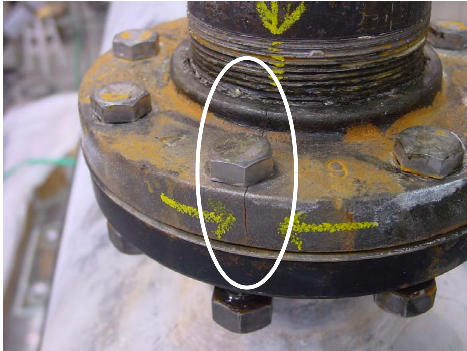
Figure 3-46 Fracture of the Flange
