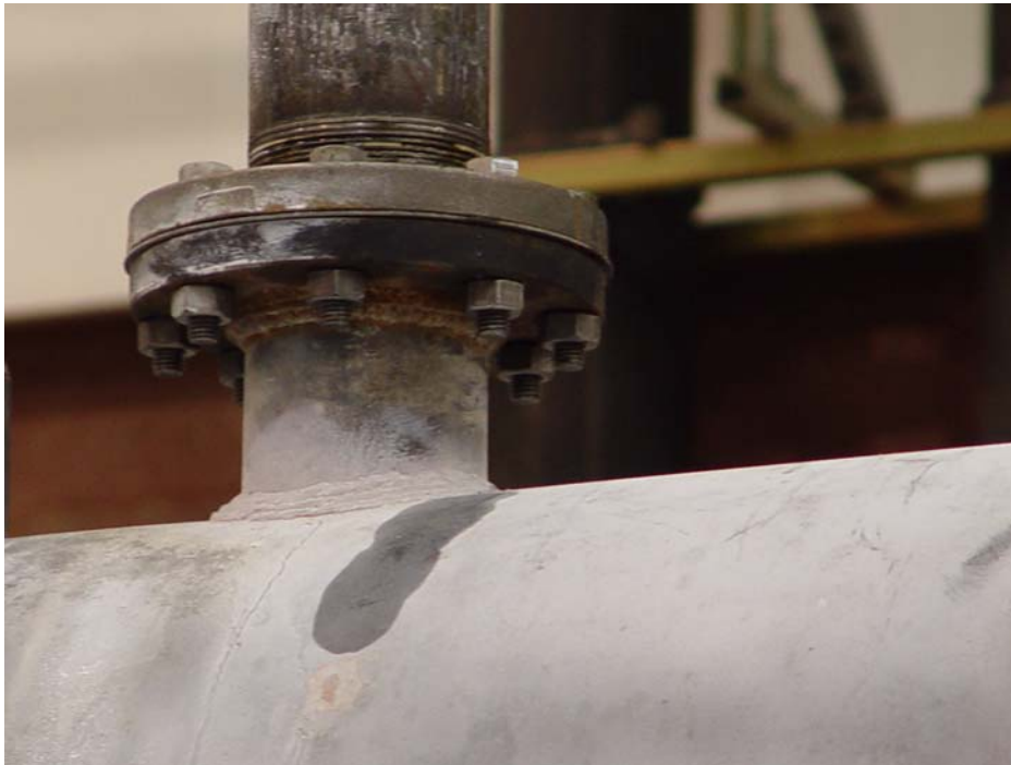
Figure 3-43 Initial Leak On Heat Exchanger Connection
