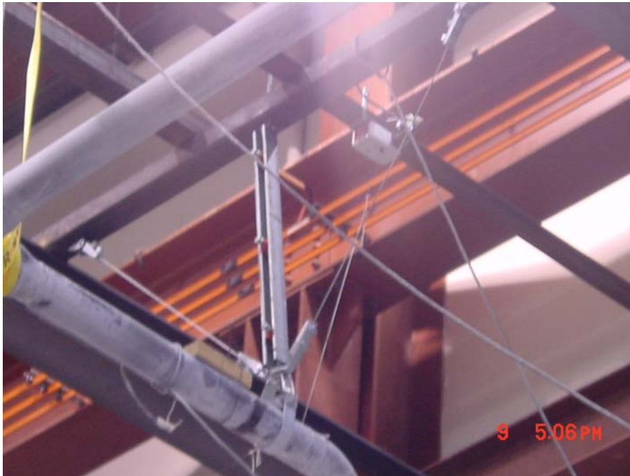
Figure 3-16 Permanent Offset of Brace B2
