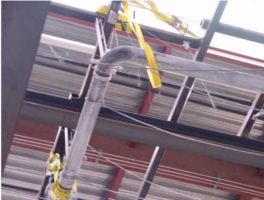
Figure 3-13 Failure of Brace B6
