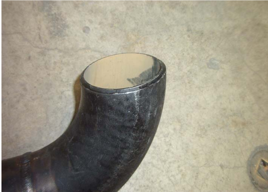
Figure 2-7 Joint Before Welding
