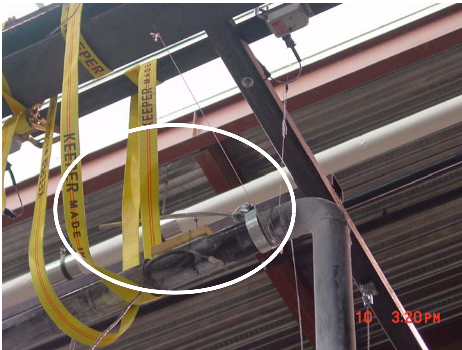
Figure 3-29 Failure of Hanger B1
