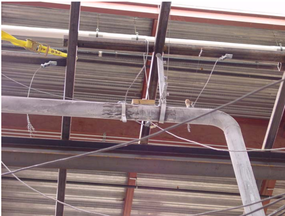
Figure 3-14 Failure of Longitudinal Portion of Brace B7
