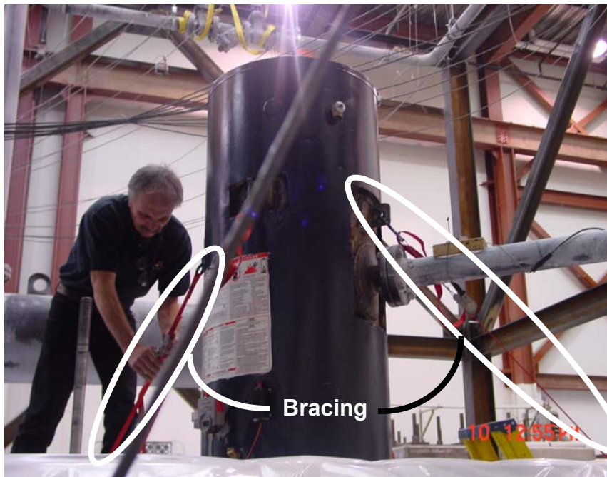
Figure 2-17 Bracing Water Heater to Table
