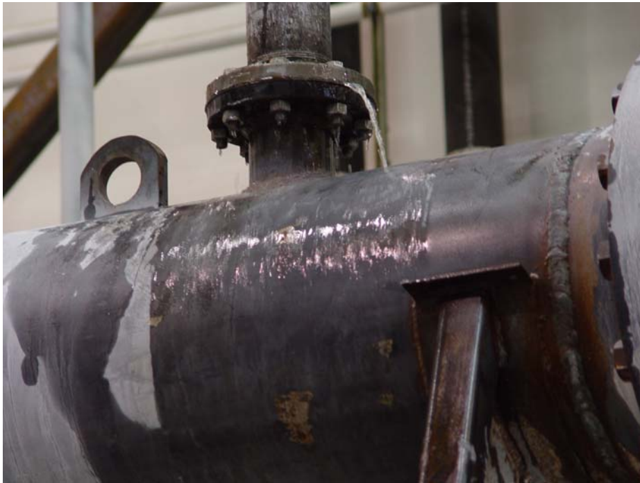
Figure 3-45 Water Flowing Out of Heat Exchanger Connection
