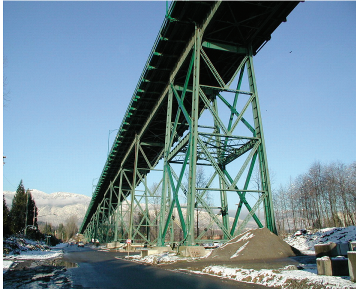
FIGURE 11-1 Braced Steel Piers
