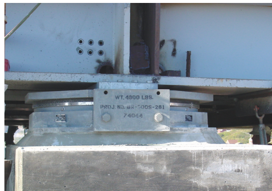
b. Friction Pendulum seismic isolator
