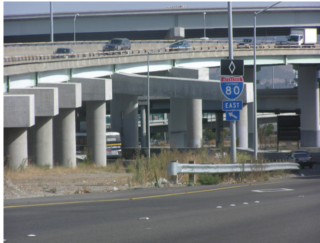
FIGURE 2-1 Reinforced Concrete Moment-Resisting Frame Construction
