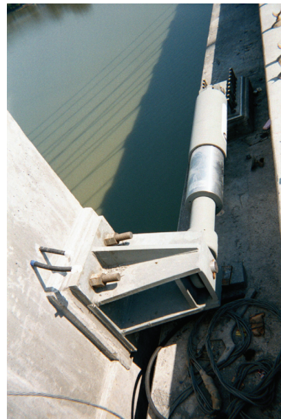
b. damper installation
