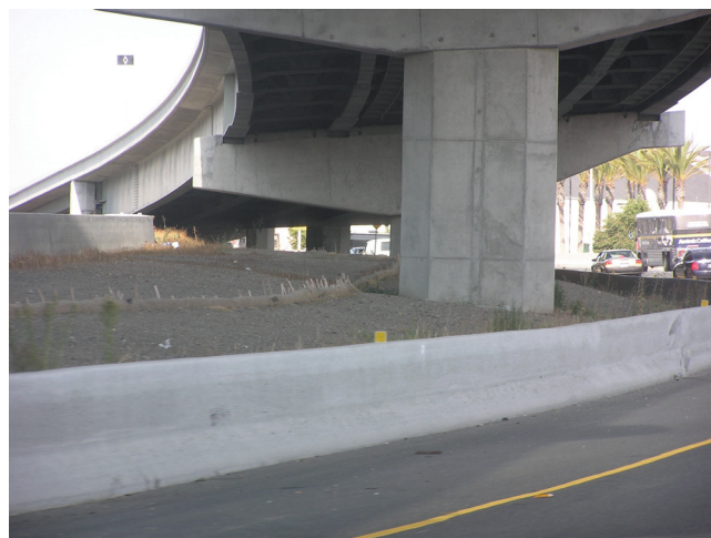
FIGURE 2-2 Reinforced Concrete Pier-Bent Cap Construction
