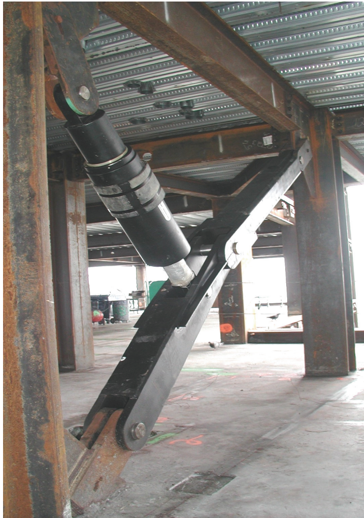
FIGURE 11-6 Reverse-toggle Brace Installation
