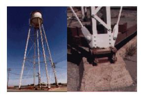
b. An application of FP bearing with uplift restrainer in an elevated water tank (<a href="http://www.earthquakeprotection.com">http://www.earthquakeprotection.com</a>)
