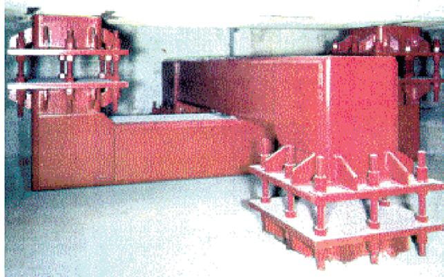
**Figure 2-13 An uplift restraint application -Excel Minami building-Kosihigaya-Japan (Mitsusaka et al., 1992)**
