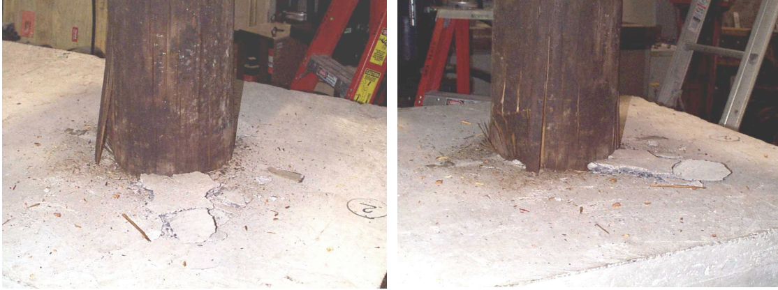
Figure 4-26. Specimen T2 connection after failing in flexural bending mode. Photo on left shows the front view; photo on right shows the rear view.
