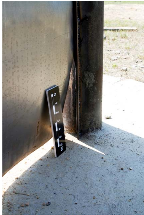
Figure 5-51 Fracture of Plate at C6 Side (Plate B2-SP56 after Test 8)
