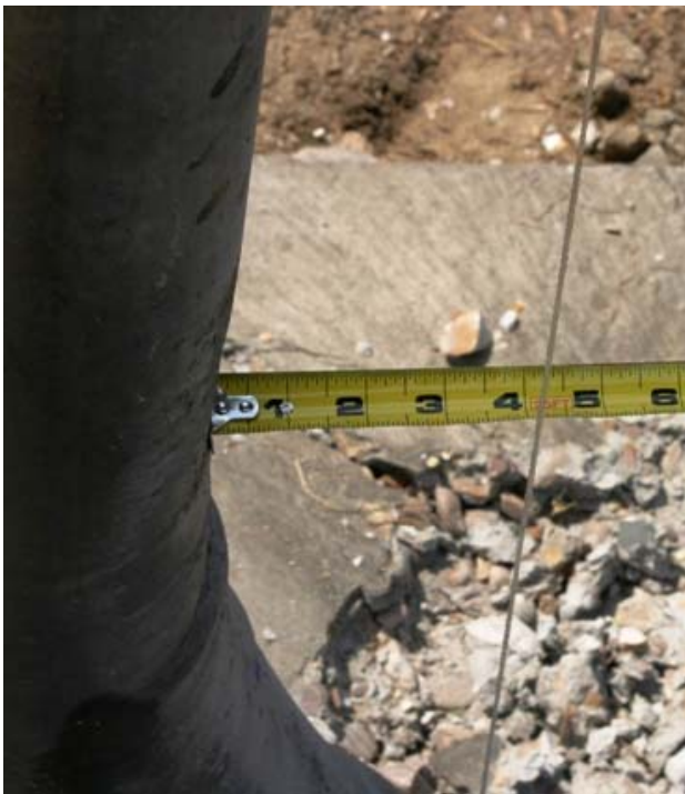
Figure 5-61 Maximum Deformation (in) of Column B2-C5 after Test 10
