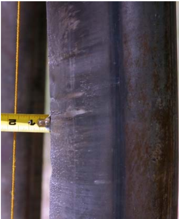
Figure 5-13 Maximum Deformation (in) of Column B1-C6 after Test 4
