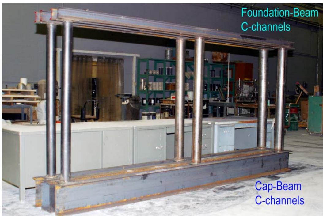
Figure 4-14 Assembly of C-channels, Columns and Connection Plates
