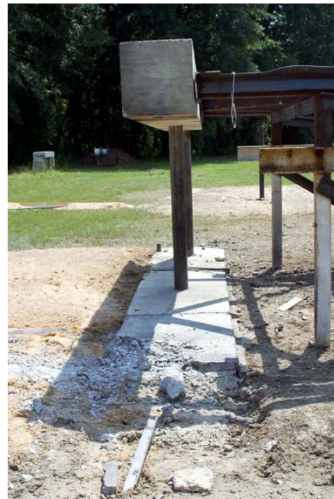
Figure 5-33 Disappearance of Column B2-C4 after Test 7
