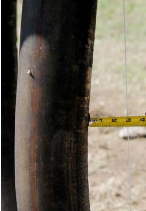
Figure 5-21 Maximum Deformation (in) of Column B1-C5 after Test 5
