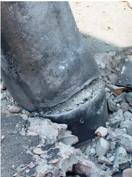
Figure 5-65 Fracture of Column (Column B2-C5, After Test 10)
