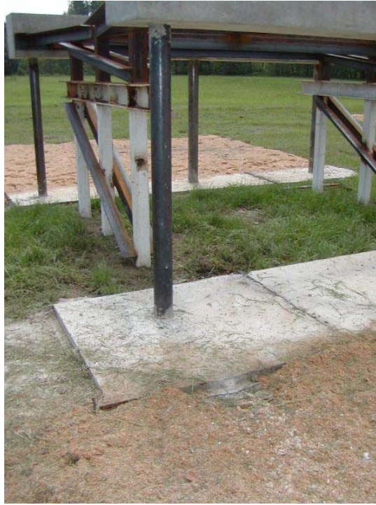
Figure 5-2 Column B1-C4 after Test 1
