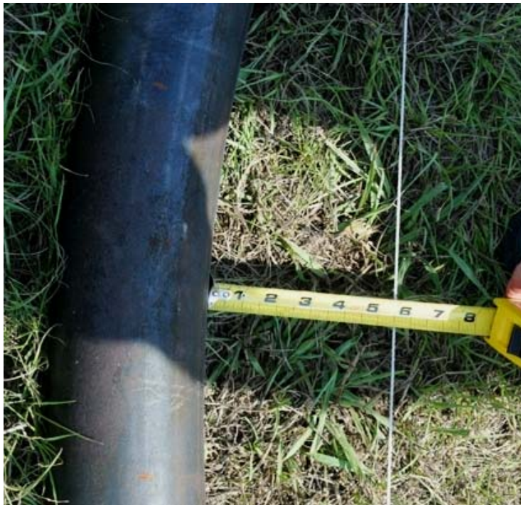
Figure 5-36 Maximum Deformation (in) of Column B2-C4 after Test 7
