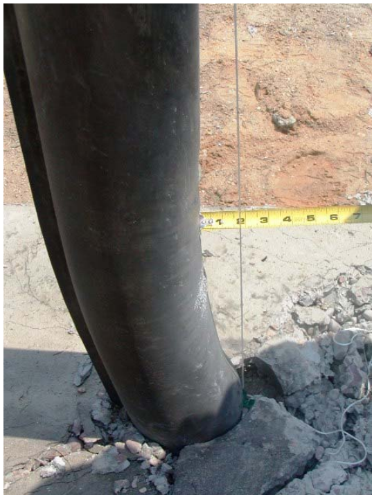
Figure 5-54 Maximum Deformation (in) of Column B2-C6 after Test 9
