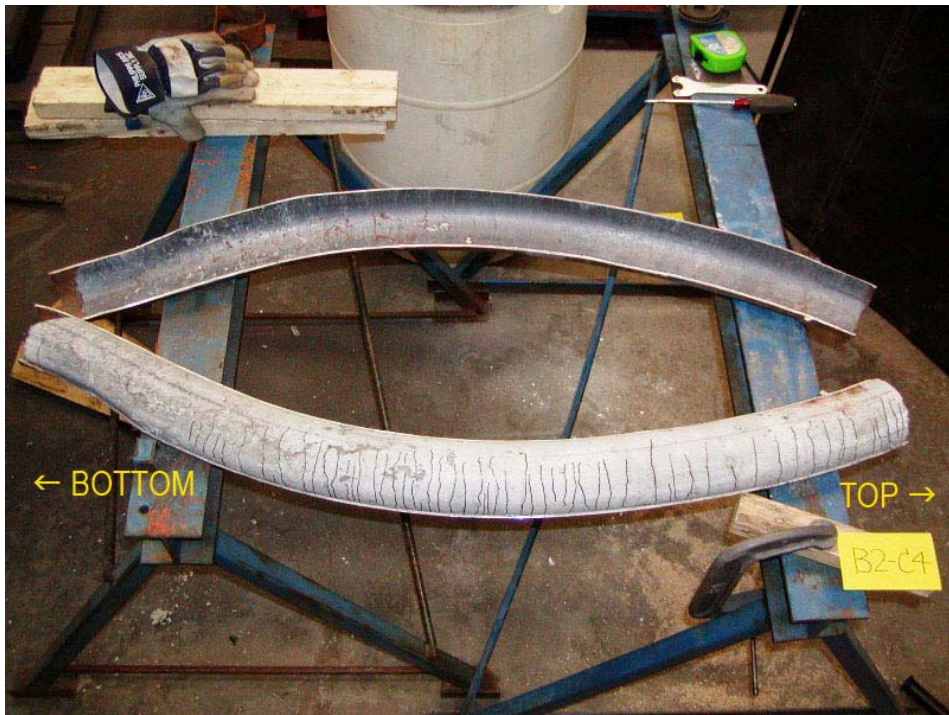
Figure 5-44 Core Concrete of Column B2-C4 after Test 7
