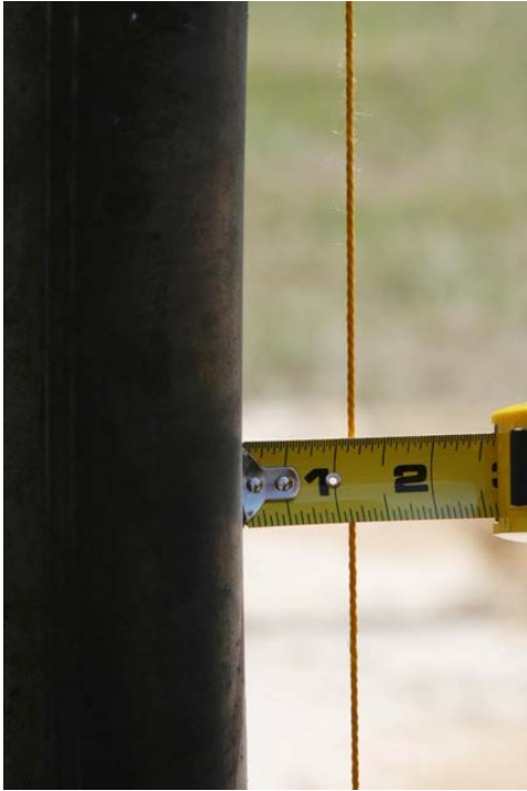
Figure 5-8 Maximum Deformation (in) of Column B1-C4 after Test 3
