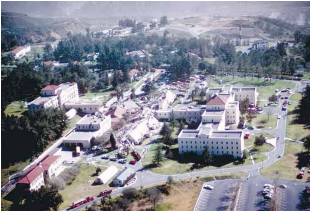
Figure 1-1. The 1971 San Fernando earthquake collapsed four buildings at the San Fernando Veterans Administration Hospital complex, killing 47 people.
