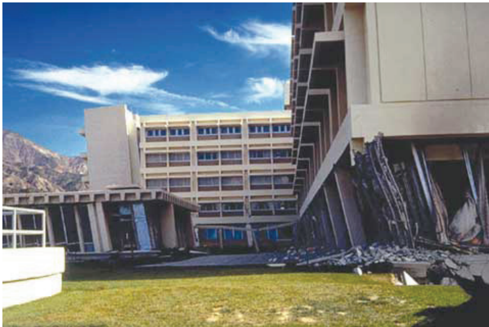
Figure 1-2. The 1971 San Fernando, California, earthquake severely damaged the “soft story” of the then-recently built Olive View Hospital in Sylmar.
