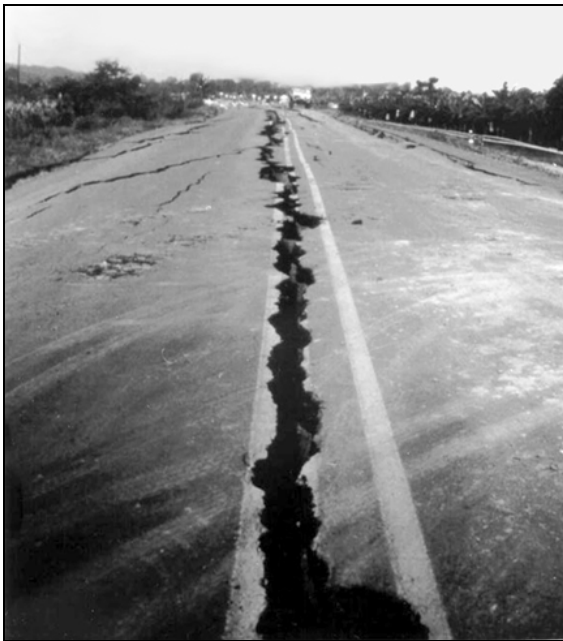
Figure 6-4. Failure mechanism beneath embankments that split, settle, and spread due to liquefaction of foundation soils.
