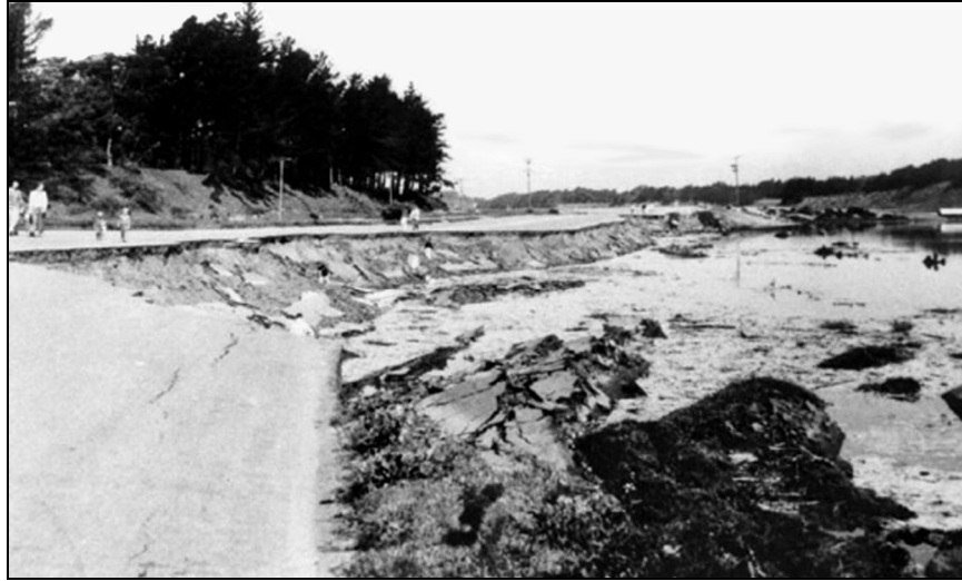
Figure 6-10. Liquefaction-induced flow failure of roadway embankment into Lake Merced during 1957 Daly City, California earthquake.
