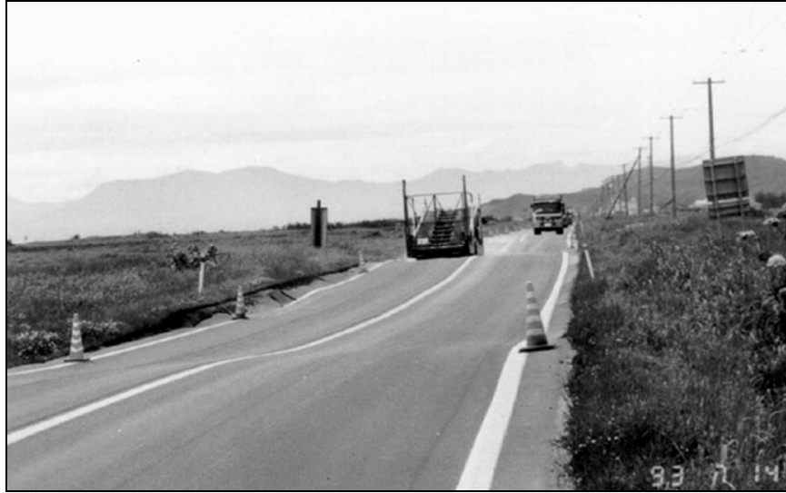
Figure 6-3. Wavy pavement due to differential settlement enhanced by liquefaction during the 1993 Hokkaido-Nansei-Oki, Japan earthquake. The site is on Highway 5 south of Oshamanbe.
