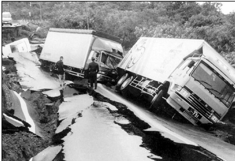
Oshamanbe Fire Department, reproduced from Harp and Youd, 1995
