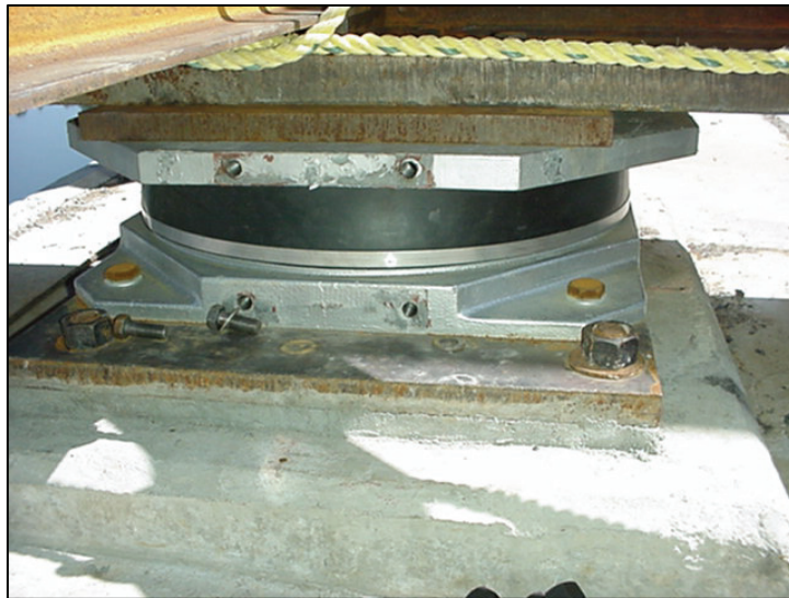
Figure 7-5. Typical Friction Pendulum Isolator
