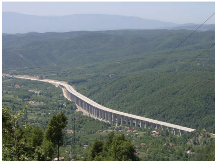
Figure 2-6. Bolu Viaduct, Trans European Motorway, Turkey
