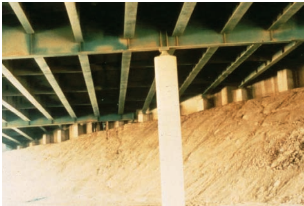
(a) Above: Single column with existing steel bearing before retrofit.
