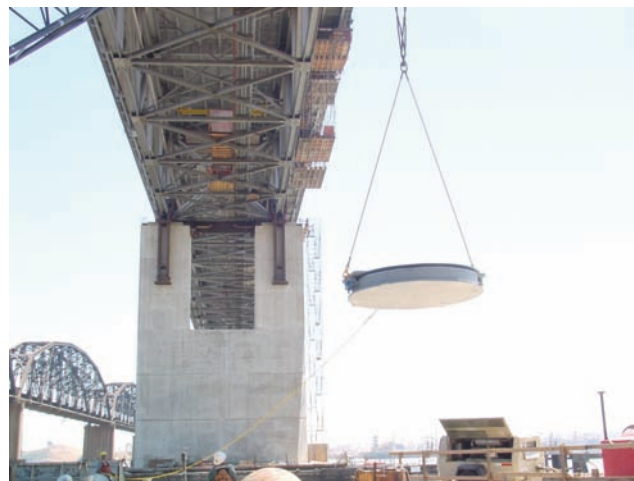
Figure 2-4. Friction Pendulum Isolator being Installed in the Benecia-Martinez Bridge, California
