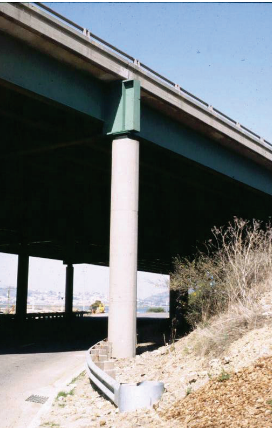
(b) Left: Replacement of existing steel bearing with lead-rubber isolator.
