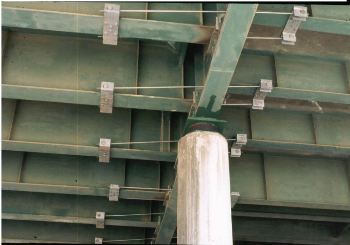
(a) Above: Single column with existing steel bearing before retrofit.
