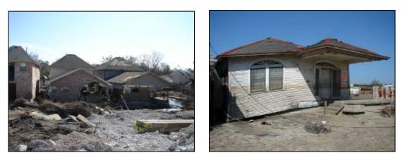
*Figure 5-17. Standing buildings within the high-velocity flooding zone adjacent to the 17<sup>th</sup> Street Canal levee breach. These buildings exemplify the WF-4 ("Destruction") damage state.*
