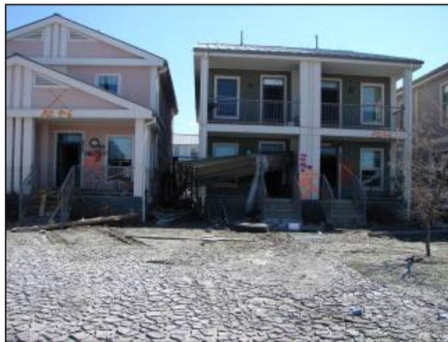
*Figure 5-15. Example of buildings in the WF-2 (“Moderate Damage”) category in a newly developed neighborhood.*
