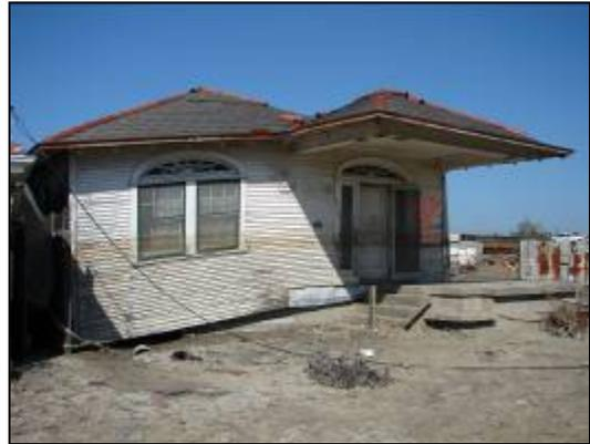
*Figure 5-17. Standing buildings within the high-velocity flooding zone adjacent to the 17<sup>th</sup> Street Canal levee breach. These buildings exemplify the WF-4 (“Destruction”) damage state.*
