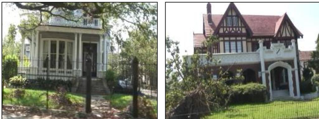
*Figure 5-13. Examples of buildings in the Garden District area classified in the WF-0 ("No Damage or Very Minor Damage") category.*
