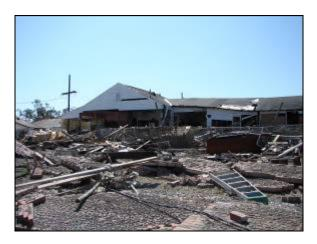
Figure 5-16. Examples of buildings in the WF-3 ("Severe Damage") category, in an older section of eastern New Orleans.
