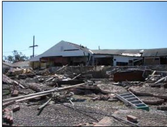
*Figure 5-16. Examples of buildings in the WF-3 (“Severe Damage”) category, in an older section of eastern New Orleans.*
