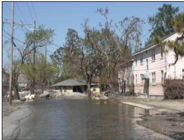
*Figure 5-18. Building washed away from its foundation in a high-velocity flooding zone adjacent to the London Avenue Canal levee breach. This building is representative of the WF-4 (“Destruction”) damage state.*
