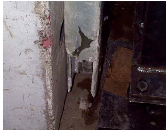
(c) outershell spalling off - bolting release
