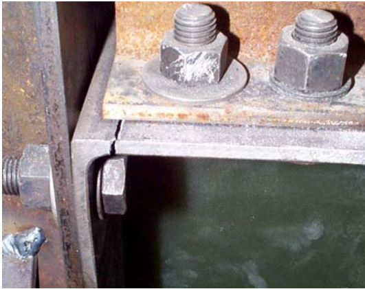
(a) Angle connection failure at top and bottom joints
