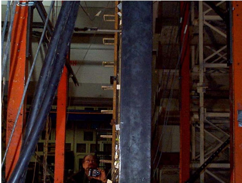
(a) Before Buckling of the Inner PMC Sandwich Panel
