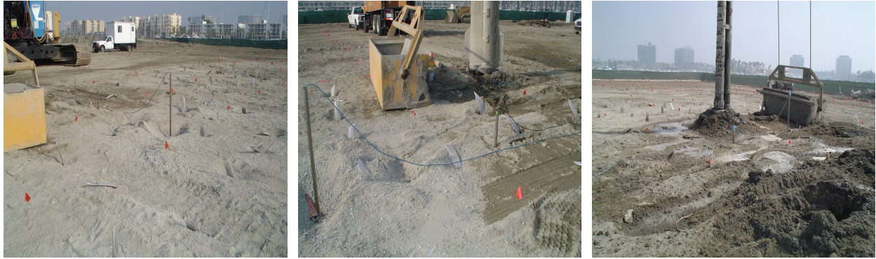
(a) Instrumentation and Wick Drains (b) Installation of Stone Columns begins (c) Stone Column Installation
