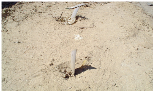
Figure 1-2. Supplementary Pre-installed Wick Drains
