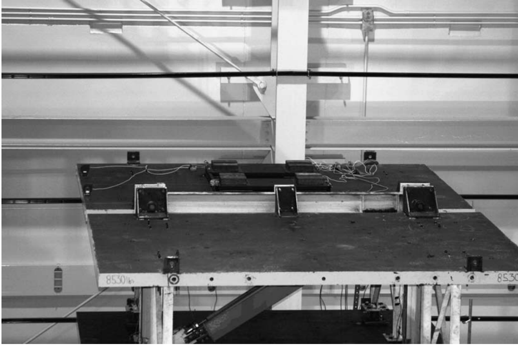
Figure 3.18. BNC Isolator on Top of Third Floor
