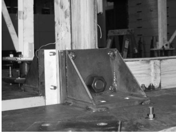
Figure 3.6. Columns Lateral Bracing
