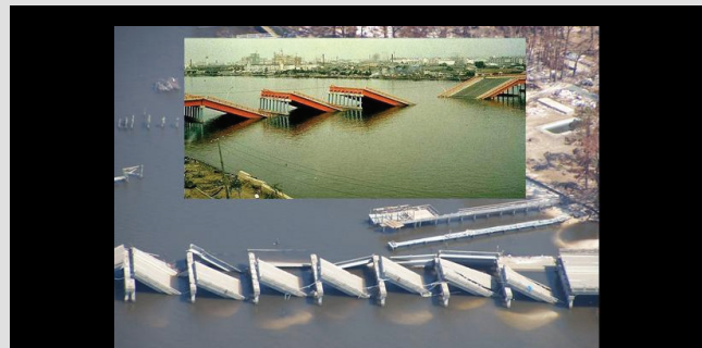
Figure 4. Bridge span collapses during Niigata earthquake (top) compared to similar damage due storm surge during Hurricane Katrina.
