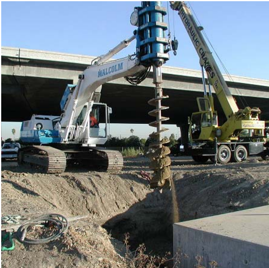
Drilling the hole for the column
