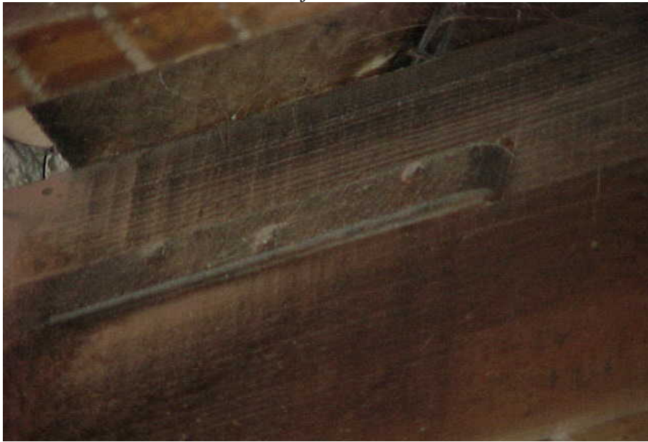
Figure 11: Details of a connection. This floor joist is supported as most are, except this floor joist has a metal strap nailed into it that is also connected to the masonry wall. Most floor joists had no such strap.
