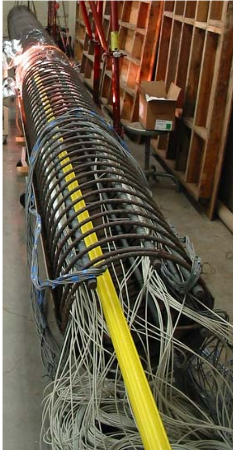
Figure 11. Column with wiring
