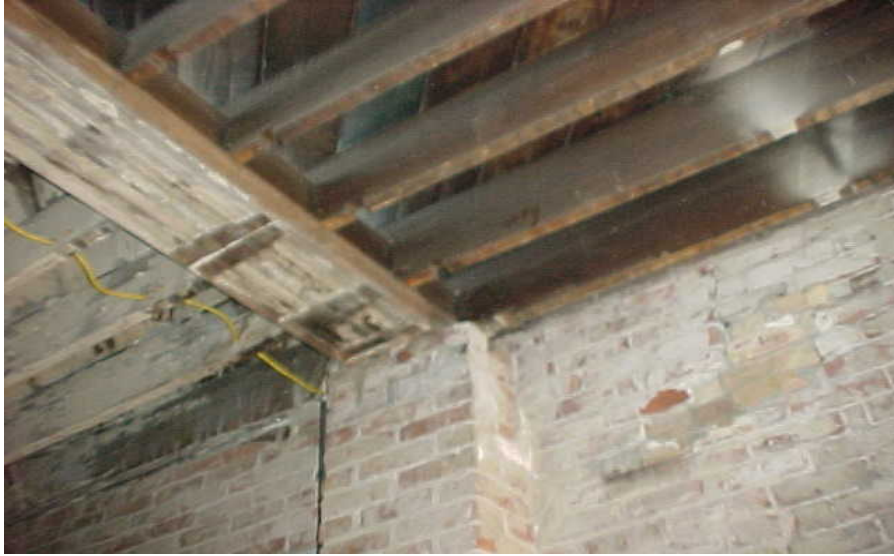
Figure 10: Supportive beam resting on brick column. This beam supports other floor joists
