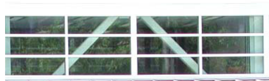
Steel cross bracing at Olin Library
