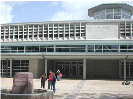
Olin Library after renovation and retrofit
