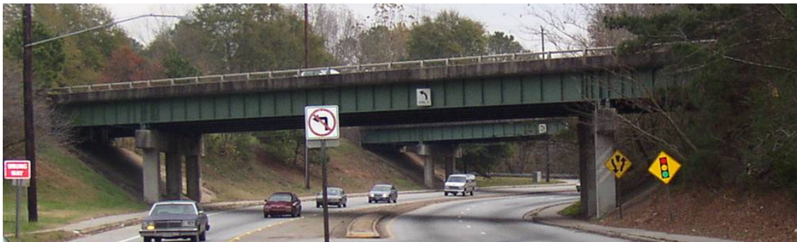
Figure 1.1: There are over 163,000 bridges in the mid-America region. This is an example of a multi-span simply supported (MSSS) steel girder bridge, the model of study in this report.
