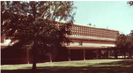
Olin Library prior to renovation and retrofit
