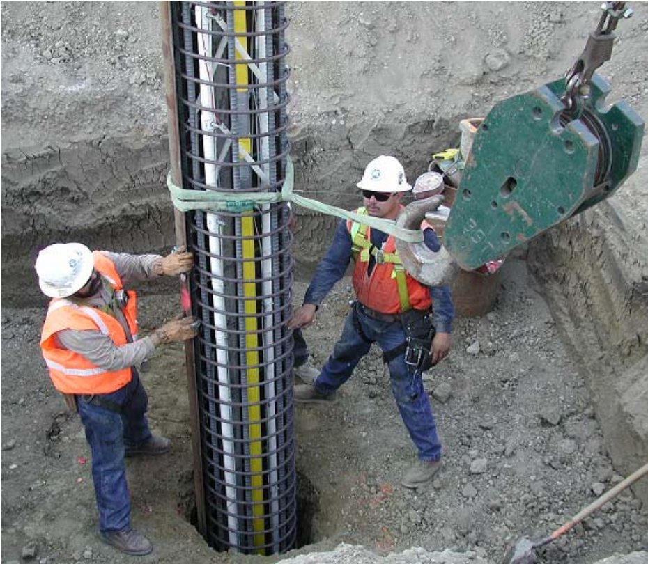
The column being inserted into the hole.
