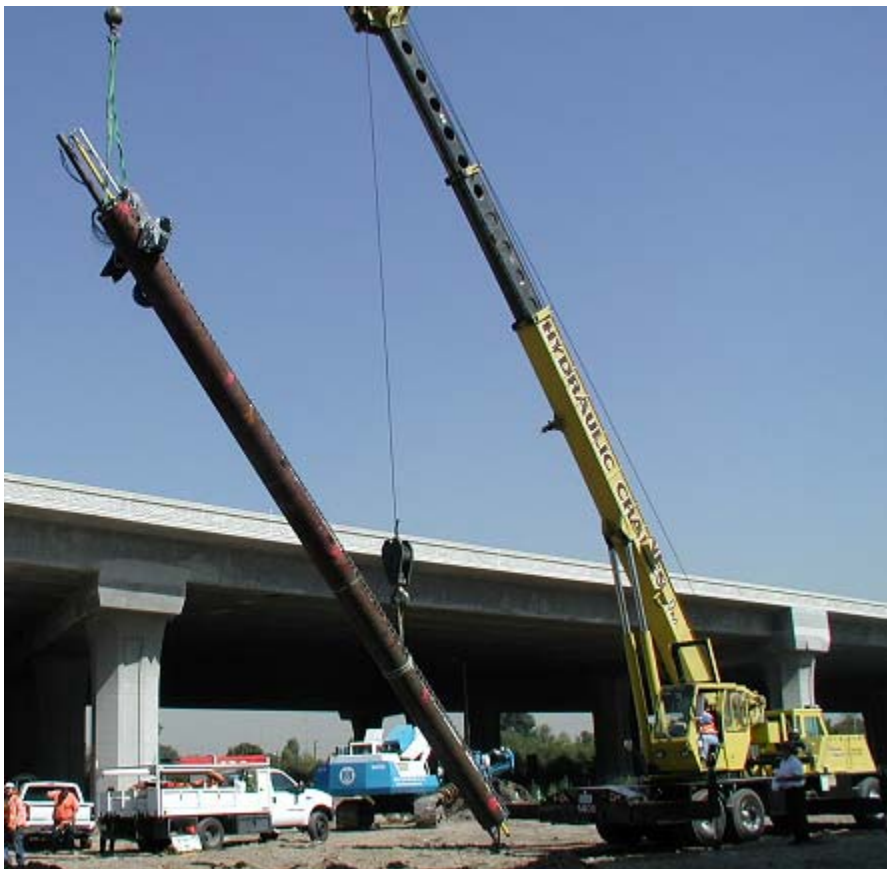
The crane lifting the column into place.
