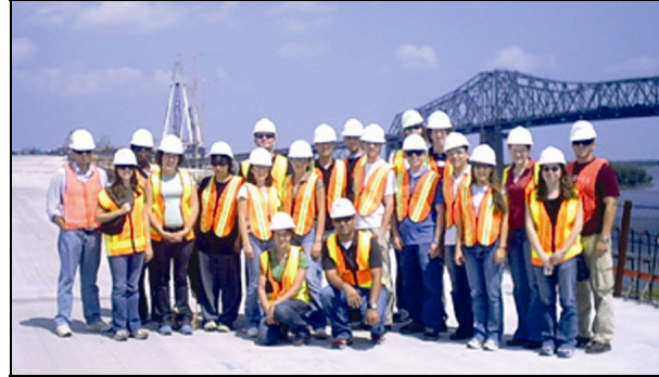
Students from the three centers toured the Cooper River Bridge with Project Manager Charles T. Dwyer. It will be the largest cable-stayed span bridge in North America when completed next summer.
