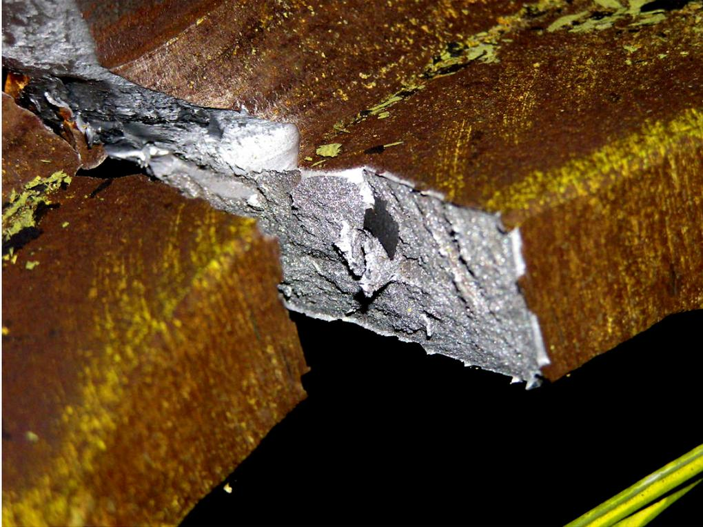
(e) Bottom flange rupture detail
