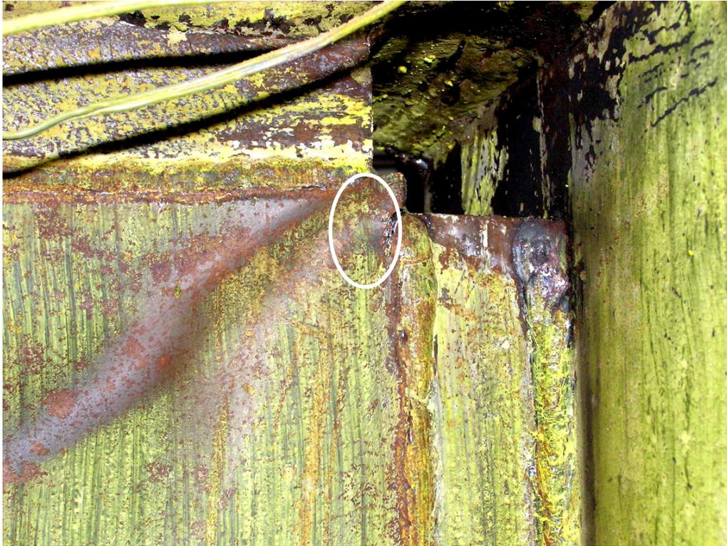
(c) Top A-side corner of infill at far column fishplate
