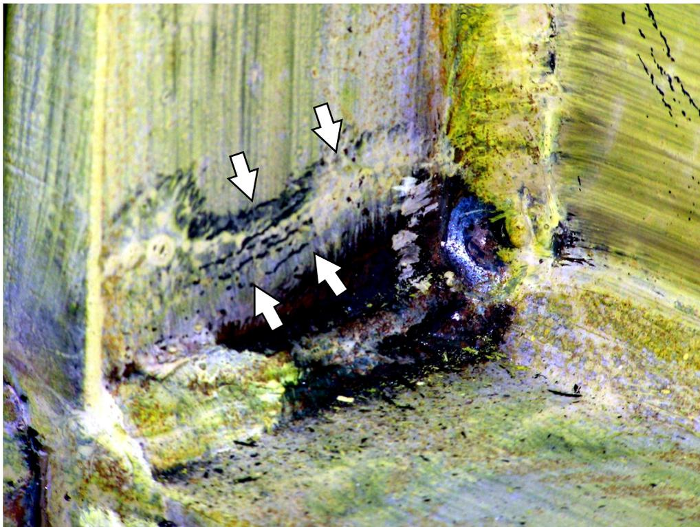
(b) Bottom flange weld to wall flange of far column
