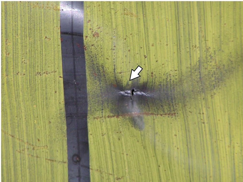
**FIGURE 5-60 Panel fracture near bottom of wall column
