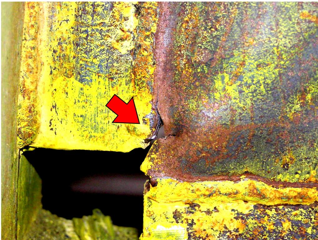
(f) Infill panel crack at wall bottom corner
