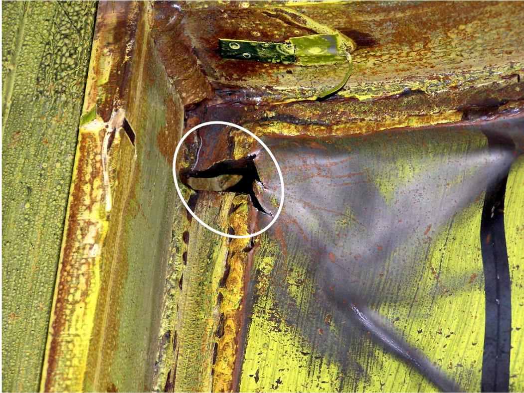
(g) Panel tear at wall arch to column connection
