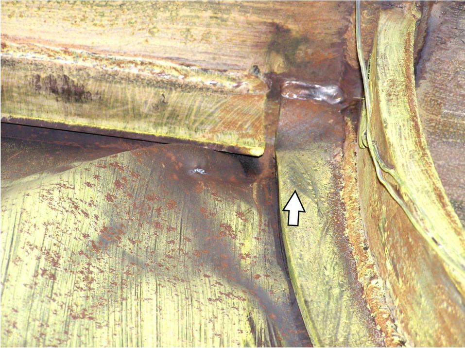
(b) Arch to beam flange connection
