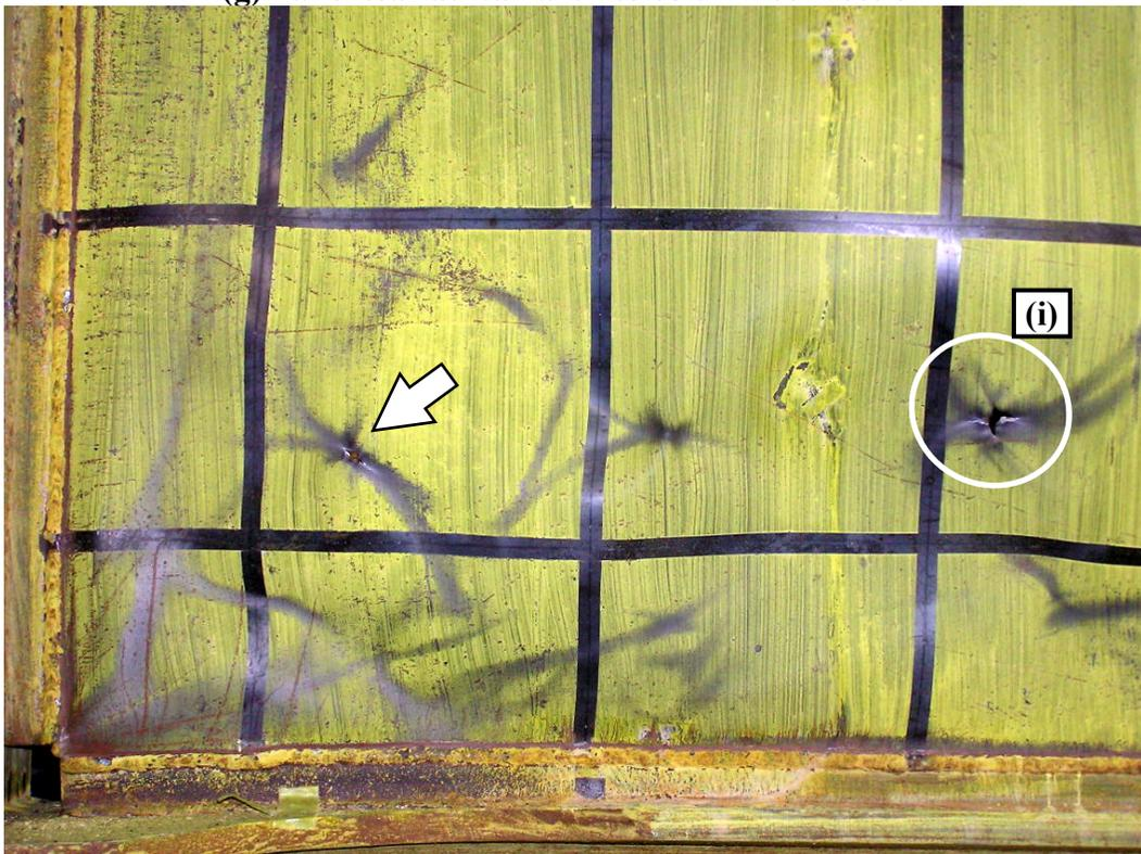
(h) Fatigue tears near bottom beam, wall side
