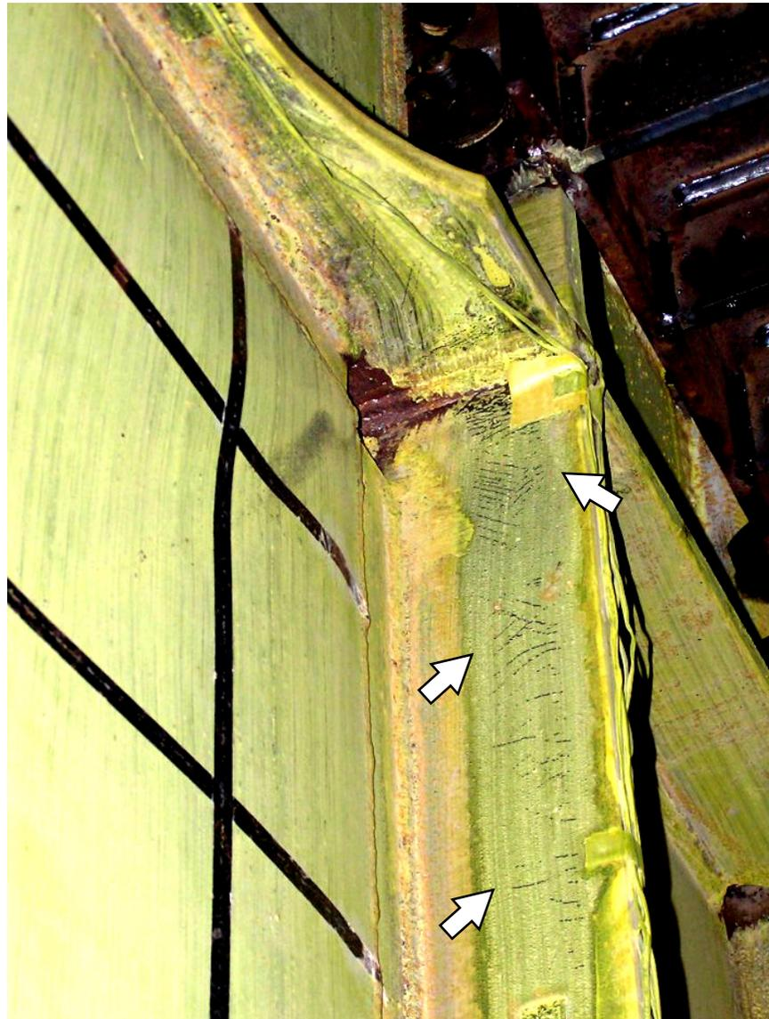
**FIGURE 5-79 Far column wall flange yielding near top beam
