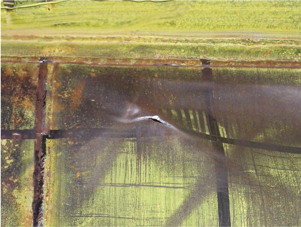
(e) Fatigue tear near top beam, far side
