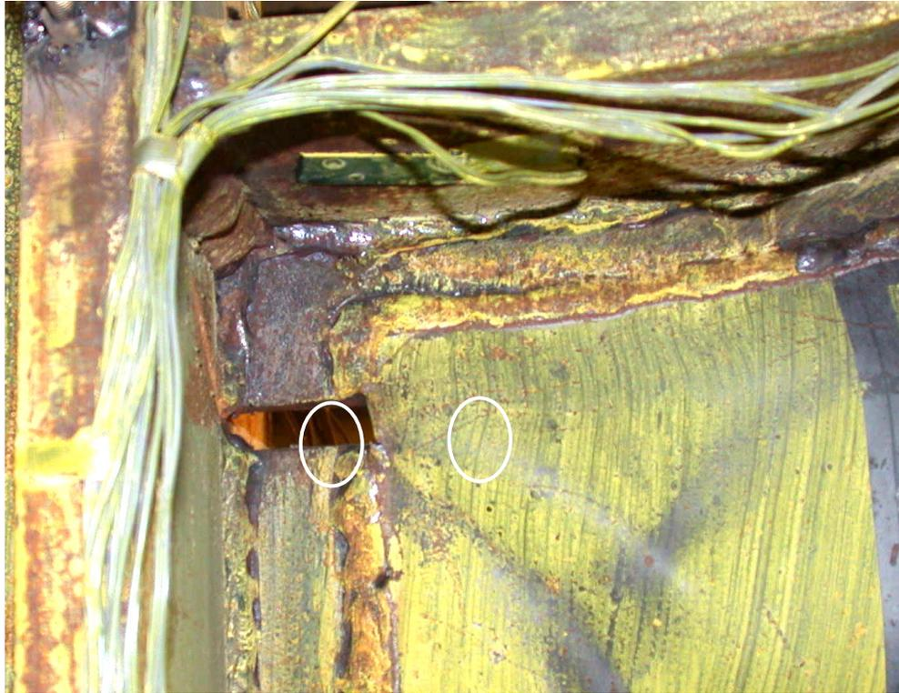
**(a) Infill panel crack at wall column/wall arch**
