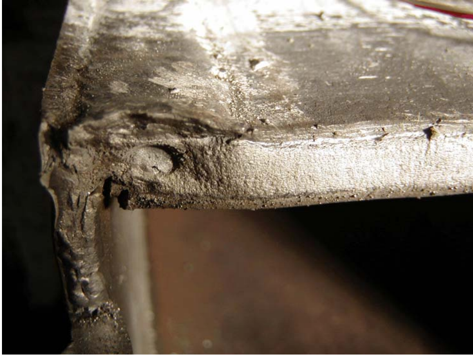
FIGURE 5-16 Fracture Surface on Link Side-1
