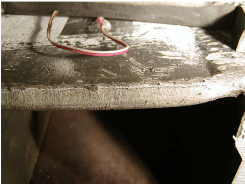
FIGURE 5-17 Fracture Surface on Link Side-2
