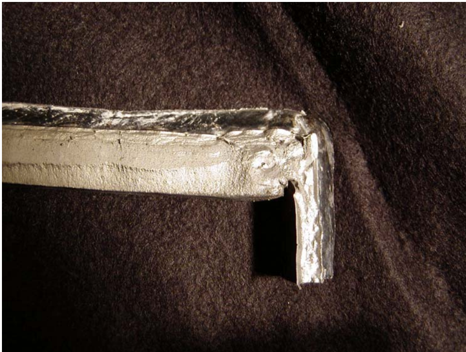
FIGURE 5-21 Fracture Surface on Brace-to-Beam Connection Side-3
