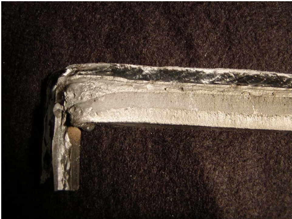
FIGURE 5-19 Fracture Surface on Brace-to-Beam Connection Side-1
