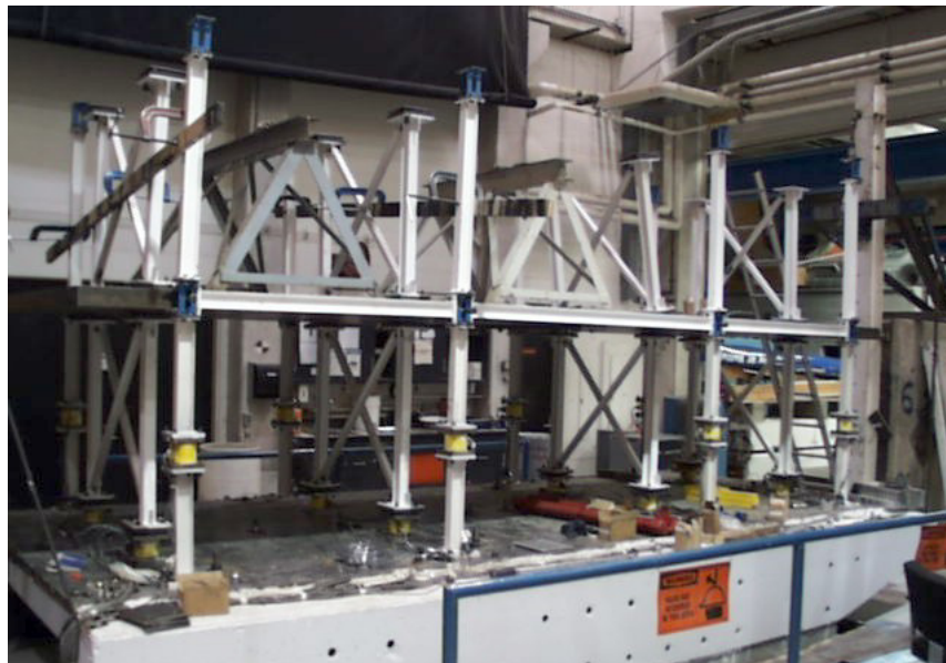
Figure D.6 Construction of the Second Floor
