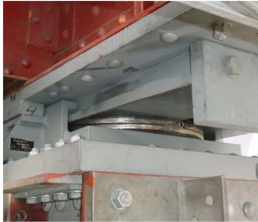
Figure 1-4: View of uni-directional FP bearing with uplift restraint installed at the San Francisco approach to the Oakland Bay Bridge.
