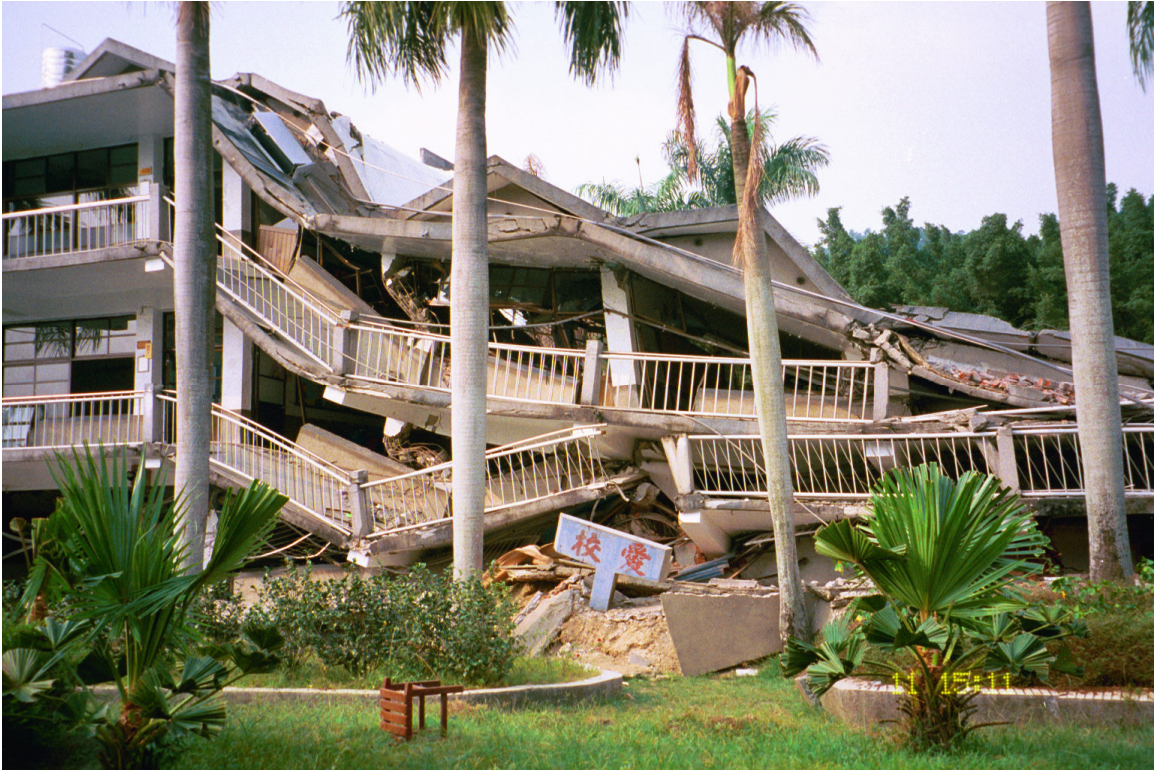
Figure 4-2 Collapsed Middle School Building in Central Taiwan Due to Surface Rupture of Chelungpu Fault in September 1999
