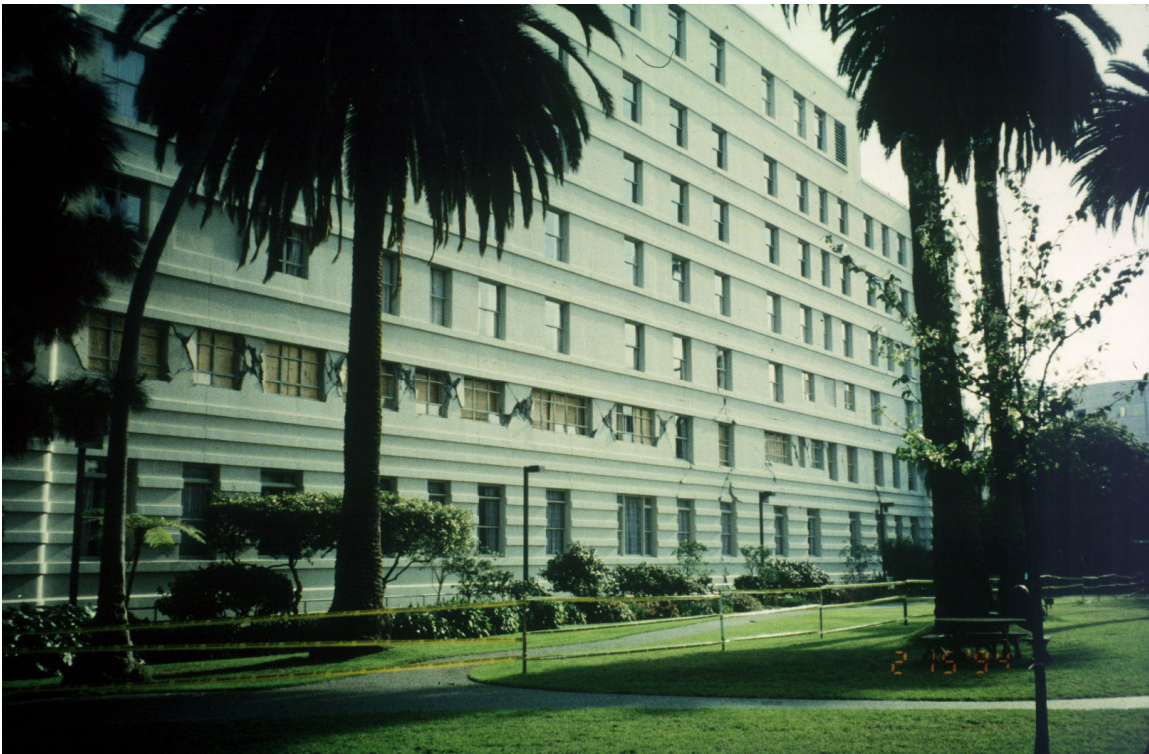
Figure 2-2 Saint John's Hospital and Health Center in Santa Monica, California, Damaged by the Northridge Earthquake in 1994
