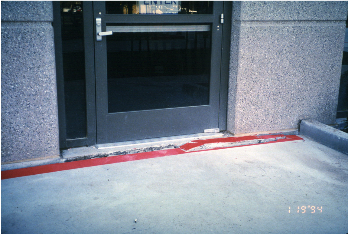
Figure 8-1 Liquefaction-Induced Settlement of Slab on Grade Adjacent to Pile-Supported Hospital Building in Woodland Hills from the Northridge Earthquake
