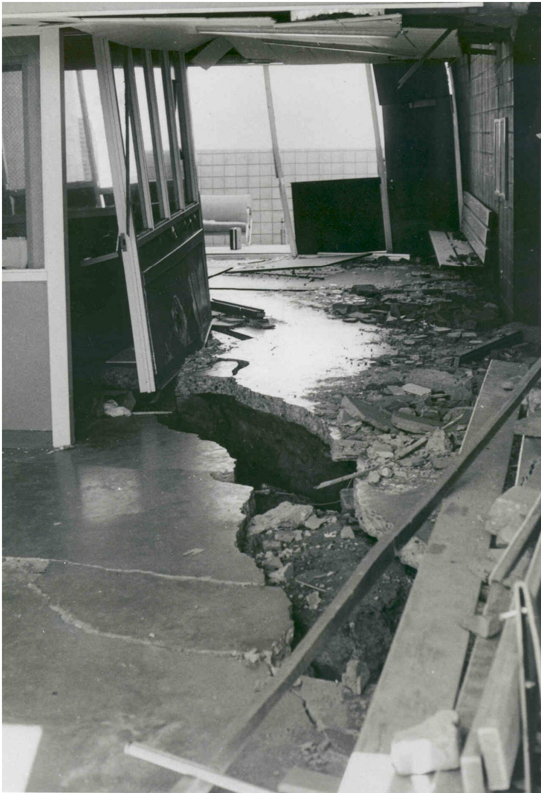
Figure 4-1 Liquefaction and Lateral Spreading Damage to Los Angeles County Juvenile Hall Facility, Sylmar, California. Photograph Courtesy of Jack Meehan
