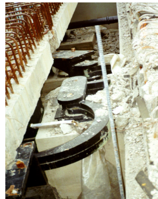
Figure 7. Failure of Yielding Steel Device Connections at Expansion Joint
