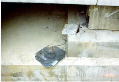
Figure 6. Failed Sliding Bearings
