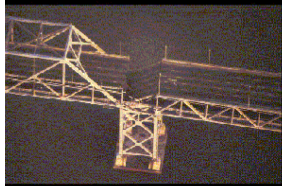
Figure 3. Damage to Bay Bridge after Loma Prieta Earthquake
