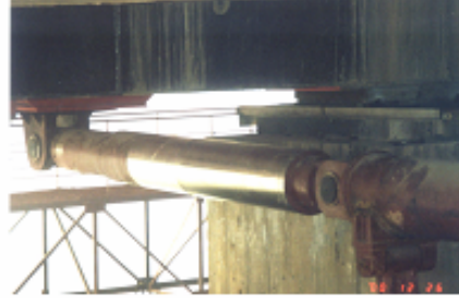
Figure 2. Setting viscous dampers
