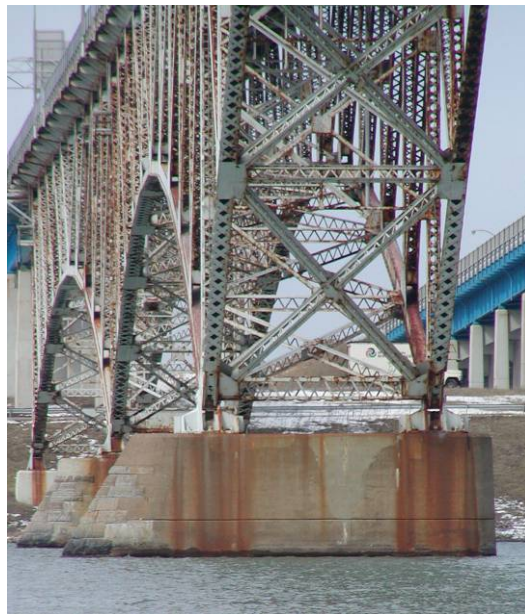
Figure 1. Typical Steel Truss Pier
