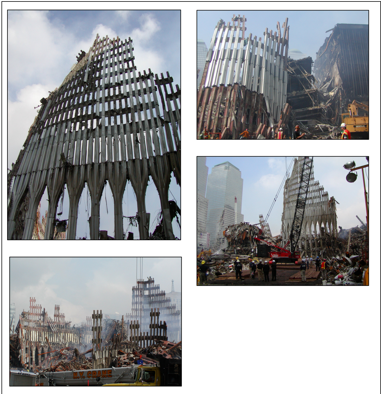
Figure 5-5. Three-column panels in down-down-down-down pattern
