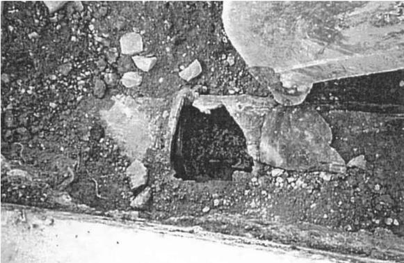
**Figure 1-3 Slip-Out of Joint on 450 mm Dia. Cast Iron Pipe from the Kobe Earthquake (Ref: Iwamoto 1995)**
