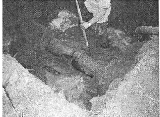
**Figure 1-2 Cracked Bell on 200 mm Dia. Cast Iron Pipe from the Northridge Earthquake (Ref: LADWP 1999)**
