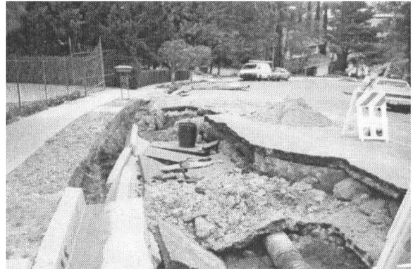
**Figure 1-8 Failure of 300 mm Dia. Steel Main from the Northridge Earthquake (Ref: LADWP 1999)**
