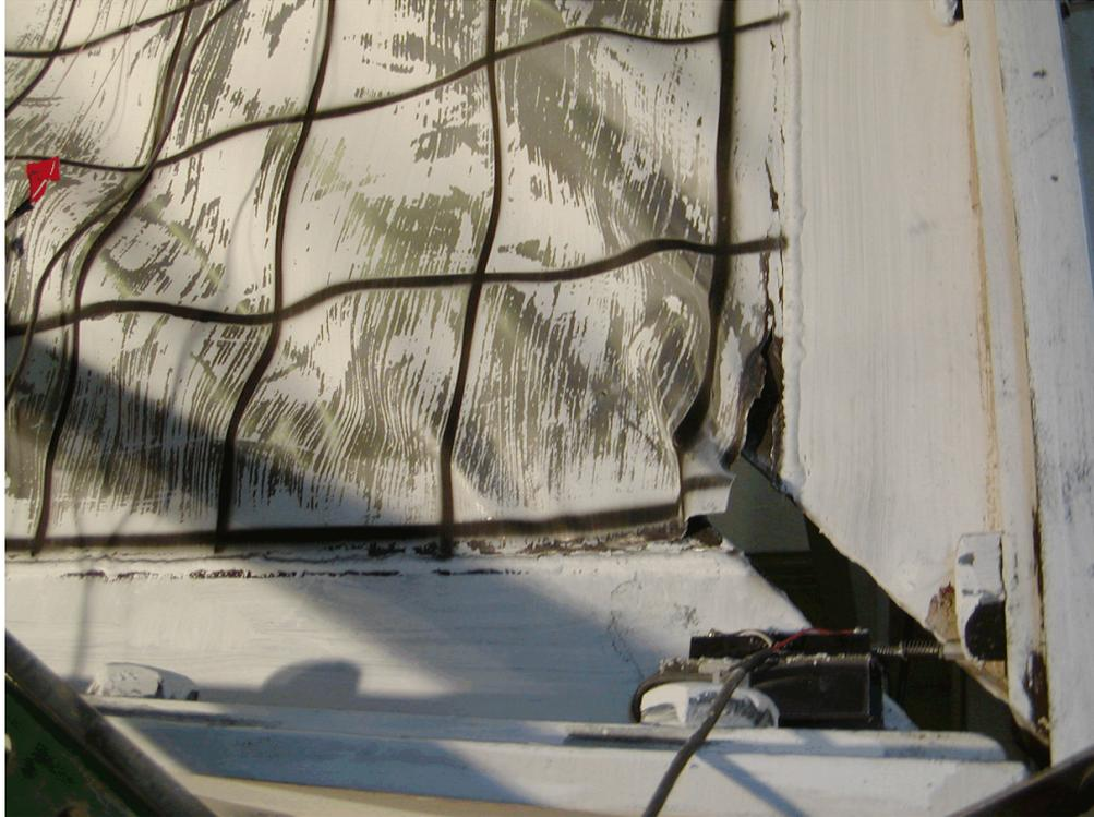
**FIGURE 5-57 Infill Fracture in Lower South Corner
