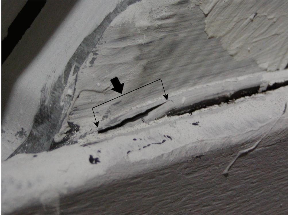
**FIGURE 5-15 Epoxy Crack Along Bottom Beam
