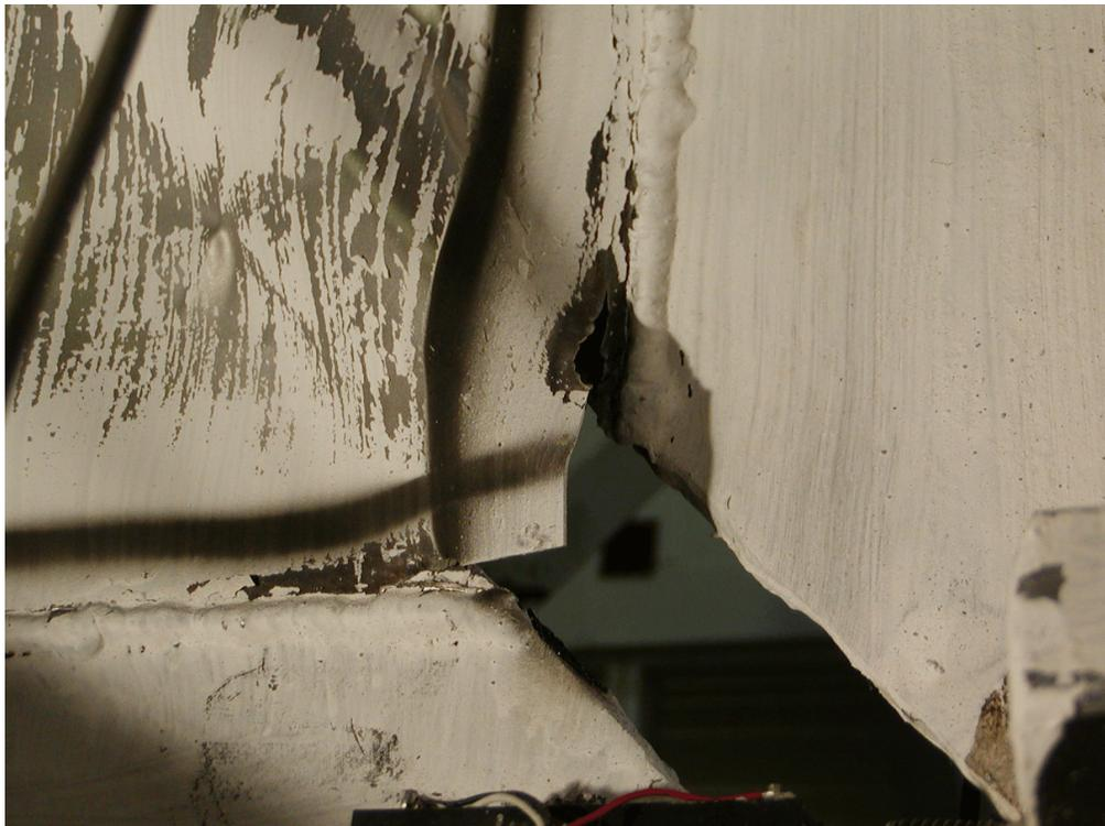
**FIGURE 5-46 Infill Fracture in Lower South Corner
