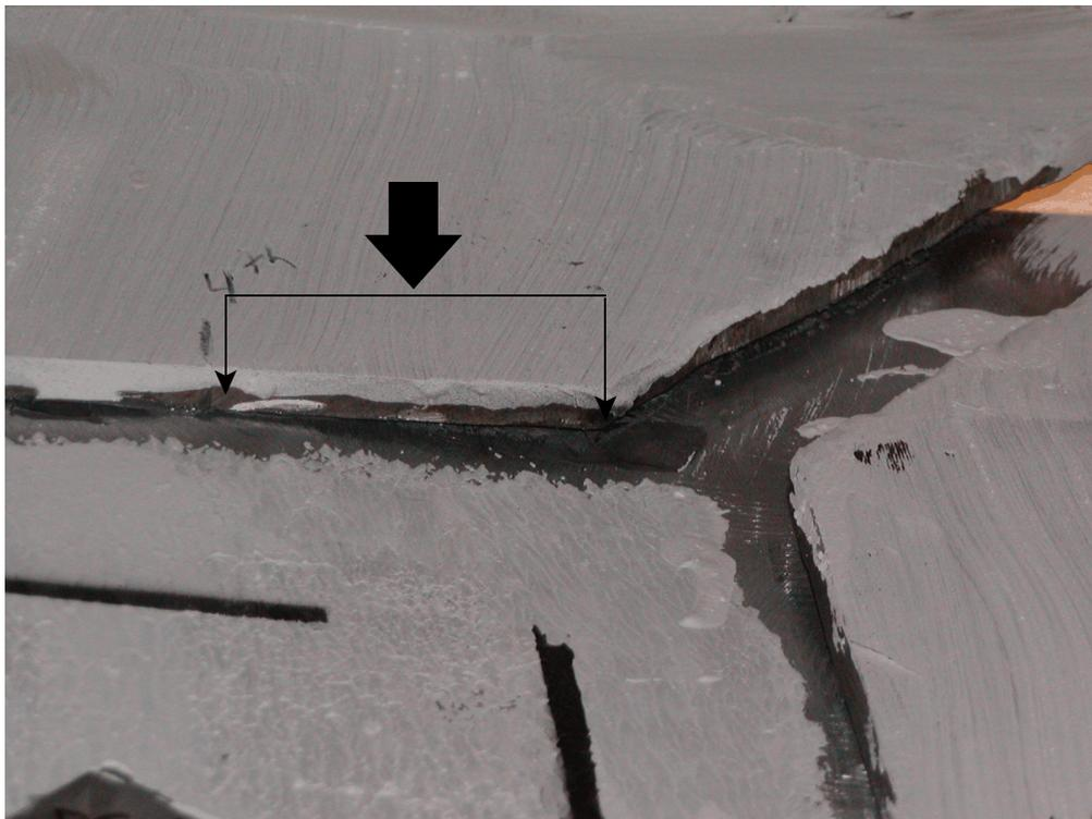
**FIGURE 5-6 Epoxy Crack - North End of Top Beam
