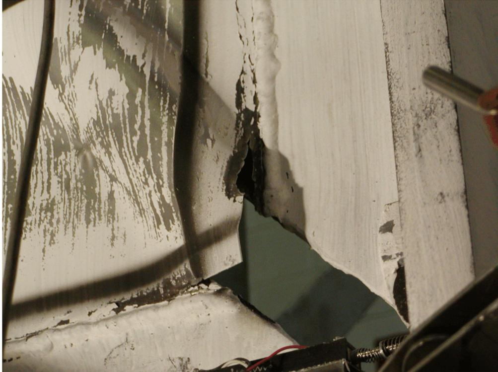
**FIGURE 5-51 Infill Fracture in Lower South Corner
