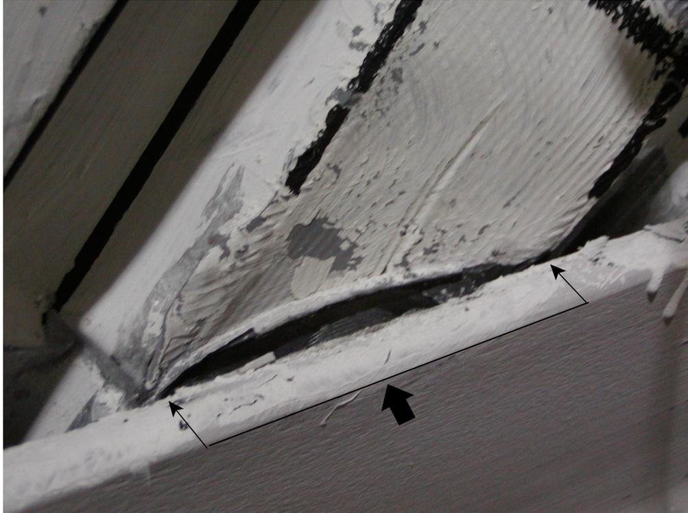
**FIGURE 5-21 Epoxy Crack Along Bottom Beam
