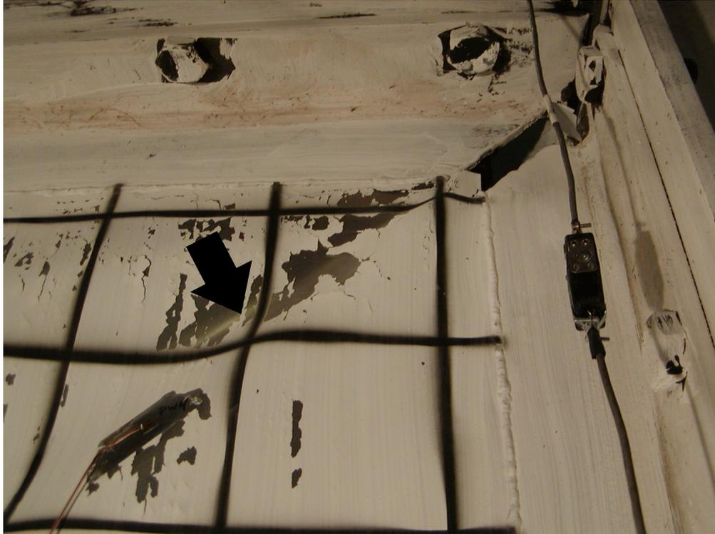
**FIGURE 5-39 Plastic Fold in Upper South Corner
