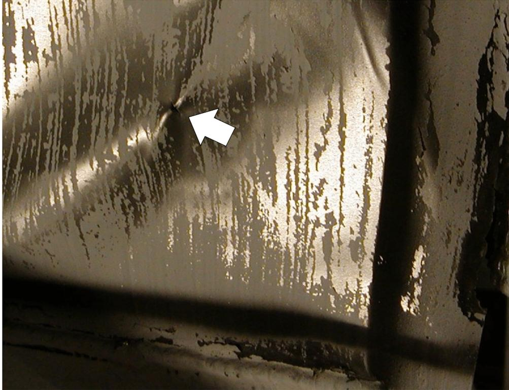
**FIGURE 5-53 Infill Tear Near South Corner
