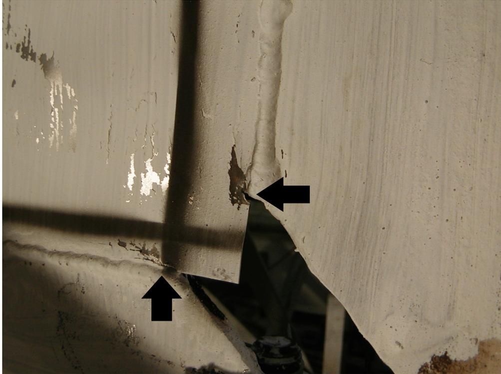
**FIGURE 5-37 Infill Fracture in Lower South Corner
