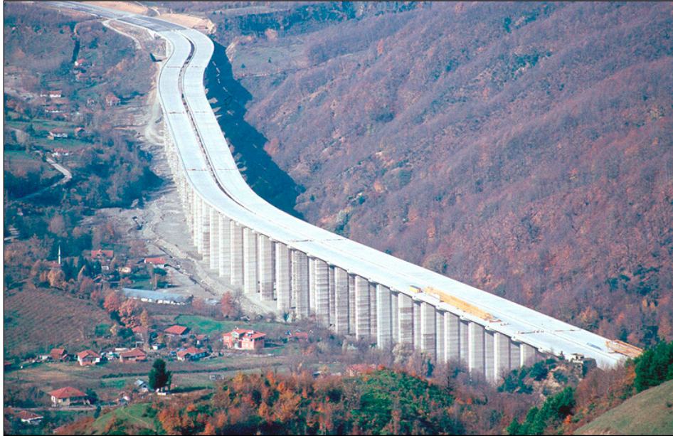
Figure 1. General View of Bolu Viaduct
