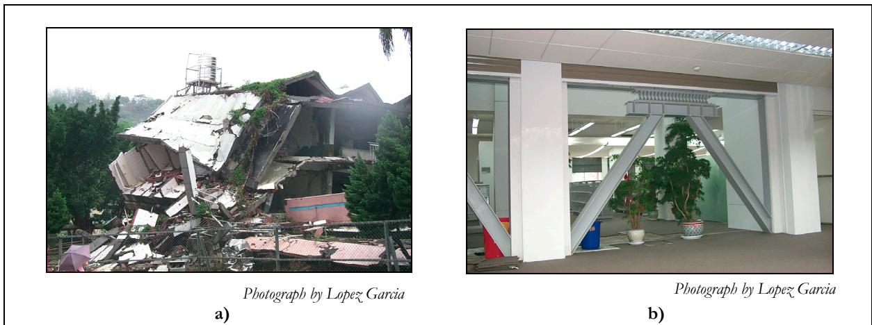
Figure 4. (a) Collapse of school building; (b) Library building retrofitted with metallic dampers
