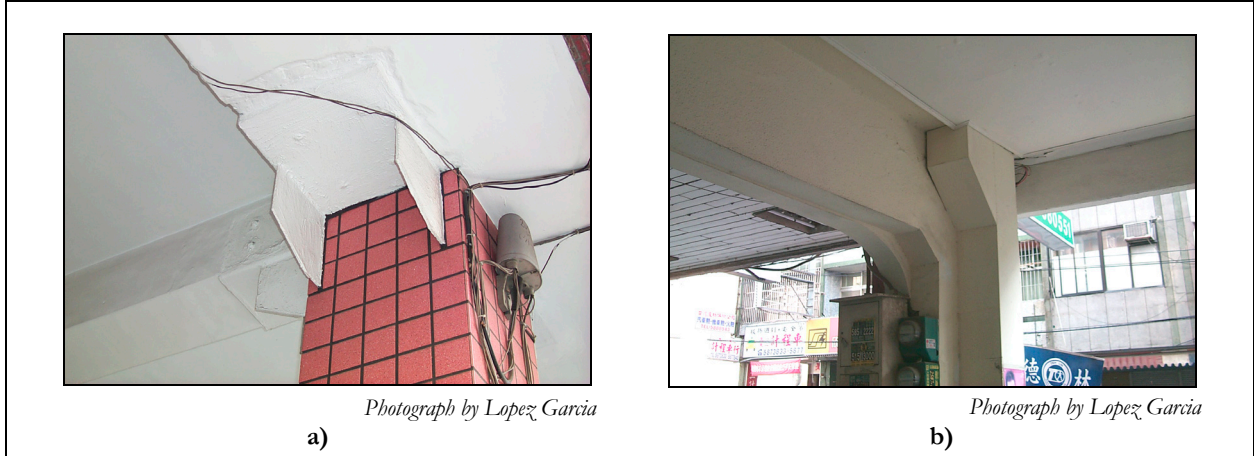
Figure 2. Non-engineered retrofit of residential buildings: (a) beam-column joint retrofitted with steel plates; (b) structure strengthened by a new column
