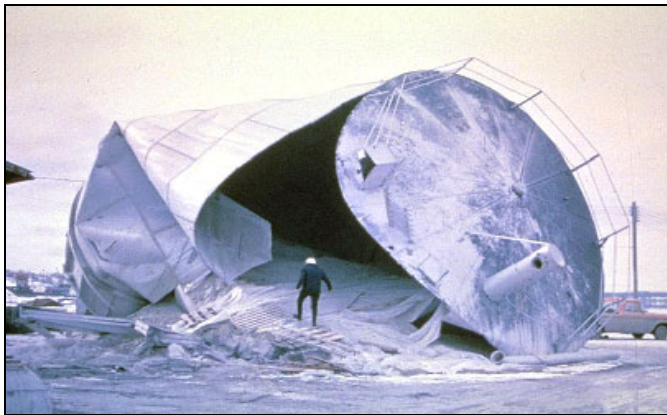
Figure 8 - Collapsed tank; Anchorage Earthquake. March 1964.
