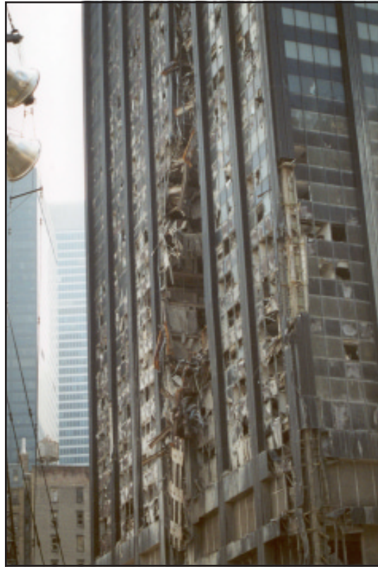
b. View of northern and western facades
