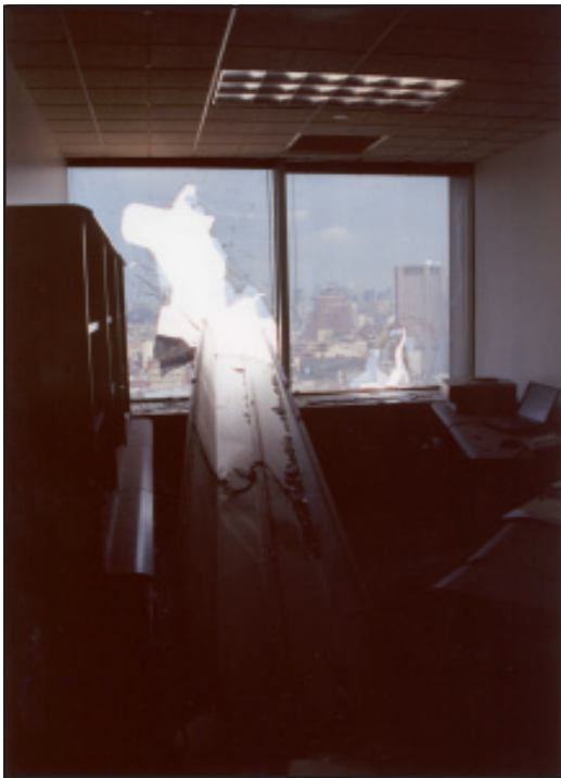
a. Penetration of WTC 2 fascia piece
