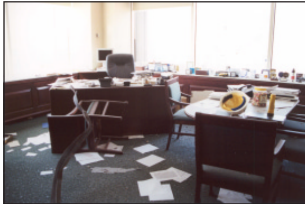
b. Typical damage in office space
