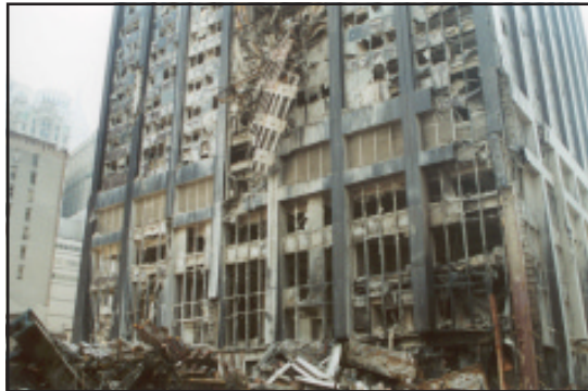
c. View of lower 10 stories of northern facade
