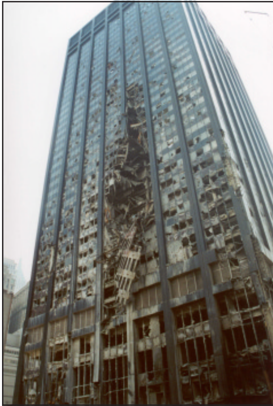
a. View of northern facade
