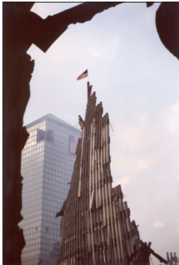
Figure 2.11. View of the WTC 2 façade looking north-west from the foyer of the building
