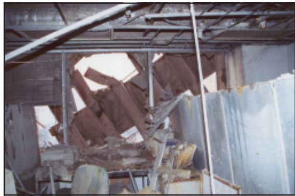
b. View of inside face of WTC 2 façade element
