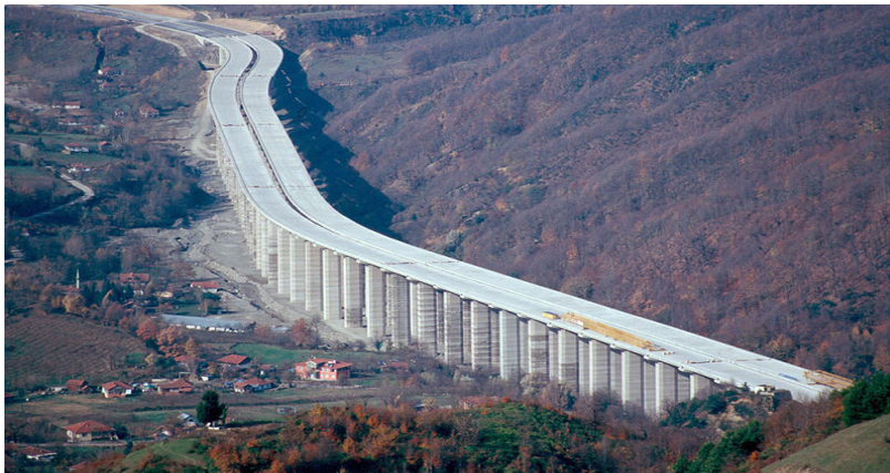
Figure 2-1 General View of Bolu Viaduct 1
