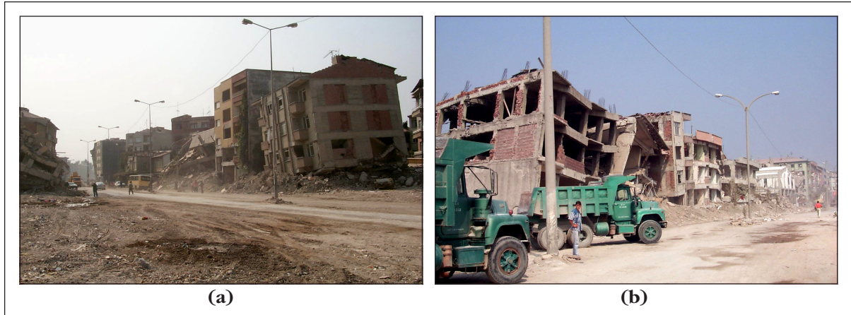
■ Figure 15 . Damage to apartment buildings in the “Circle Area” of Adapazarı. Left image is view (a) in Figure 14b. Right image is view (b) in Figure 14b.
