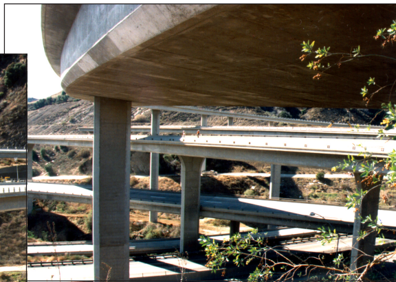
■ Figure 3. Research in spatial variation of ground motion included case studies of the SR14/I-5 interchange and other bridges damaged during the Northridge, California earthquake. Further research is needed to define the importance of these effects and to develop simplified design procedures for a broad range of bridge configurations.
