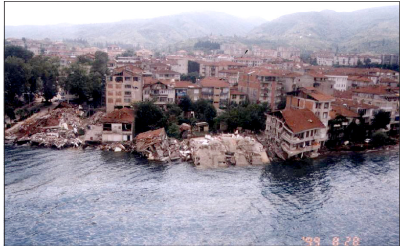
■ Figure 4. Aerial view of earthquake damage in Gölcük. This area was affected by ground subsidence caused by liquefaction.
