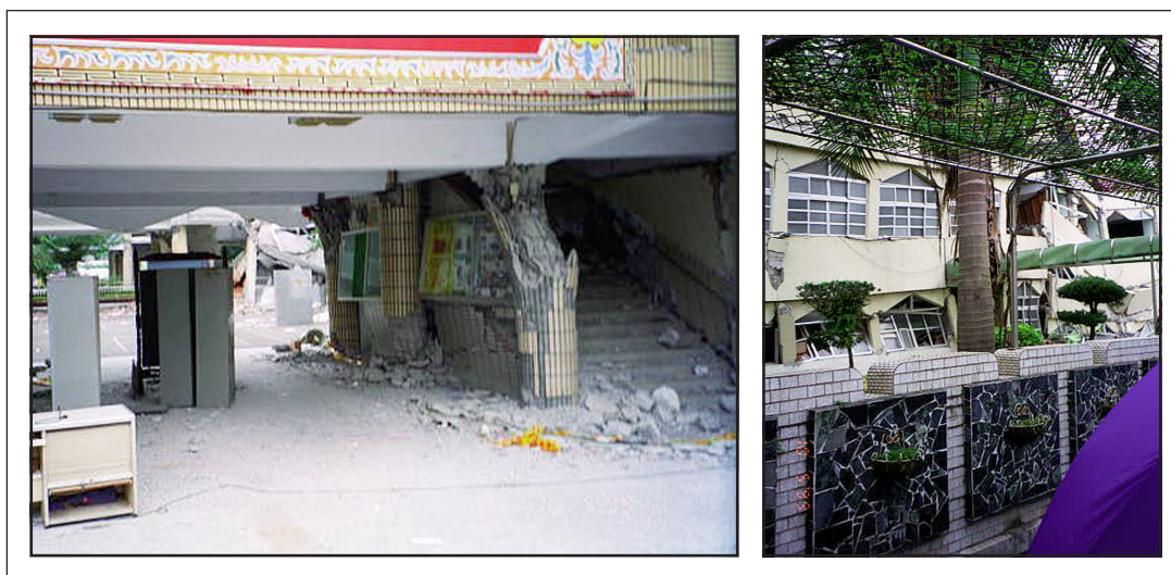
■ Figure 7. Typical damage to schools due to short-column effect and eccentricity
