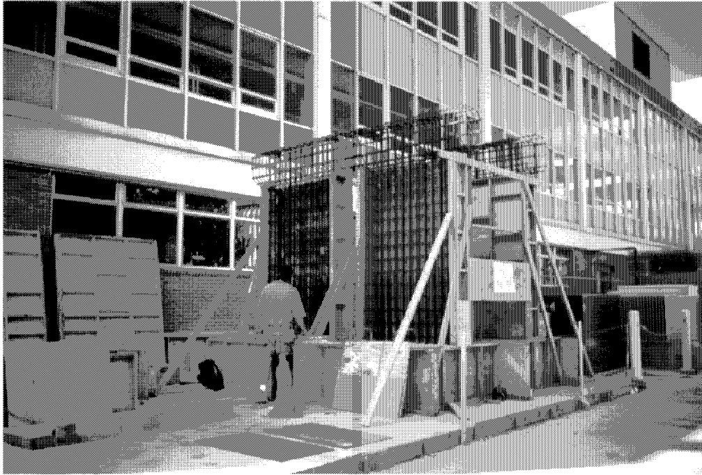
Figure 3-10 Construction of Test Specimens
