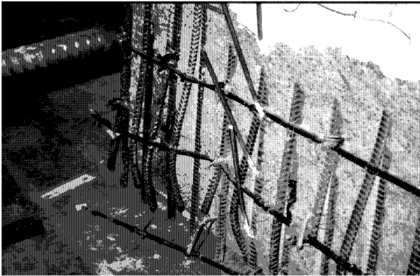
Figure 4-44 Buckling of the Vertical and the Lateral Bars in Specimen 4
